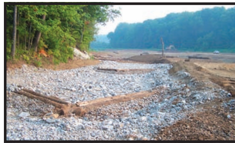
Ongoing Restoration Work North of Broomsage Road
