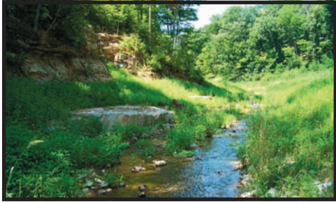
Completed Restoration South Broomsage Road
