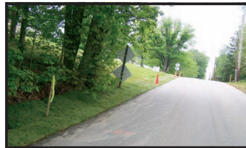
Road Shoulder Repairs
