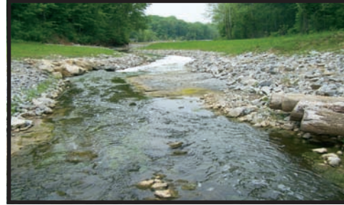
New Restoration Work
