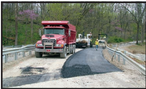
Paving the Broomsage Culvert
