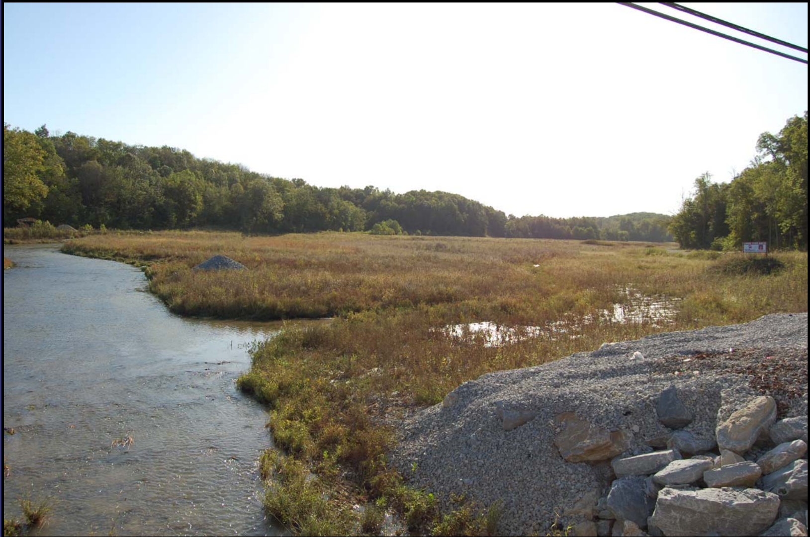
Restoration east of Peerless Road
