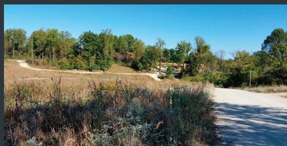
PILOT TRENCH ALIGNMENT LOOKING NORTH
