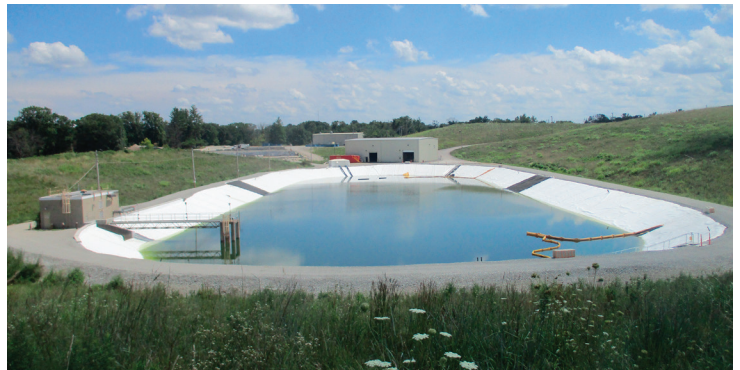
OVERVIEW OF STORMWATER POND
