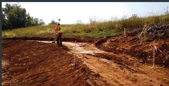
CONSTRUCTION ON AOI 8 REMEDIAL COLLECTION SYSTEM
