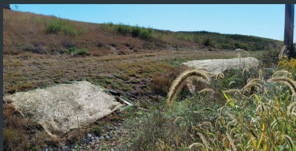
EROSION REPAIRS ON EAST PLANT AREA COVER SYSTEM
