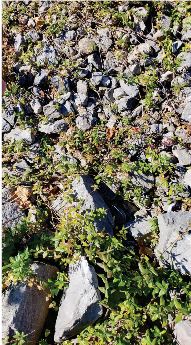
Photo 17: Drainage along EV9 East Plant Area Cover facing southwest
