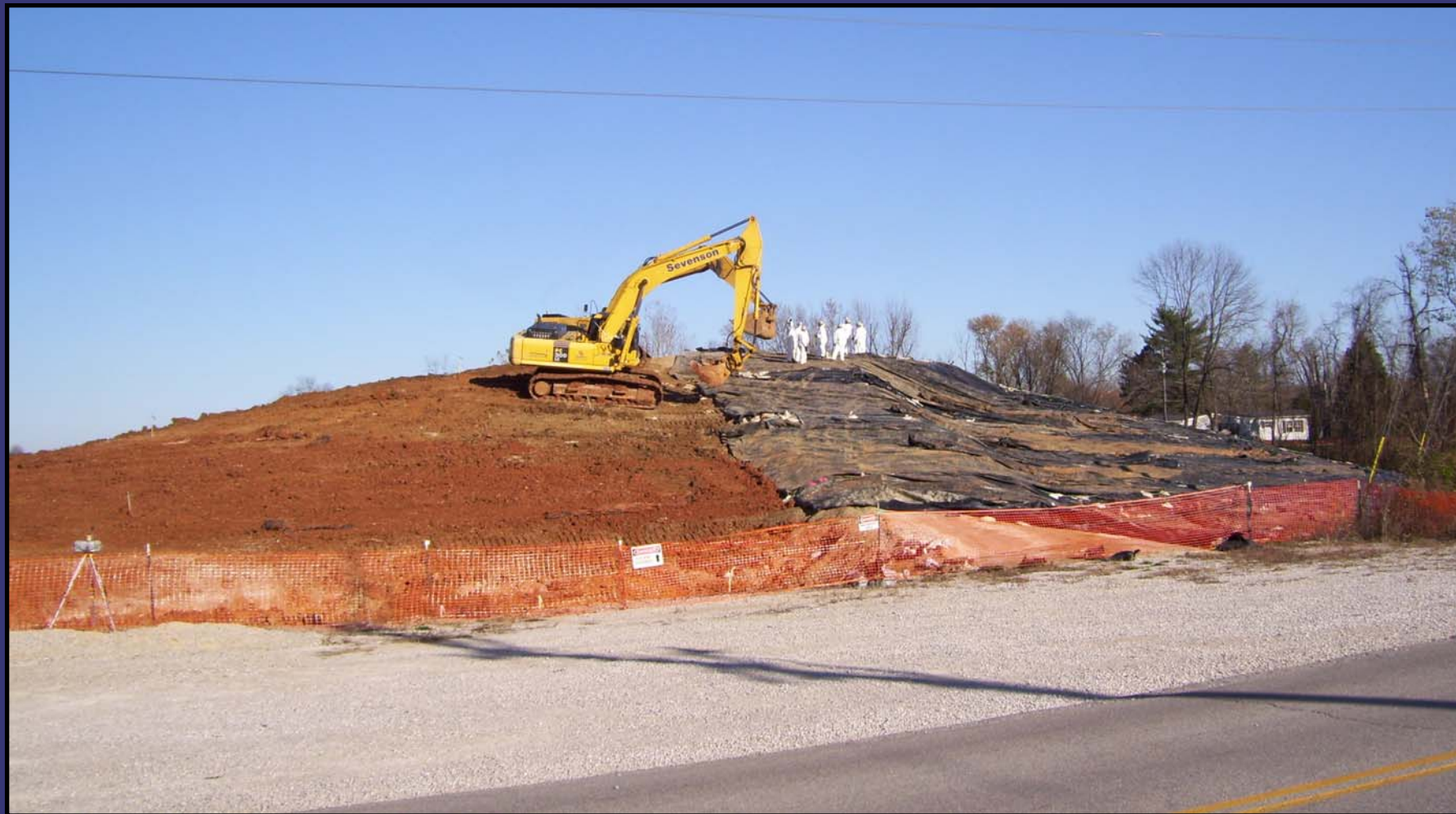
Parcel 201 soil grading off of GM Drive
