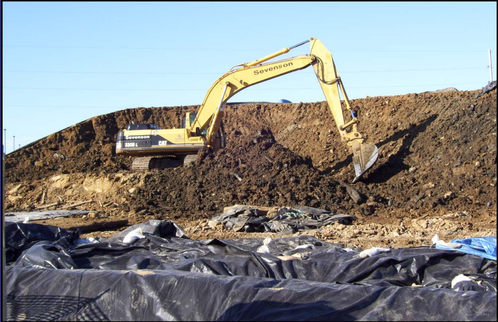
Moving grading fill in the East Plant Area to Parcel 201
