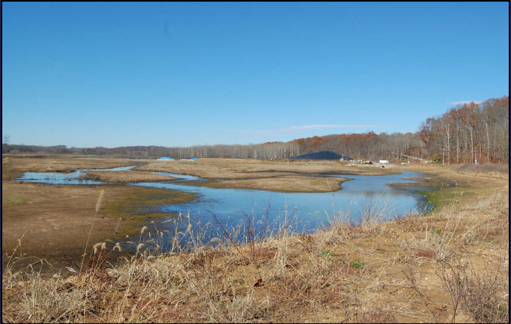
Excavation west of Peerless Road
