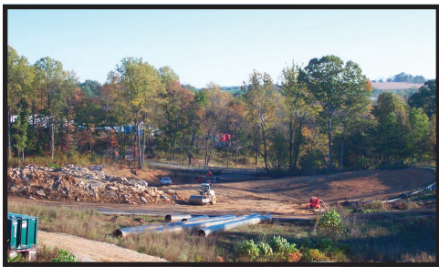
Sediment Pond Construction Near Bailey Scales Road
