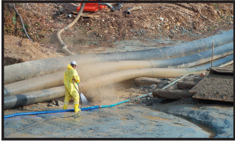
Bedrock Cleaning at Culvert
