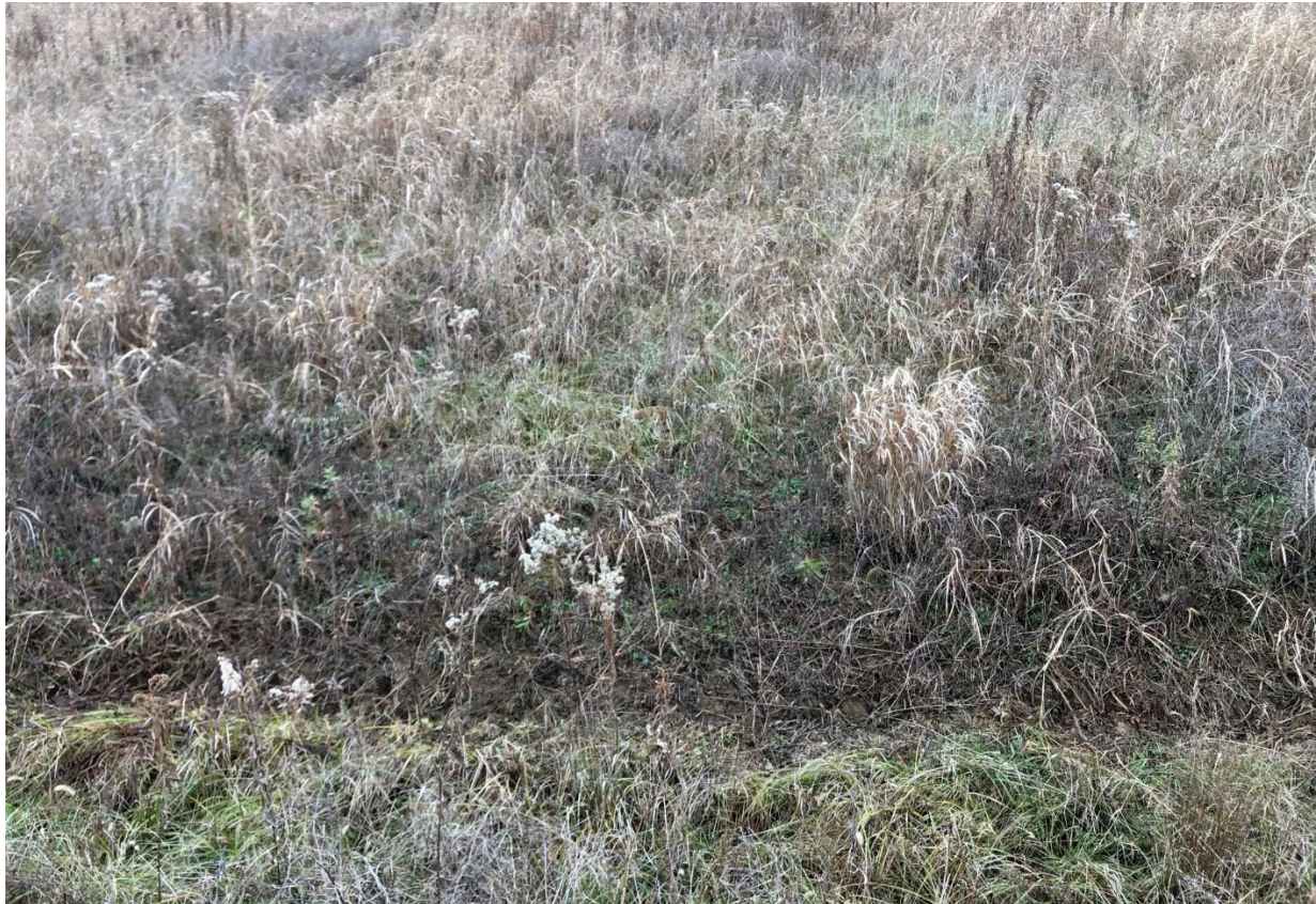
Photo 2: Evidence of erosion near WWTP; facing north
