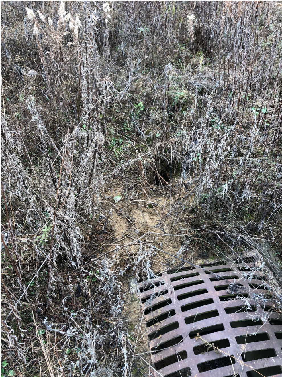
Photo 3: Burrows near ES2 over Vault Cover System; facing southwest
