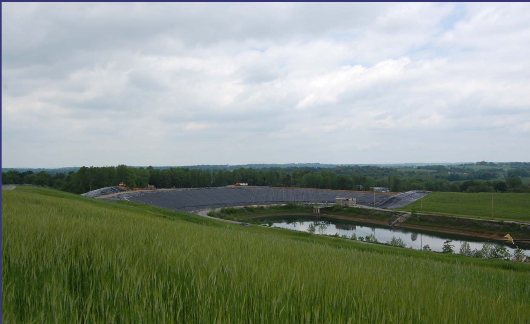
Partially completed cover work around the storm water pond.
