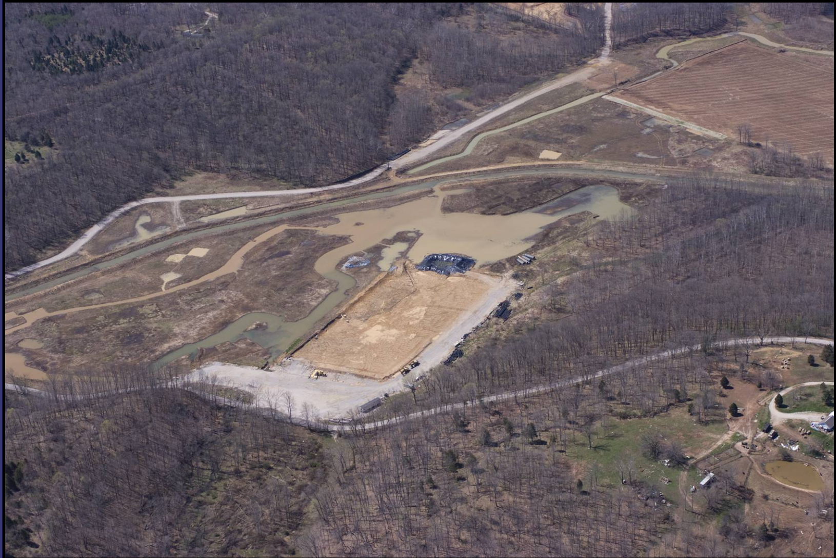
Excavation remaining west of Peerless Road
