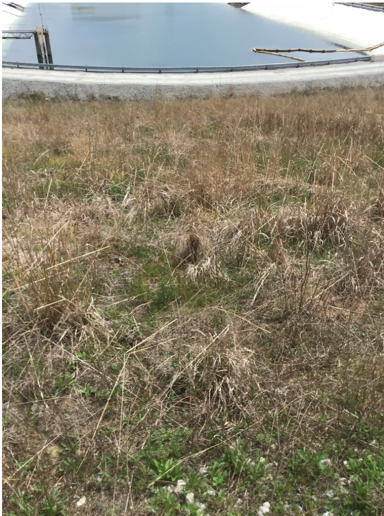
Photo 3: EV3 East Plant Cover facing south towards stormwater pond
