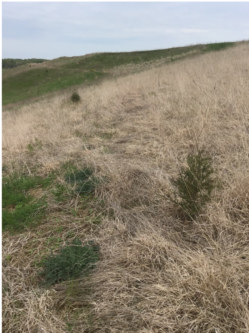
Photo 6: EV2 East Plant Cover area facing southeast
