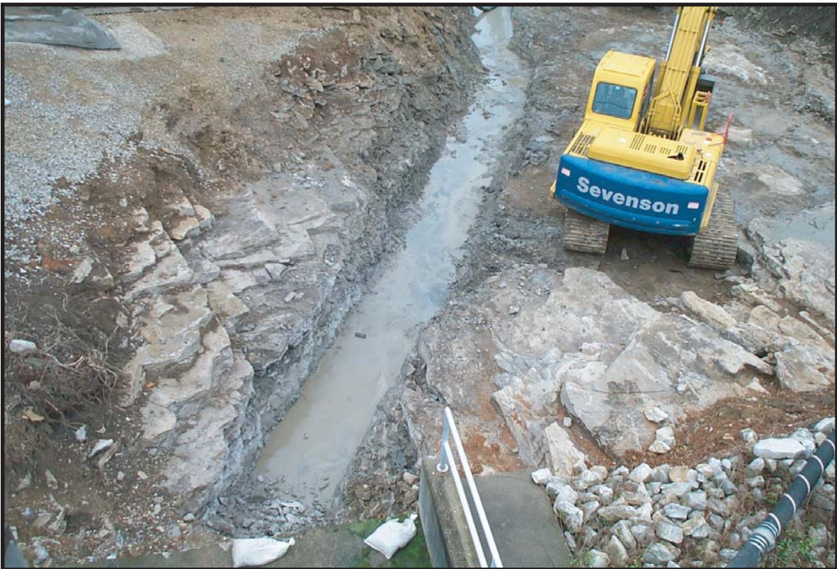
Photo 6- Rock removal immediately downstream of Outfall 002, looking toward Trench 1
