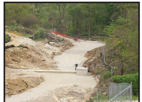
Site Source Control system during installation
