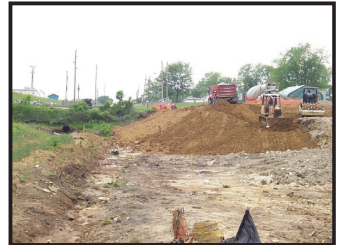
Back filling activities north of GMs property
