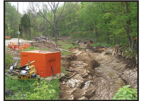
View looking east of Bailey Scales Road - during excavation activities
