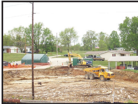
Soil removal to bedrock north of GMs property
