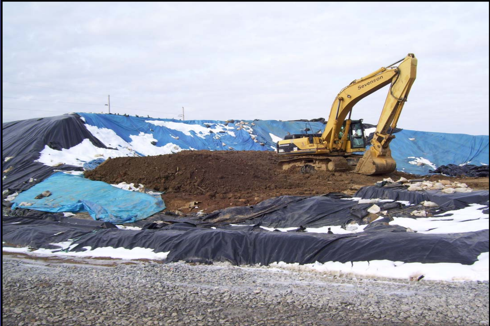
Moving grading fill in the East Plant Area at AOI 15
