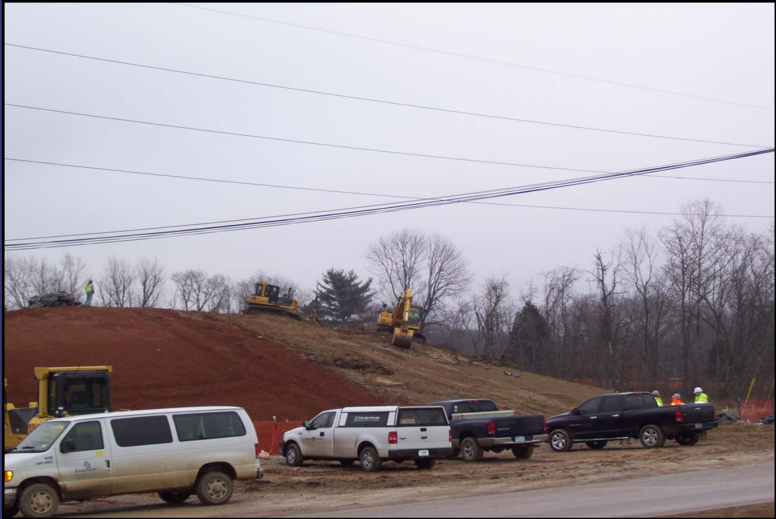
Parcel 201 soil grading off of GM Drive
