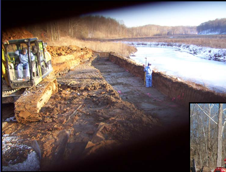
Excavation status in January
