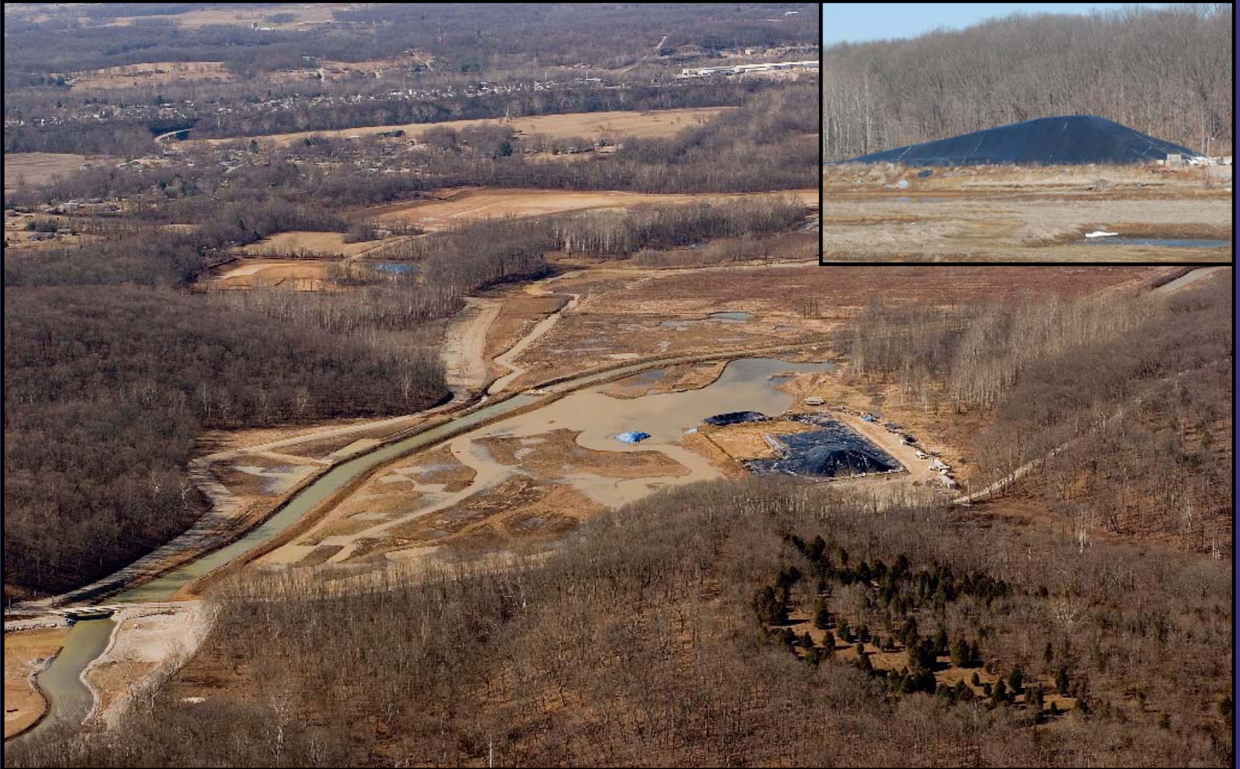
Excavation and soil pile remaining west of Peerless Road
