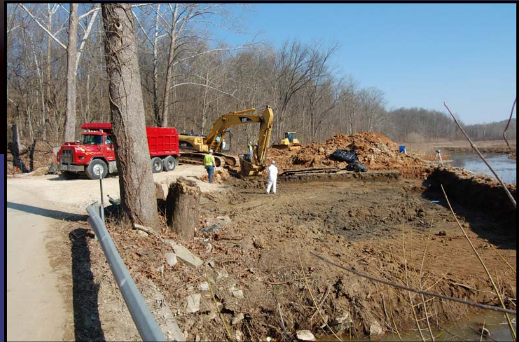
Excavation status in March
