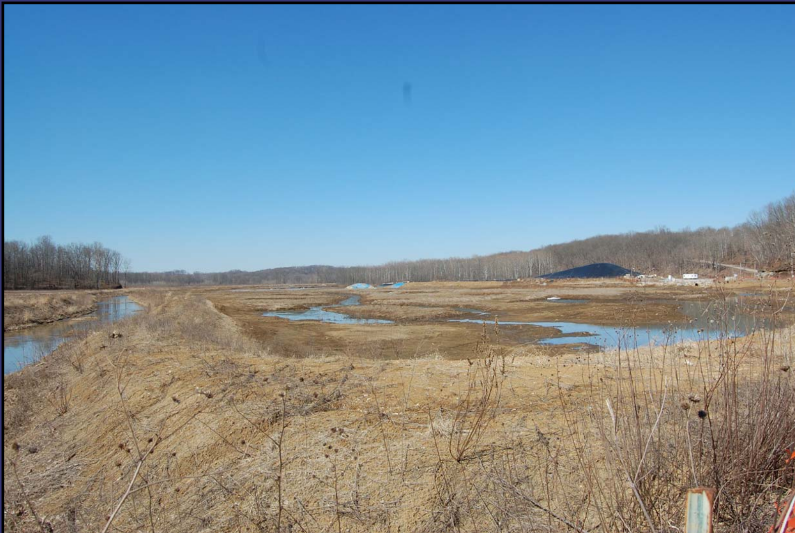
Excavation west of Peerless Road
