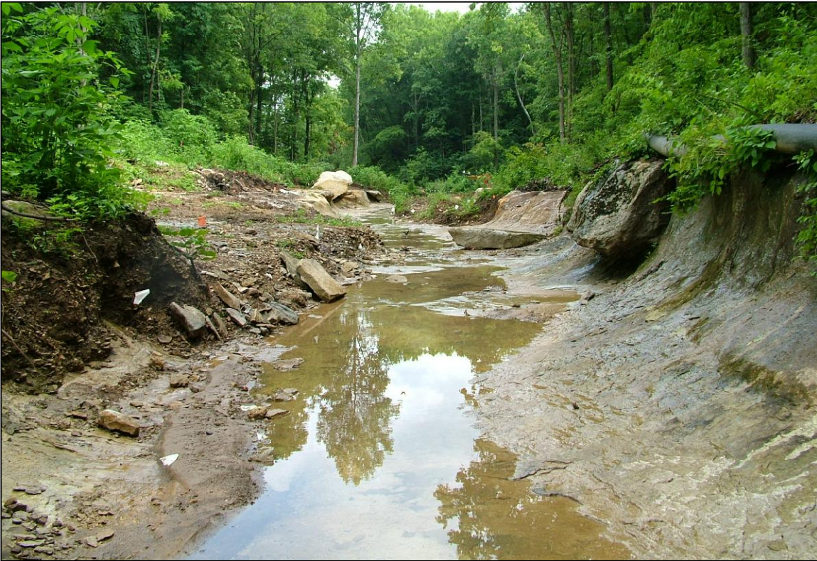
PHOTO No.42, PARCELS 8 & 10: LOOKING DOWNSTREAM ALONG CHANNEL EXCAVATION (JUL. 2004)
