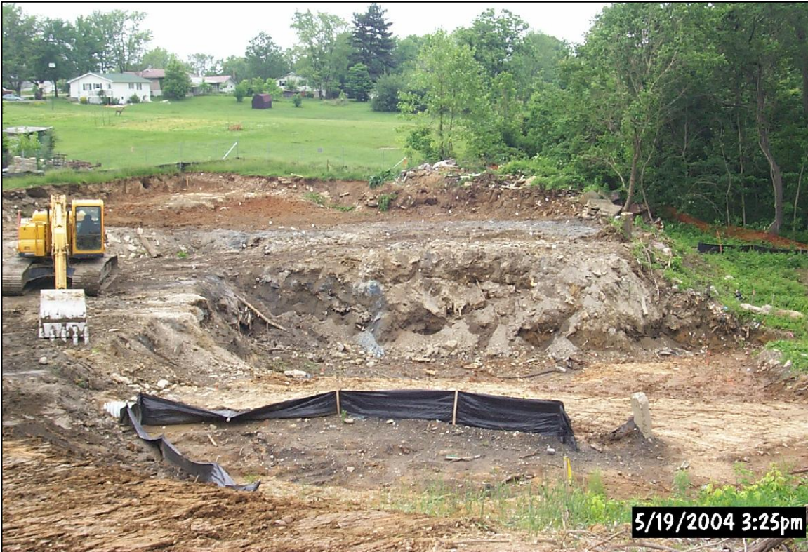
PHOTO No.72, PARCEL 401: EXCAVATION OF PARCEL 401 FILL AREA (MAY 2004)
