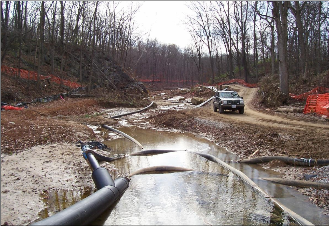
PHOTO No.55, PARCELS 11 & 12: LOOKING DOWNSTREAM ALONG CREEK EXCAVATION (NOV. 2004)
