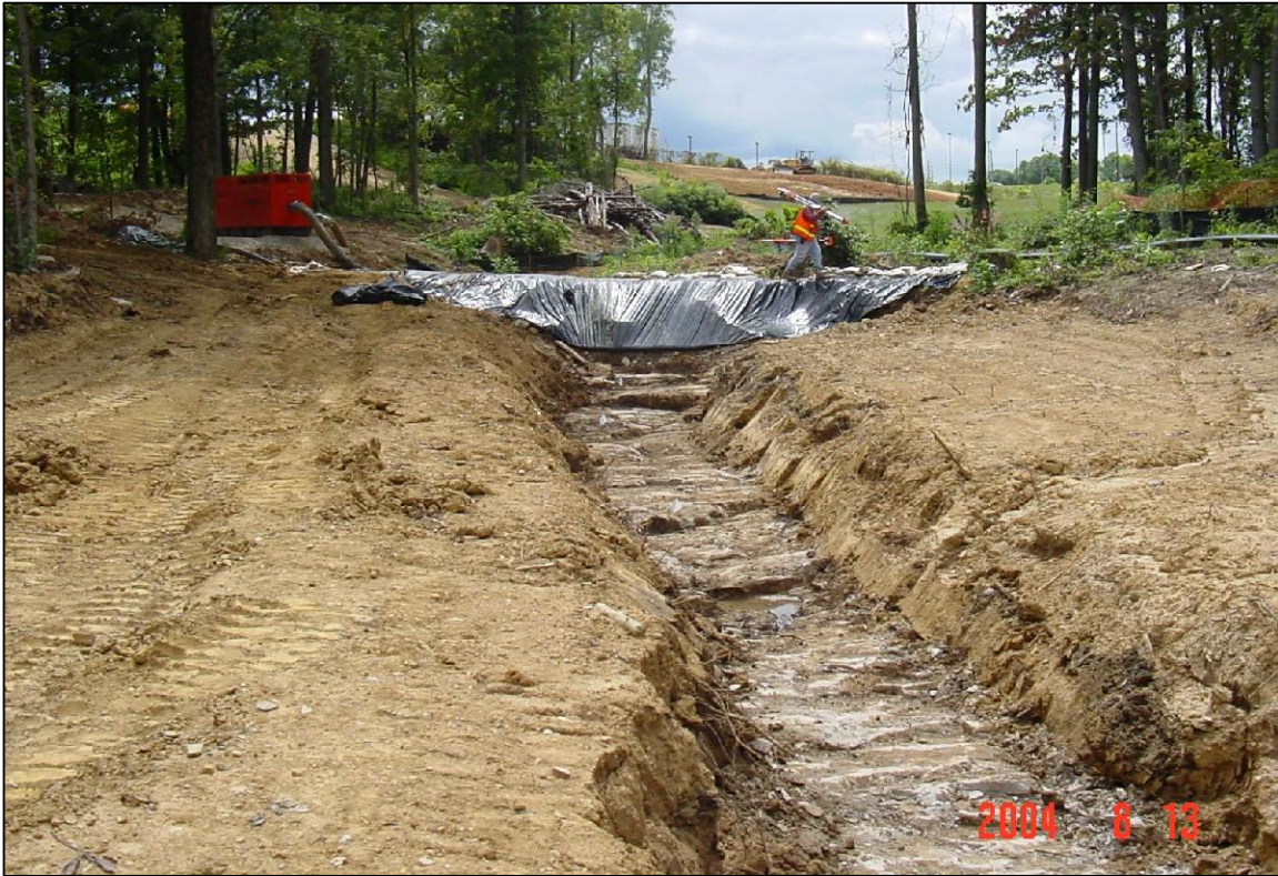
PHOTO No.81, N AOI 4: EXCAVATION LOOKING WEST AT DAM (AUG. 2004)
