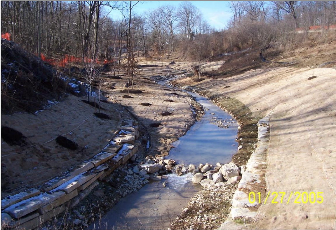
PHOTO No.29, PARCEL 5: COMPLETED RESTORATION INSTALLATION (JAN. 2005)
