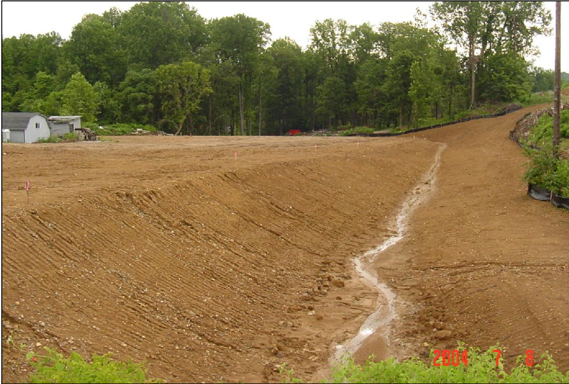
PHOTO No.73, PARCEL 401: BACKFILLED CREEK ALIGNMENT ALONG PARCEL 401 AND AOI 4 (JUL. 2004)
