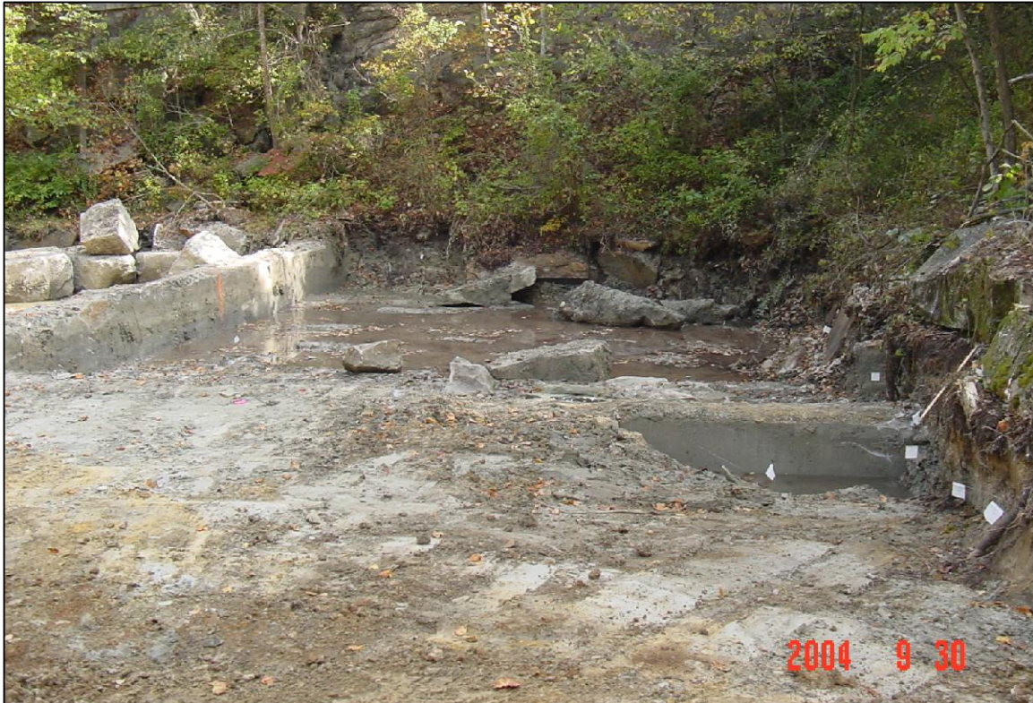
PHOTO No.64, QUARRY: ONGOING EXCAVATION IN THE LOWER QUARRY (SEP. 2004)
