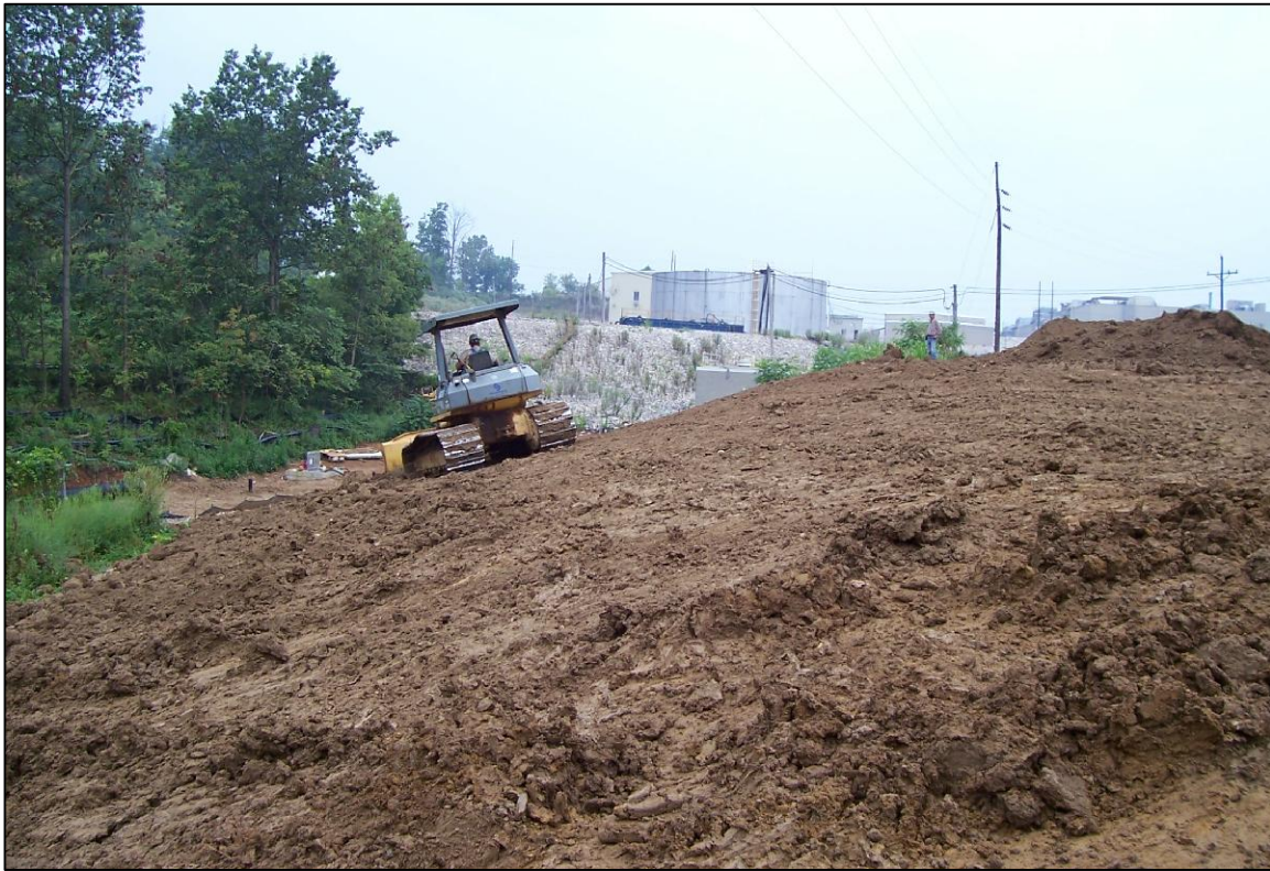
PHOTO No.11, PARCEL 205: GRADING BACKFILL IN PARCELS 3 AND 205 RESTORATION (AUG. 2004)
