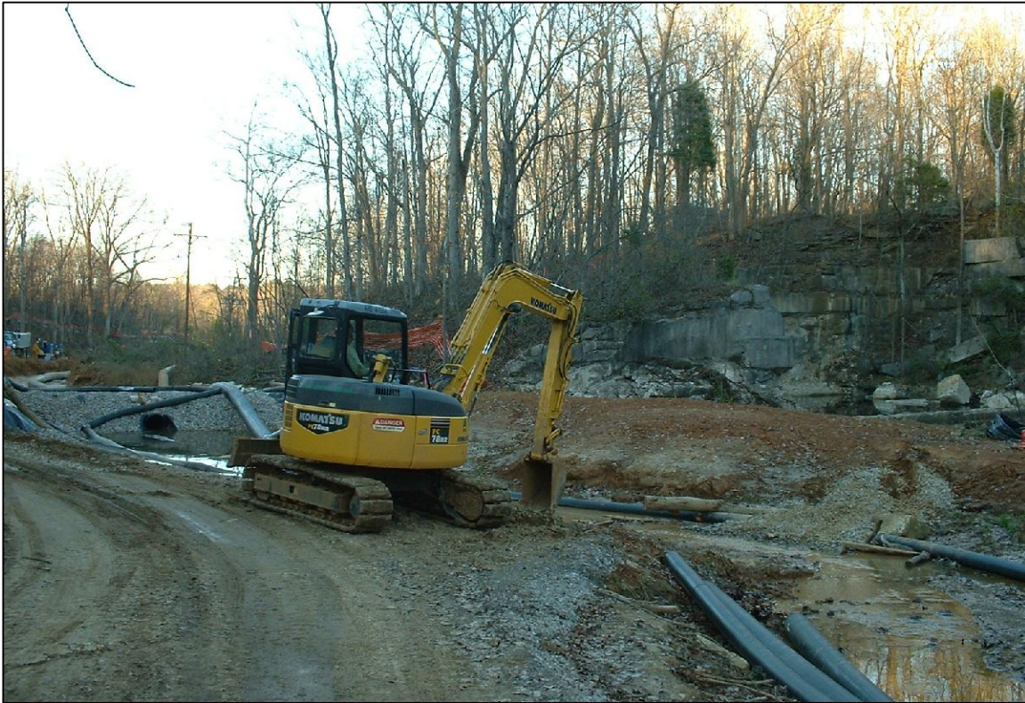
PHOTO No.54, PARCELS 11 & 12: ONGOING RESTORATION OF QUARRY PARCEL 11 REGION (NOV. 2004)
