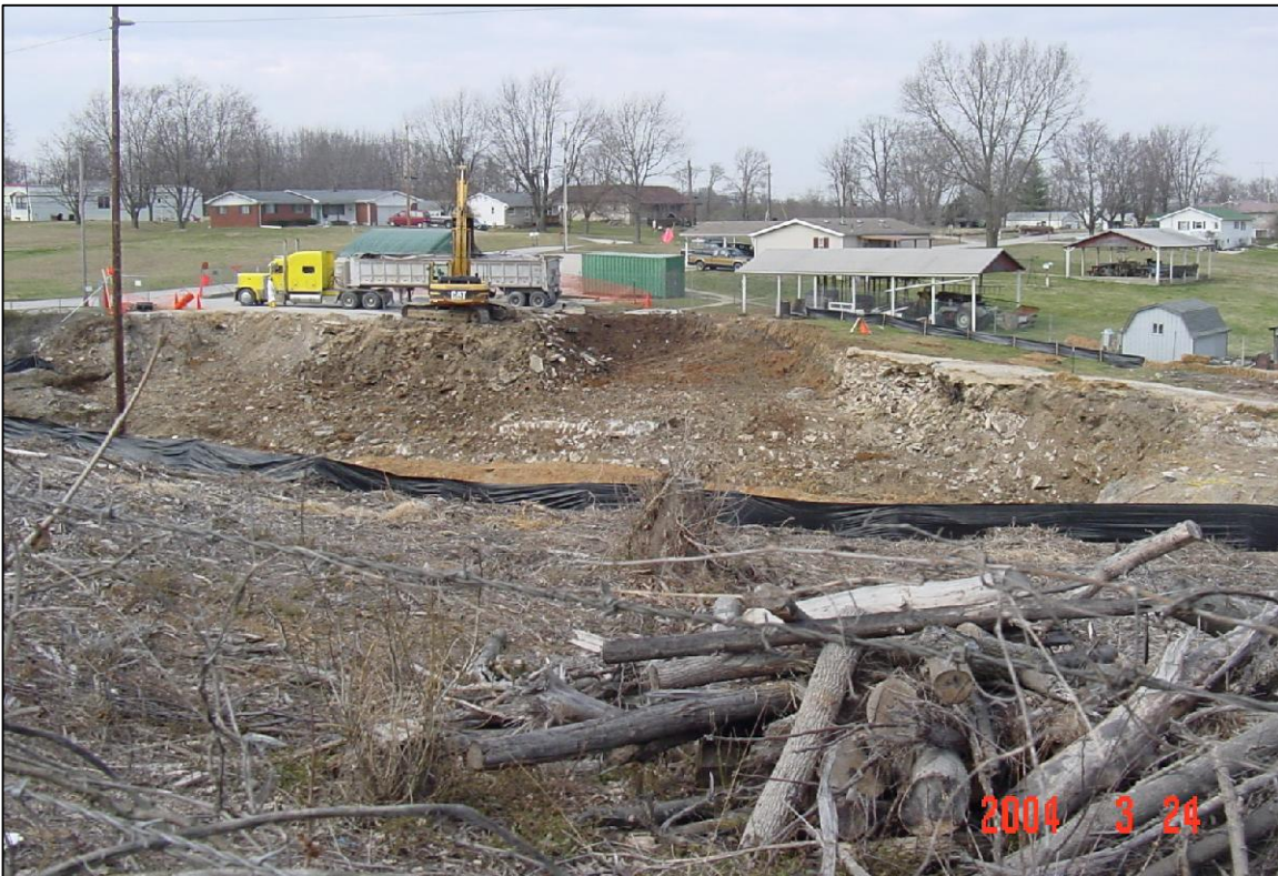
PHOTO No.70, PARCEL 401: EXCAVATION OF FILL AREA (MAR. 2004)
