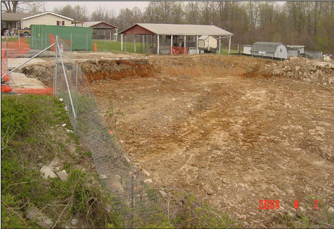
PHOTO No.71, PARCEL 401: EXCAVATION OF FILL AREA (APR. 2004)
