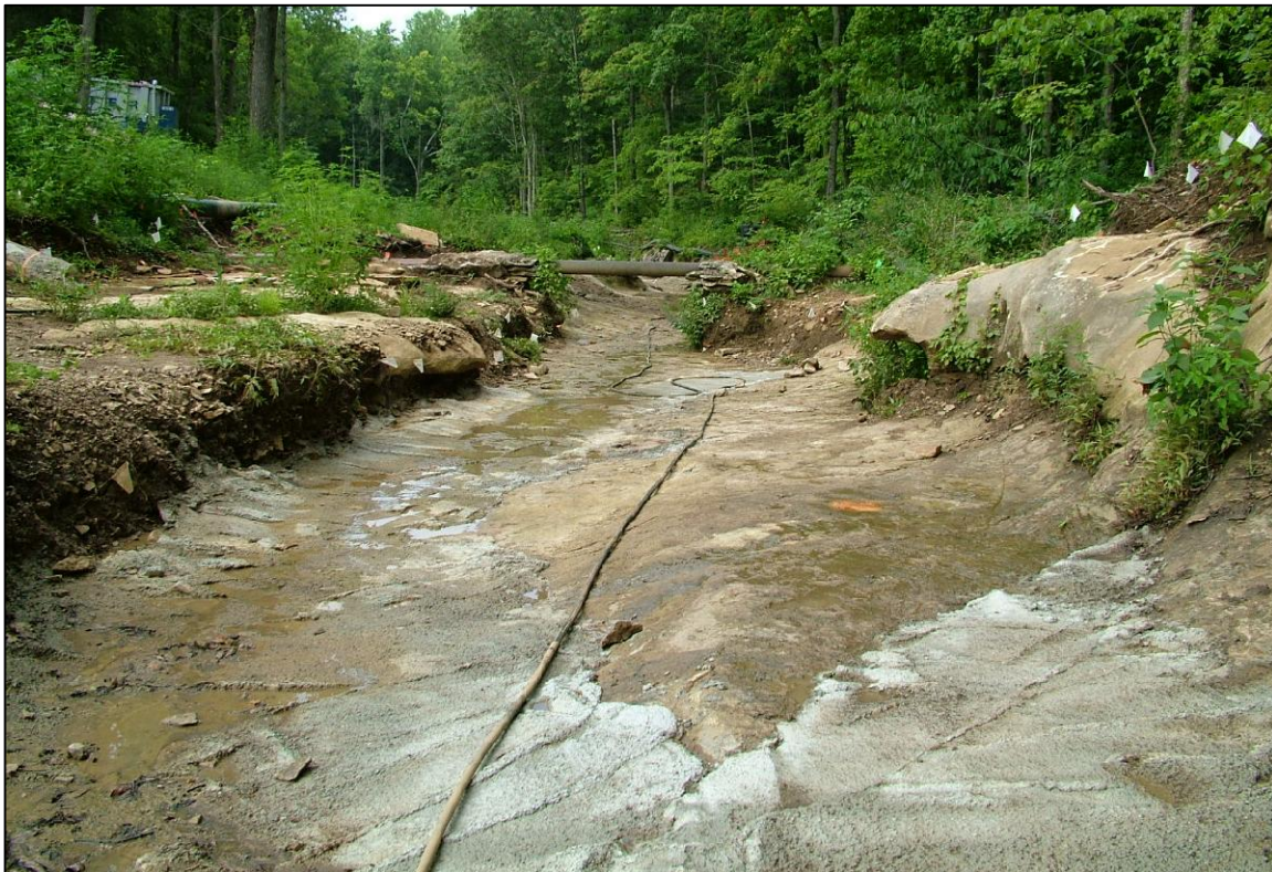
PHOTO No.37, PARCELS 7 & 8: EXCAVATED CREEK CHANNEL FACING DOWNSTREAM (NORTHEAST) (JUL. 2004)
