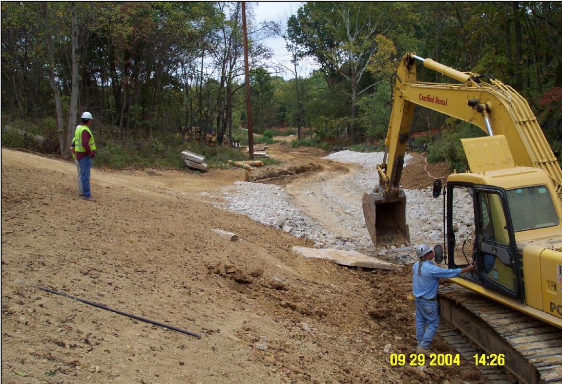
PHOTO No.17, PARCEL 4: BACKFILL AND ROUGHBACK PLACEMENT ALONG CREEK ALIGNMENT (SEP. 2004)
