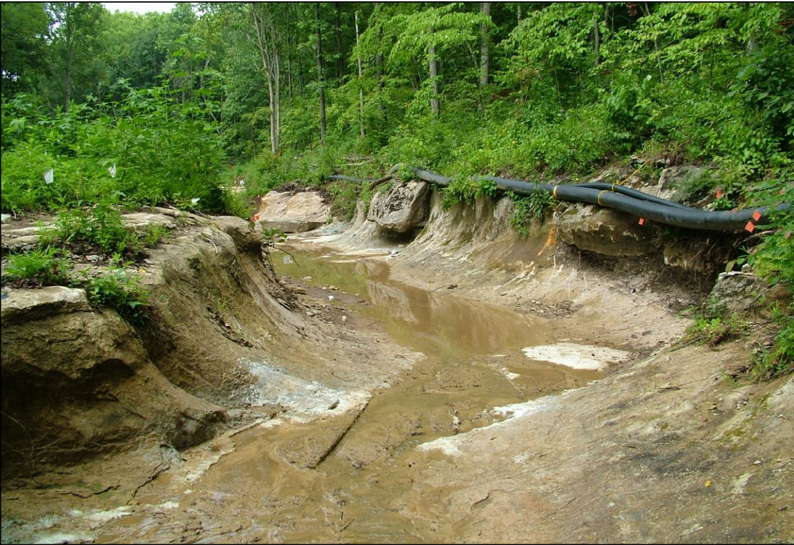
PHOTO No.43, PARCELS 8 & 10: LOOKING DOWNSTREAM ALONG CHANNEL EXCAVATION (JUL. 2004)
