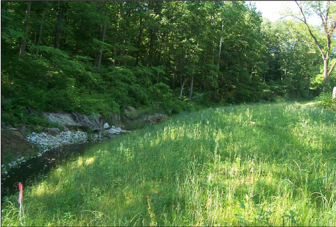
PHOTO No.48, PARCELS 8 & 10: RESTORED CREEK ON PARCELS 8 AND 10 (JUN. 2005)
