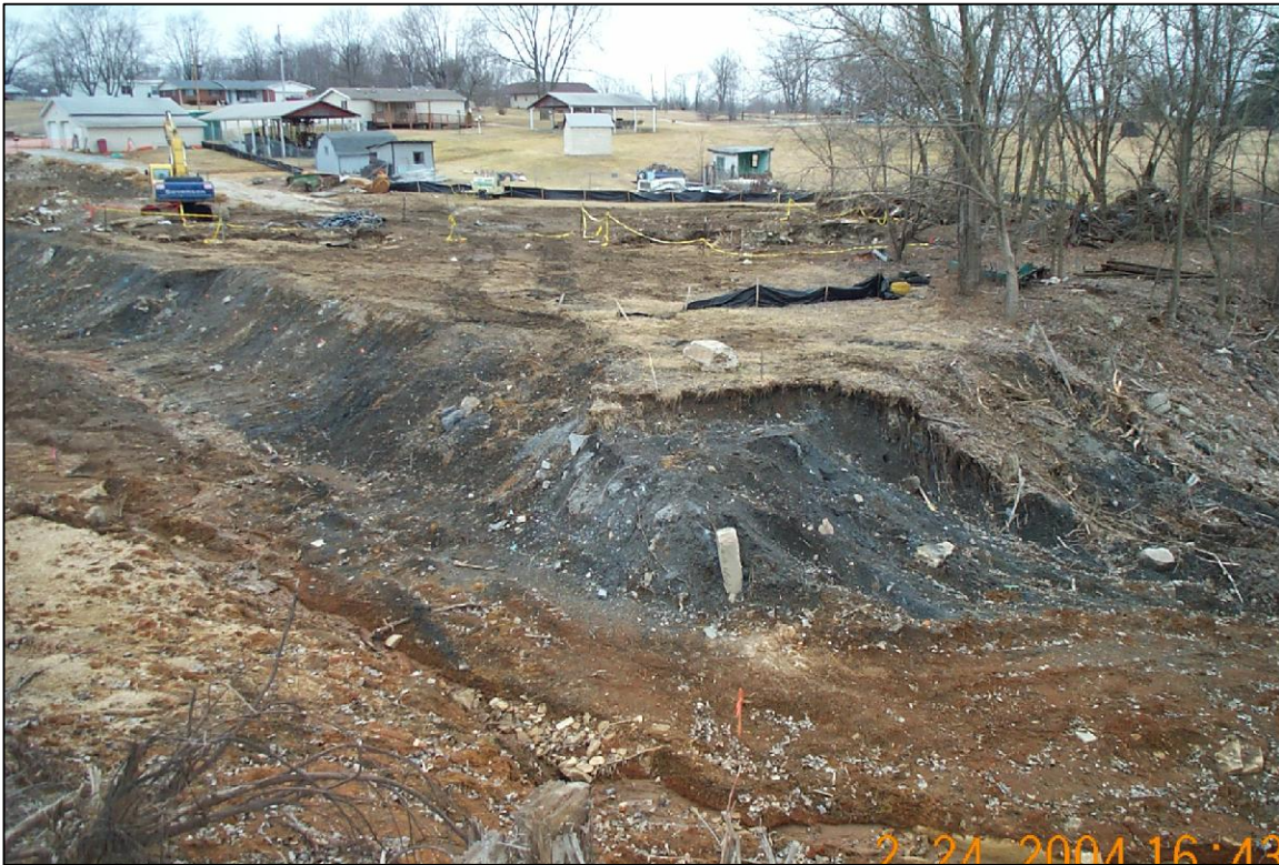
PHOTO No.69, PARCEL 401: EXCAVATION OF PARCEL 401 FILL AREA (FEB. 2004)
