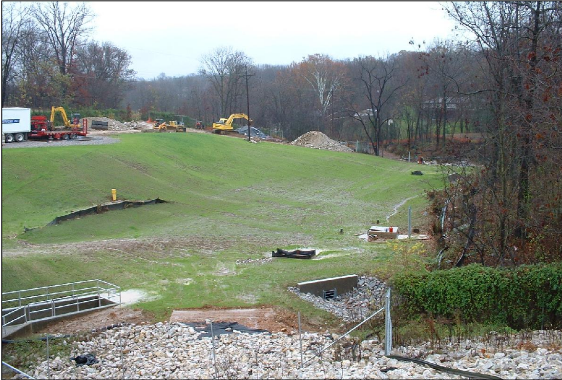
PHOTO No.7, PARCEL 3: RESTORED PARCEL 3 AND 205, FACING DOWNSTREAM (EAST) (NOV. 2004)
