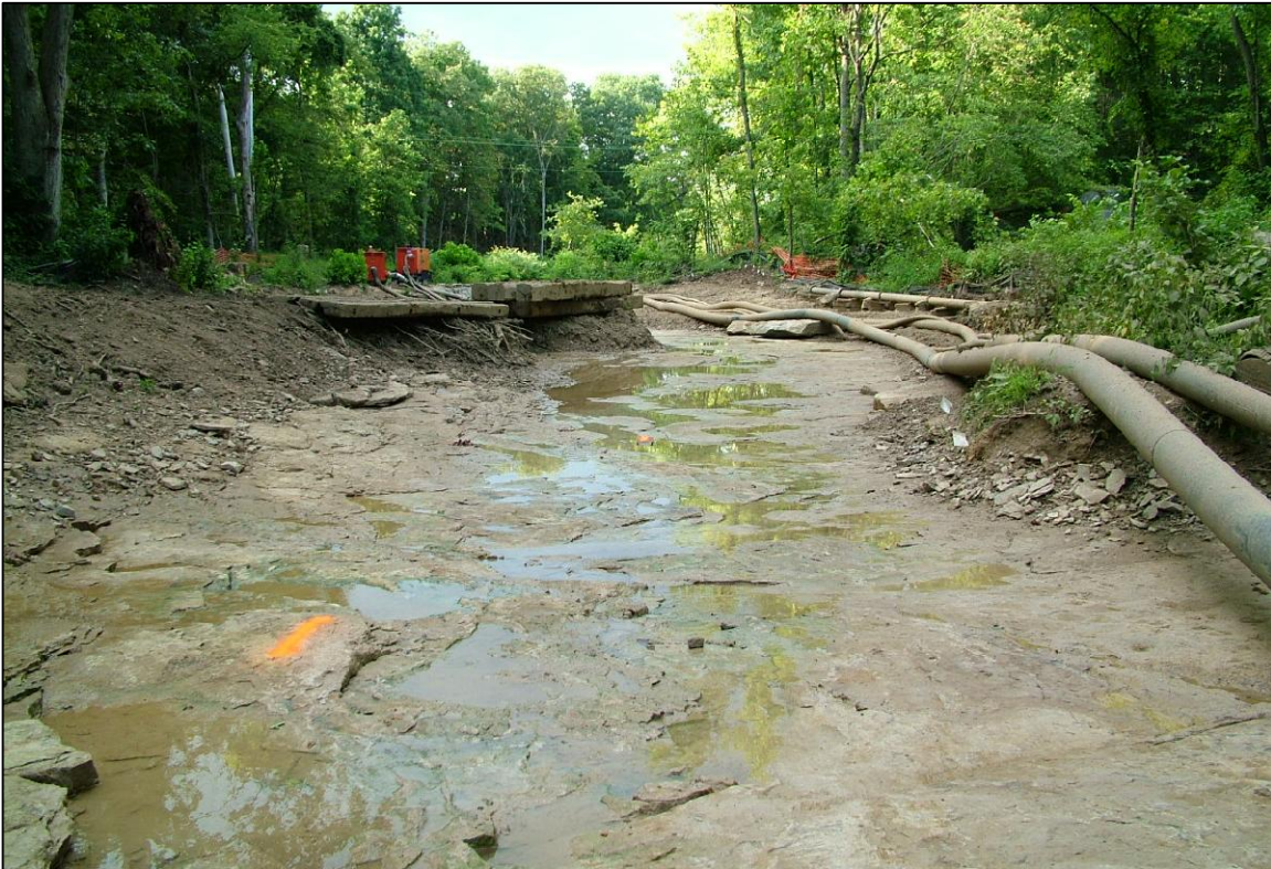
PHOTO No.53, PARCELS 11 & 12: WASHED CREEKBED FACING DOWNSTREAM (AUG. 2004)
