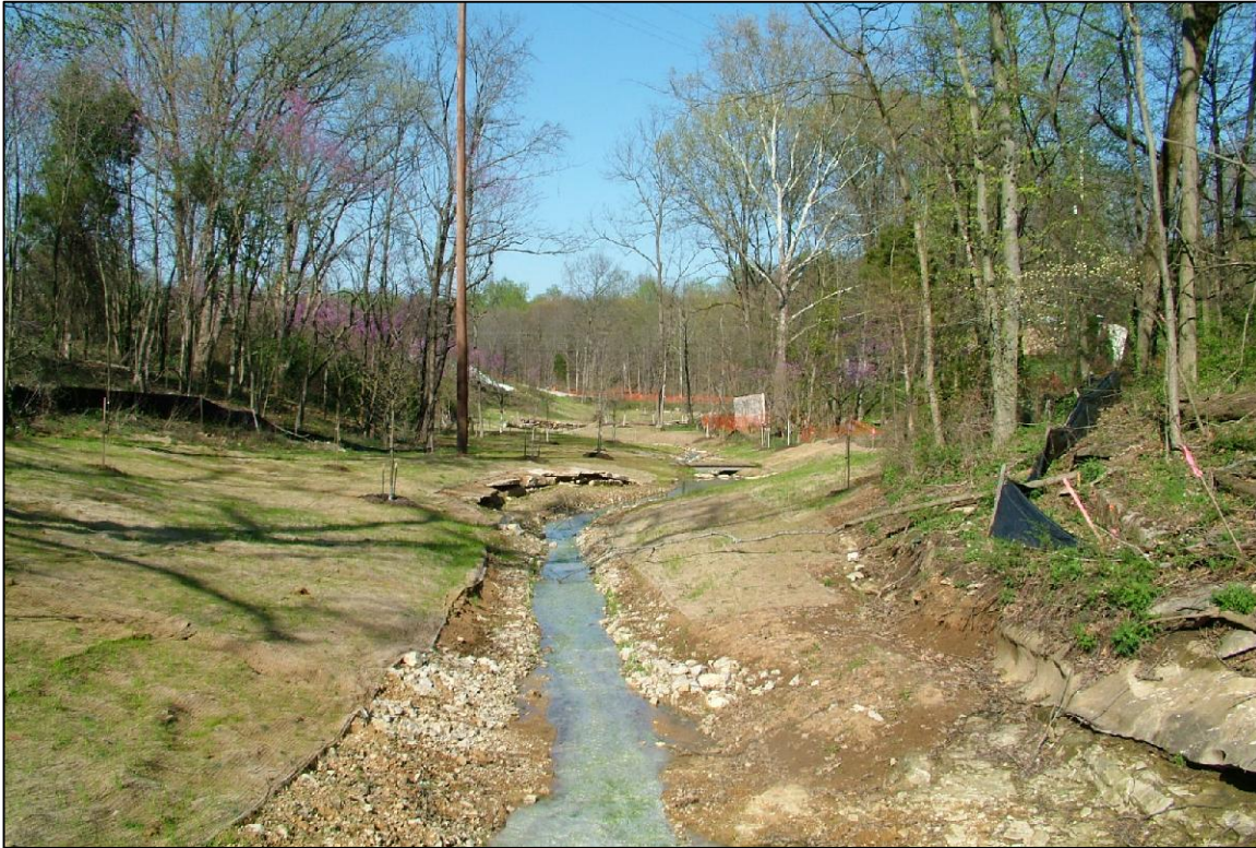
PHOTO No.18, PARCEL 4: RESTORED CREEK ALIGNMENT (APR. 2005)
