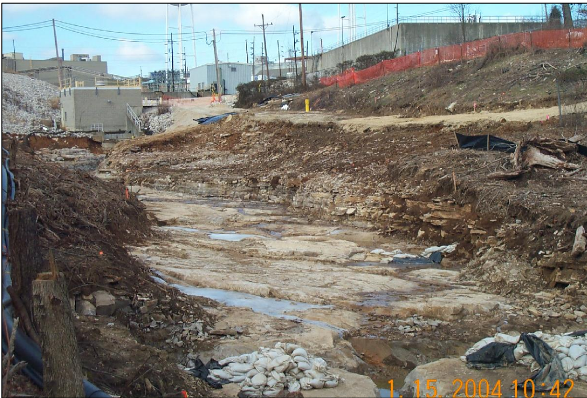
PHOTO No.5, PARCEL 3: UPSTREAM (WEST) ALONG EXCAVATED CREEK ALIGNMENT (JAN. 2004)
