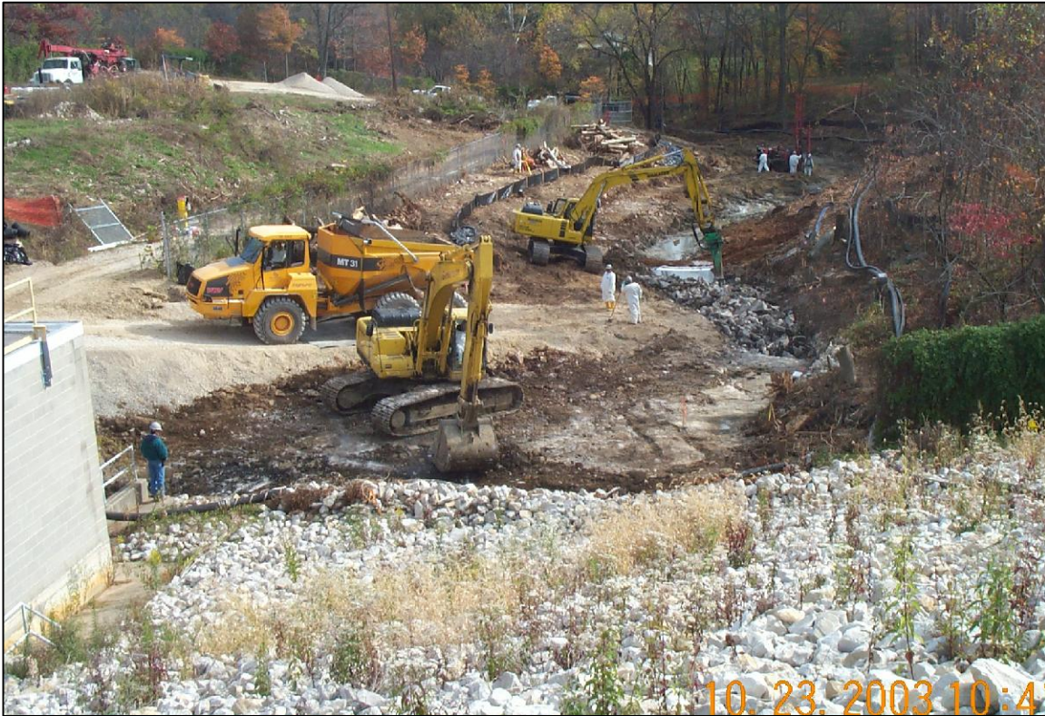
PHOTO No.3, PARCEL 3: EXCAVATION AND ROCK BREAKING, FACING DOWNSTREAM (EAST) (OCT. 2003)
