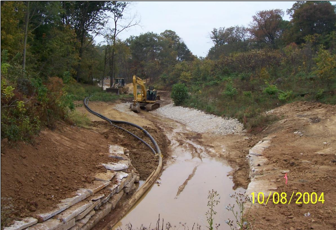
PHOTO No.27, PARCEL 5: GRADING BACKFILL IN PARCEL 5 AND 6 RESTORATION (OCT. 2004)
