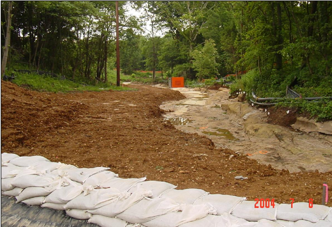
PHOTO No.16, PARCEL 4: BACKFILL PROGRESS ON PARCEL 4 (JUL. 2004)
