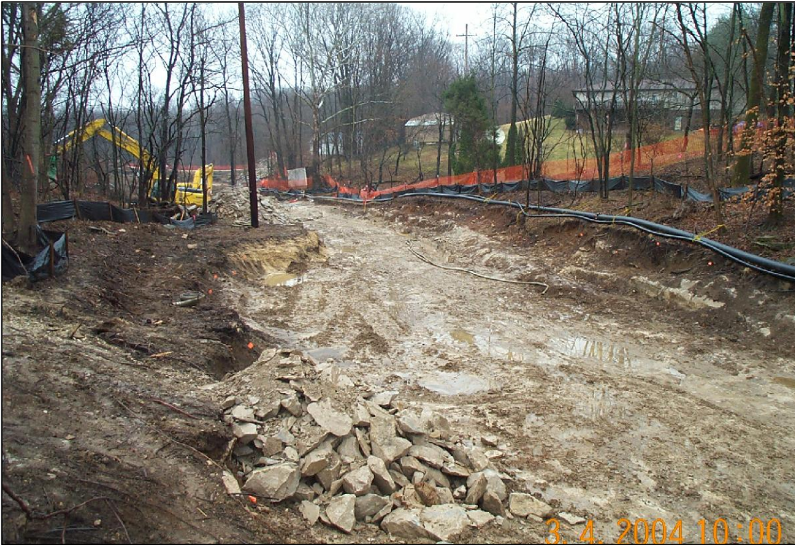
PHOTO No.15, PARCEL 4: EXCAVATION WORK ON PARCEL 4 PROGRESSING DOWNSTREAM (NORTHEAST) (MAR. 2004)
