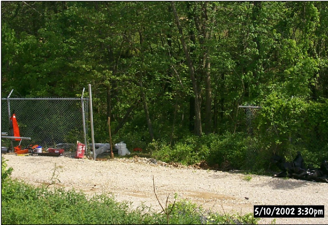
PHOTO No.9, PARCEL 205: MOBILIZATION AT OUTFALL 002 ON PARCEL 205 (MAY 2002)
