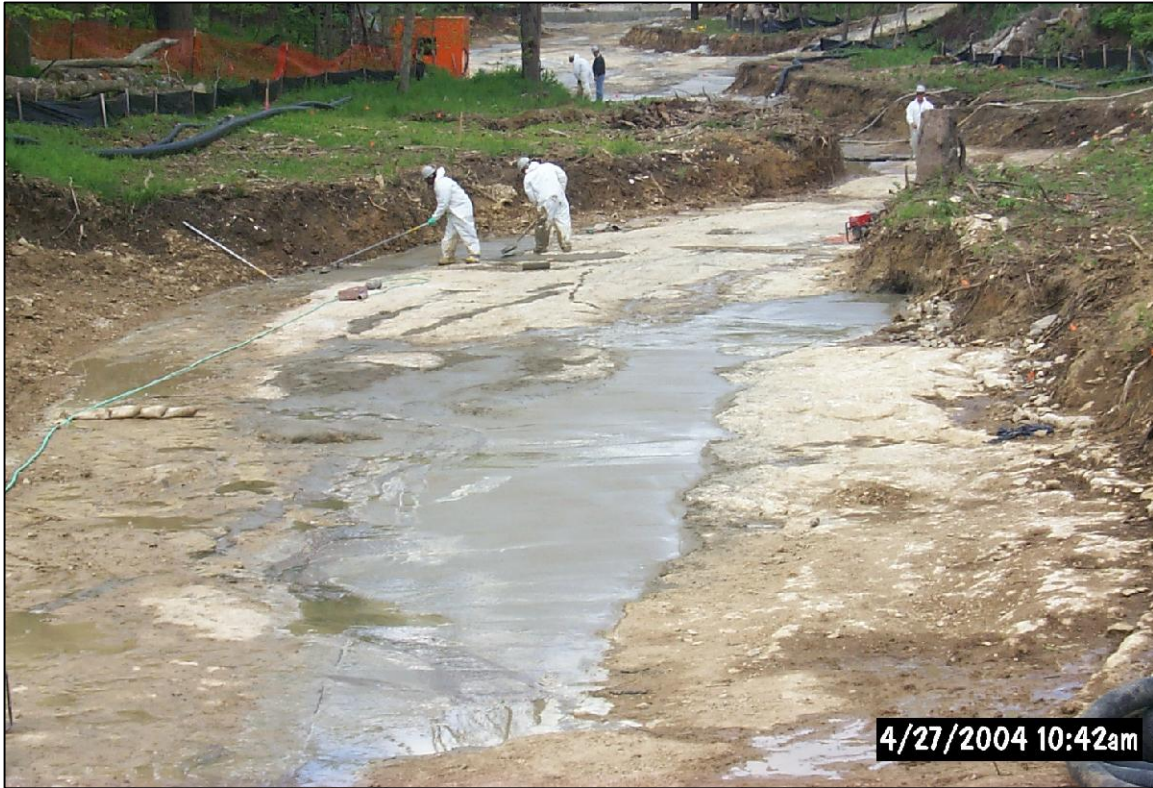
PHOTO No.25, PARCEL 5: CRACK FILLING ALONG PARCEL 5 AND 6 CREEK ALIGNMENT (APR. 2004)
