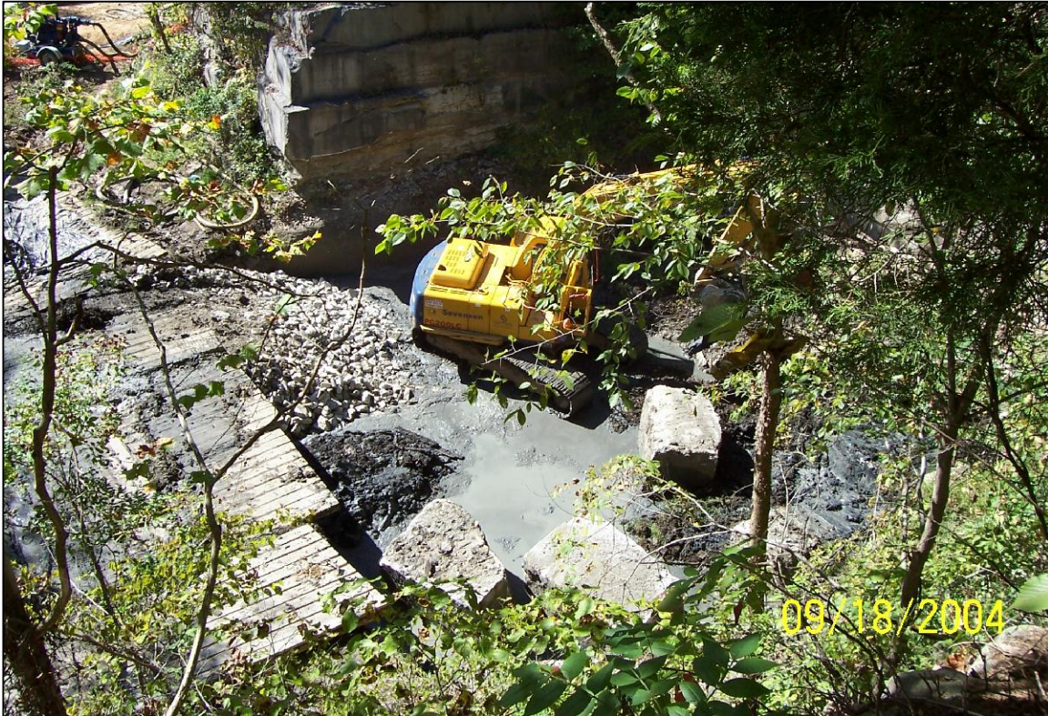
PHOTO No.62, QUARRY: LOOKING DOWN INTO QUARRY DURING CONSTRUCTION ACTIVITIES (SEP. 2004)
