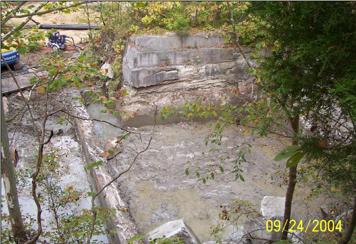
PHOTO No.63, QUARRY: CLEANED QUARRY EXCAVATION (SEP. 2004)
