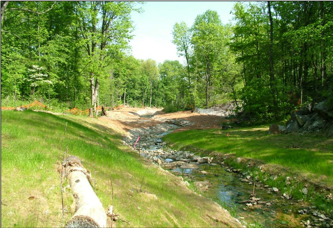
PHOTO No.57, PARCELS 11 & 12: RESTORED PARCELS; LOG FEATURE IN FOREGROUND, RIFFLE FEATURE IN CREEK (MAY 2005)
