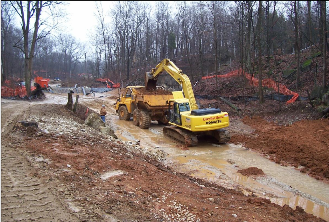
PHOTO No.56, PARCELS 11 & 12: RESTORATION BACKFILLING (JAN. 2005)
