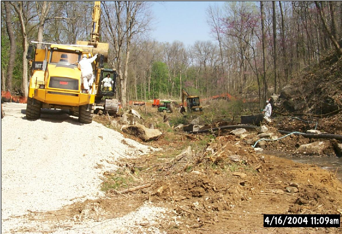
PHOTO No.52, PARCELS 11 & 12: LOOKING UPSTREAM. CONSTRUCTION MOBILIZATION ONGOING (APR. 2004)
