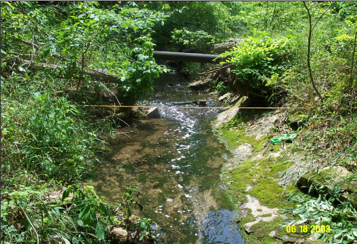
PHOTO No.36, PARCELS 7 & 8: FACING DOWNSTREAM (NORTHEAST) TOWARDS PIPE CROSSING CREEK AT PARCEL 7 AND 8
