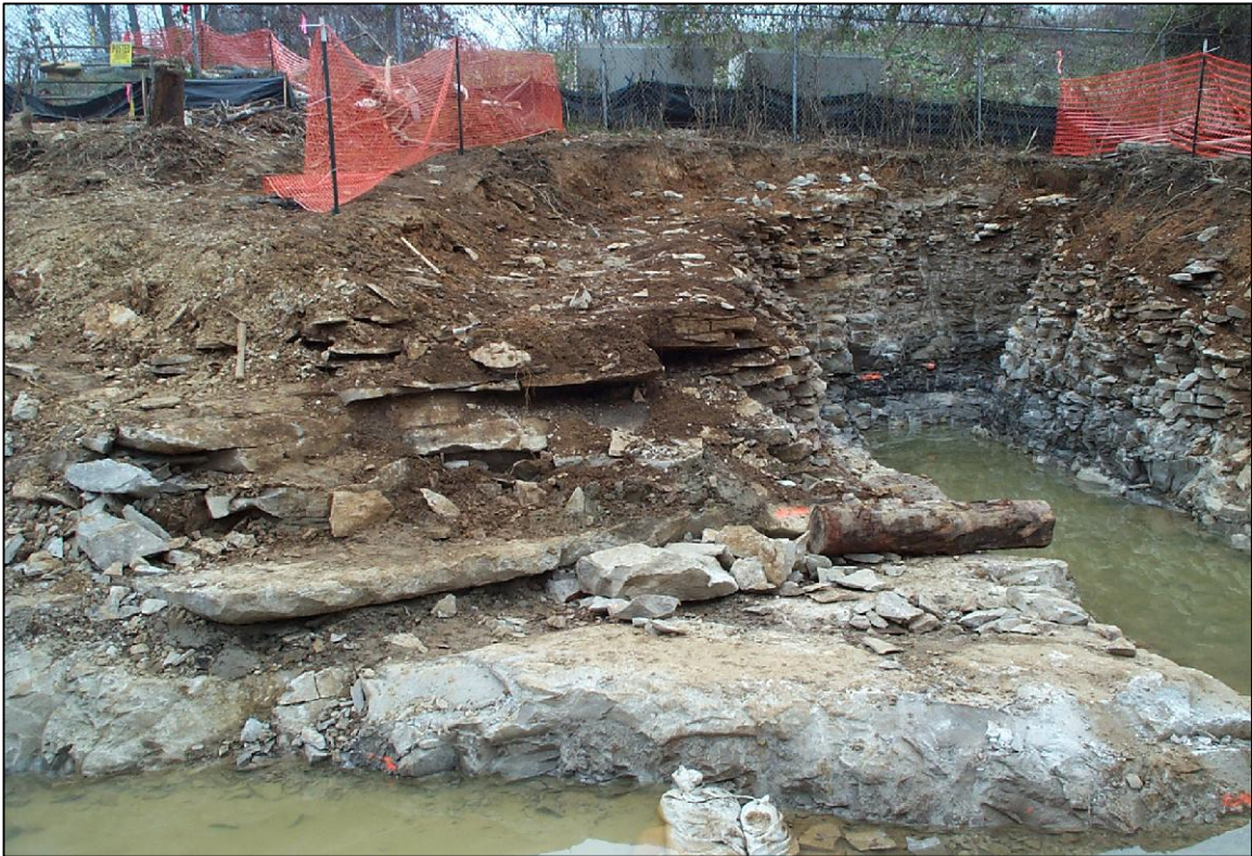
PHOTO No.10, PARCEL 205: TRENCH 1 EXCAVATION ALONG PARCEL 205 SIDEWALL (NOV. 2003)
