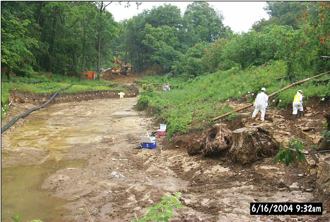
PHOTO No.26, PARCEL 5: VERIFICATION SOIL SAMPLING PARCEL 5 AND 6 EXCAVATION LIMITS (JUN. 2004)
