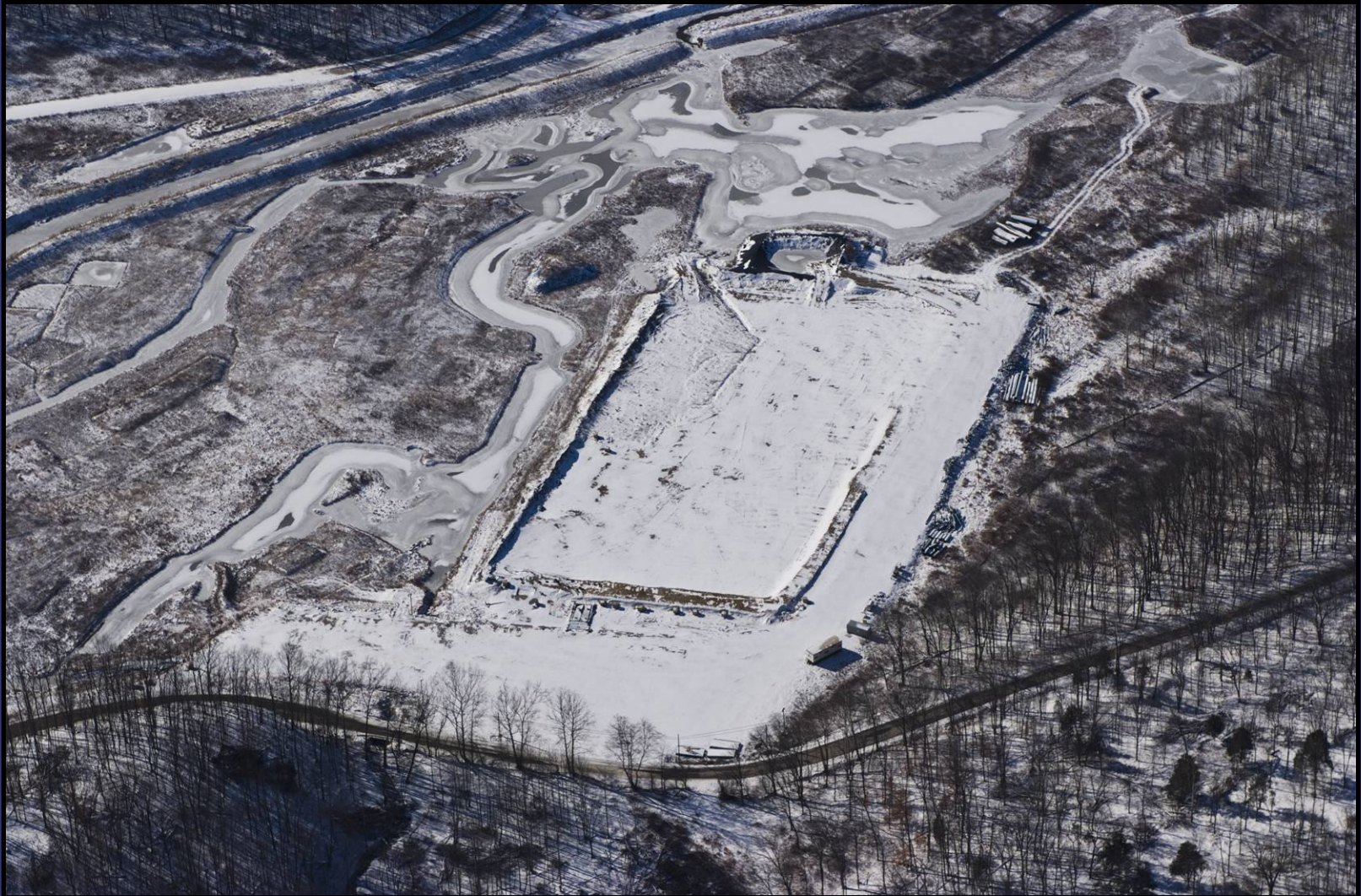
Excavation remaining west of Peerless Road
