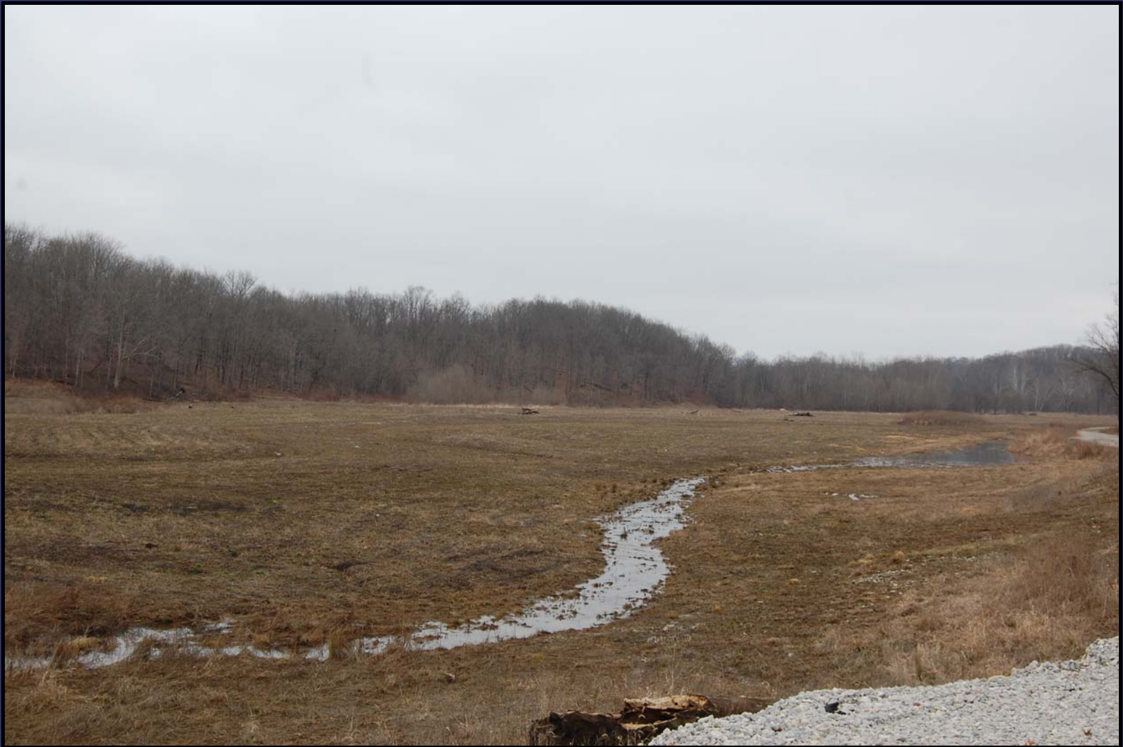
Restoration East of Peerless Road
