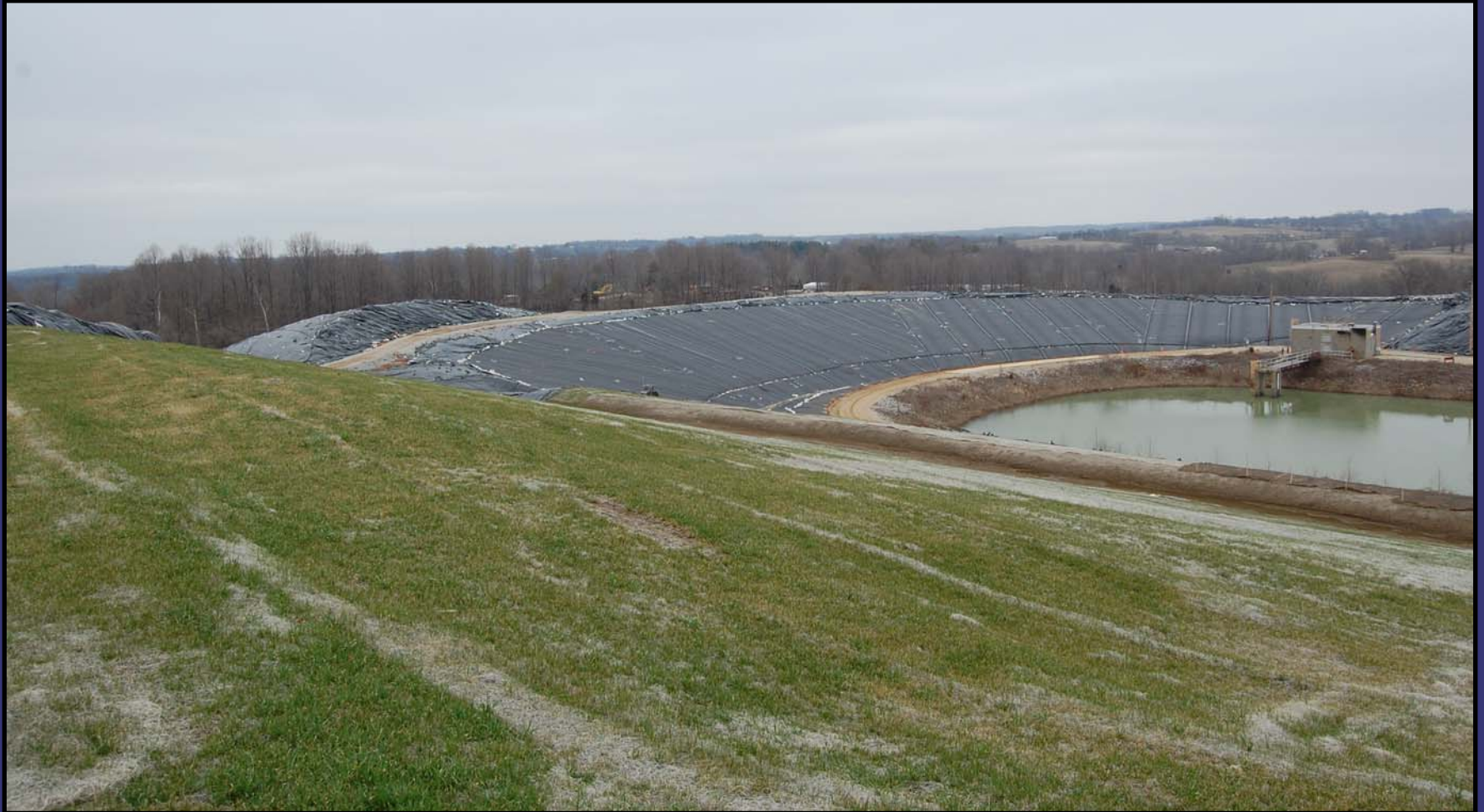
Partially completed cover work around the storm water pond.
