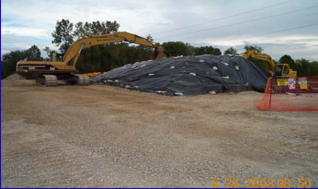
Covered soil pile on soil staging pad on AOI 4
