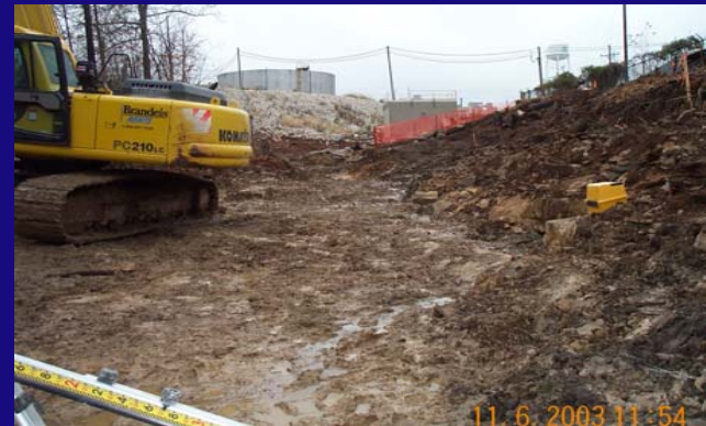
Excavated channel looking west to Outfall 002
