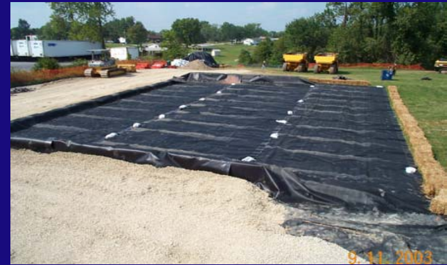
Construction of soil staging pad located east of the Zipp lot on AOI 4
