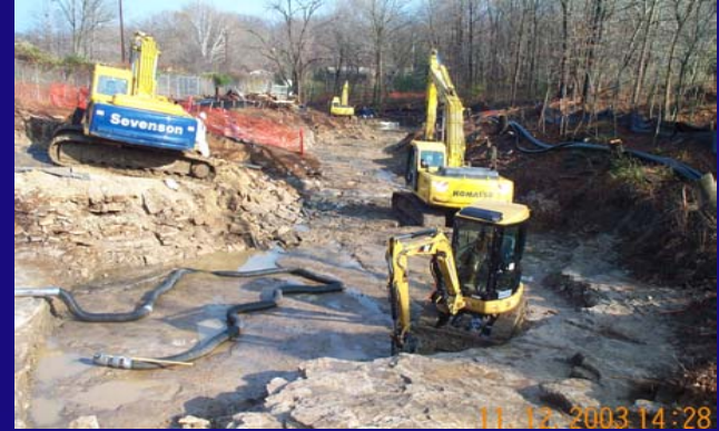
Excavated channel looking east from Outfall 002; Test trench 1 with safety fence
