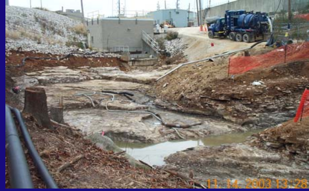
Excavated channel looking west to Outfall 002; Test trench 1 with safety fence
