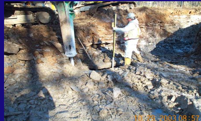
Intersection of stream channel and test trench
