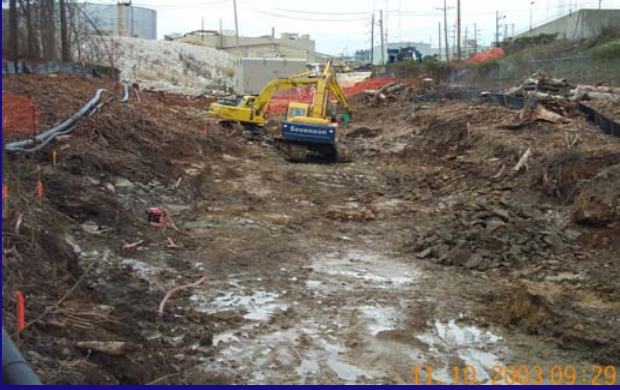
Excavated channel looking west to Outfall 002
