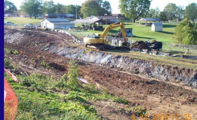
South embankment along property line of Parcel 401. Test Pit 002 being excavated.
