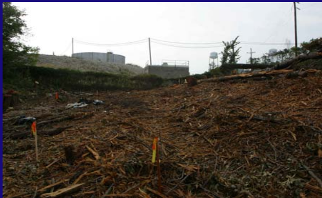
Parcel 3 cleared looking at Outfall 002
