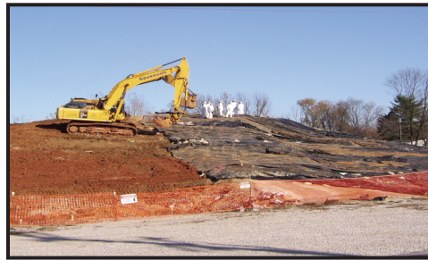
Parcel 201 Cover System Grading
