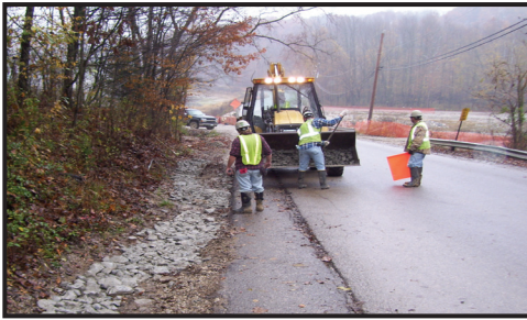
Peerless Road Shoulder Repairs
