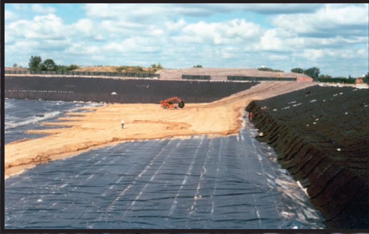
Placement of Drainage Layer over HDPE Liner
