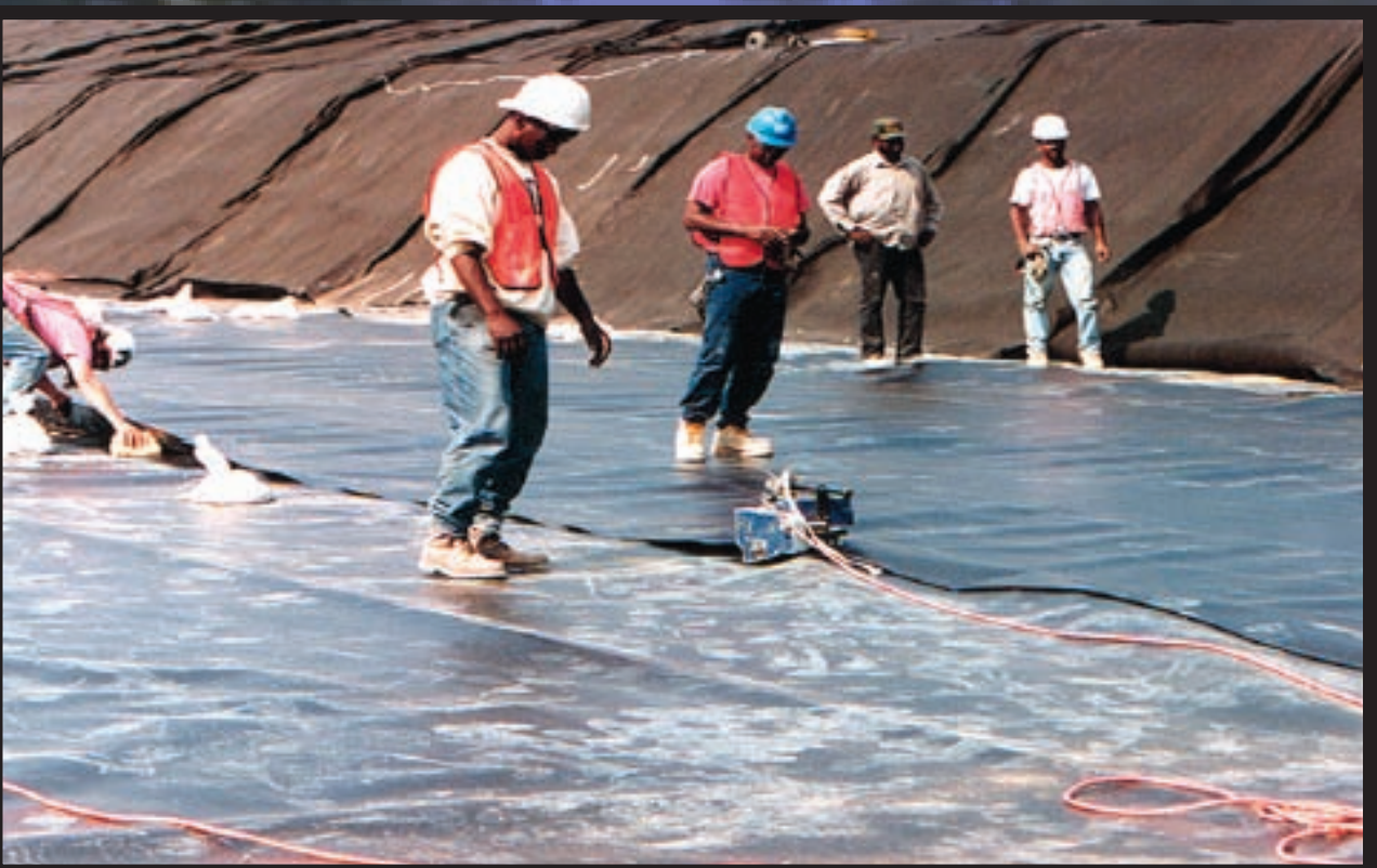
High Density Polyethylene (HDPE) Liner Seaming
