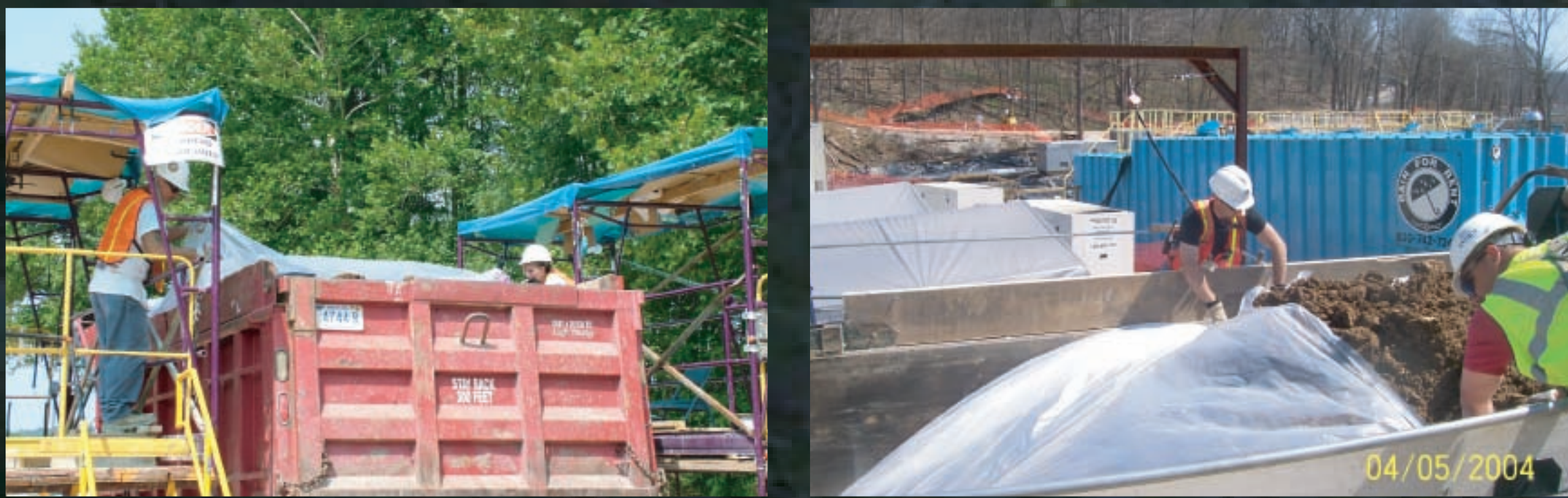
Unloading soil material containing <50 ppm PCBs into the East Plant Area.
