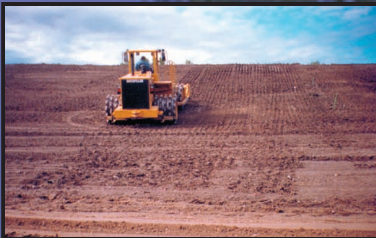
Placement of Clay Layer of Vault Cap
