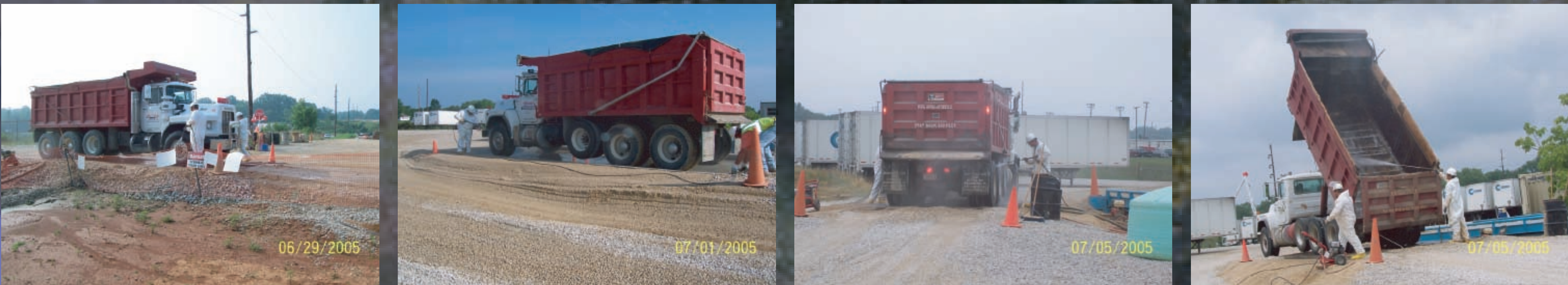
To ensure that there is no track out of potentially contaminated soil, wheel wash stations have been installed at exits from staging and grading areas. Wheels are thoroughly washed and the water is collected for treatment.
