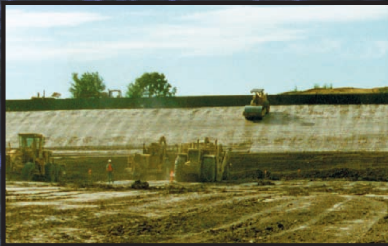
Placement of Clay Layer of Vault Cap
