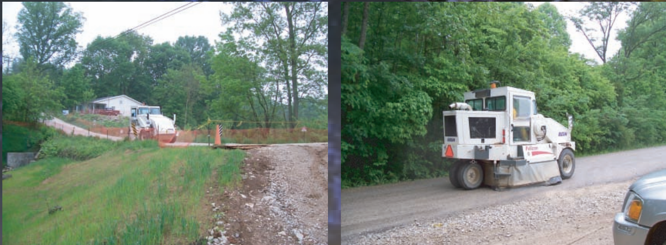
Street sweepers work throughout the day along the truck traffic routes cleaning up the everyday soil material which cars and trucks track out from parking lots and property entrance ways not associated with the project.
