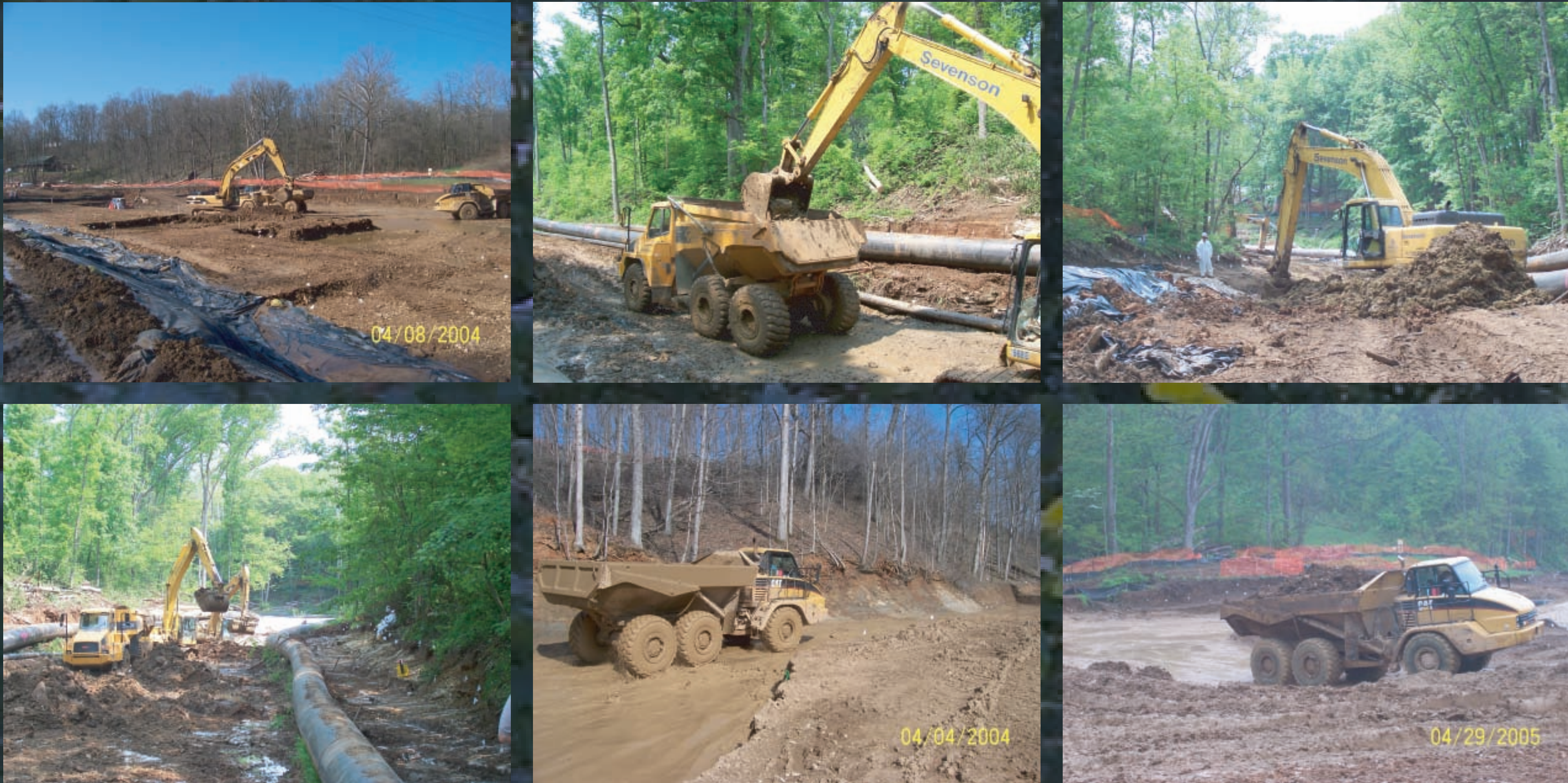
Excavation and loading soil material into off-road trucks for transportation within the excavation area.
