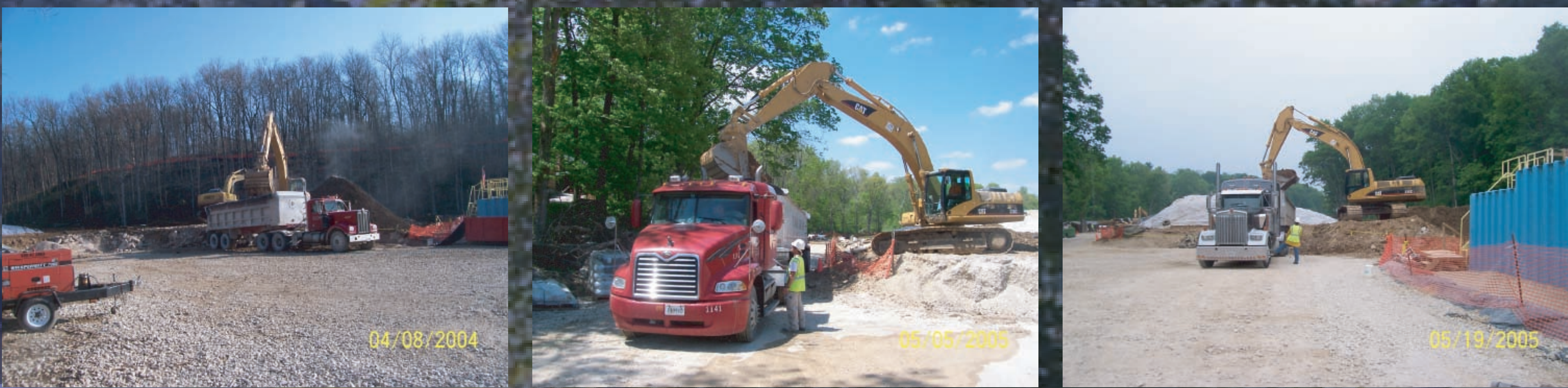
To ensure that there is no track out of potentially contaminated soil, wheel wash stations have been installed at exits from staging and grading areas. Wheels are thoroughly washed and the water is collected for treatment.
