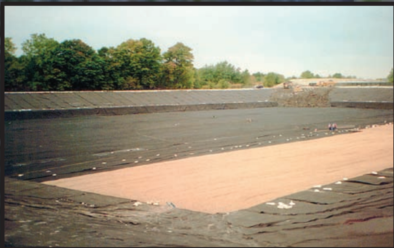
High Density Polyethylene (HDPE) Liner Placement
