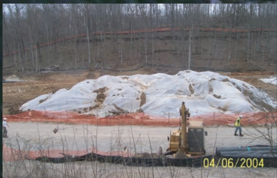
Soil material placed into staging areas is covered until sample results confirm the appropriate location for transport.
