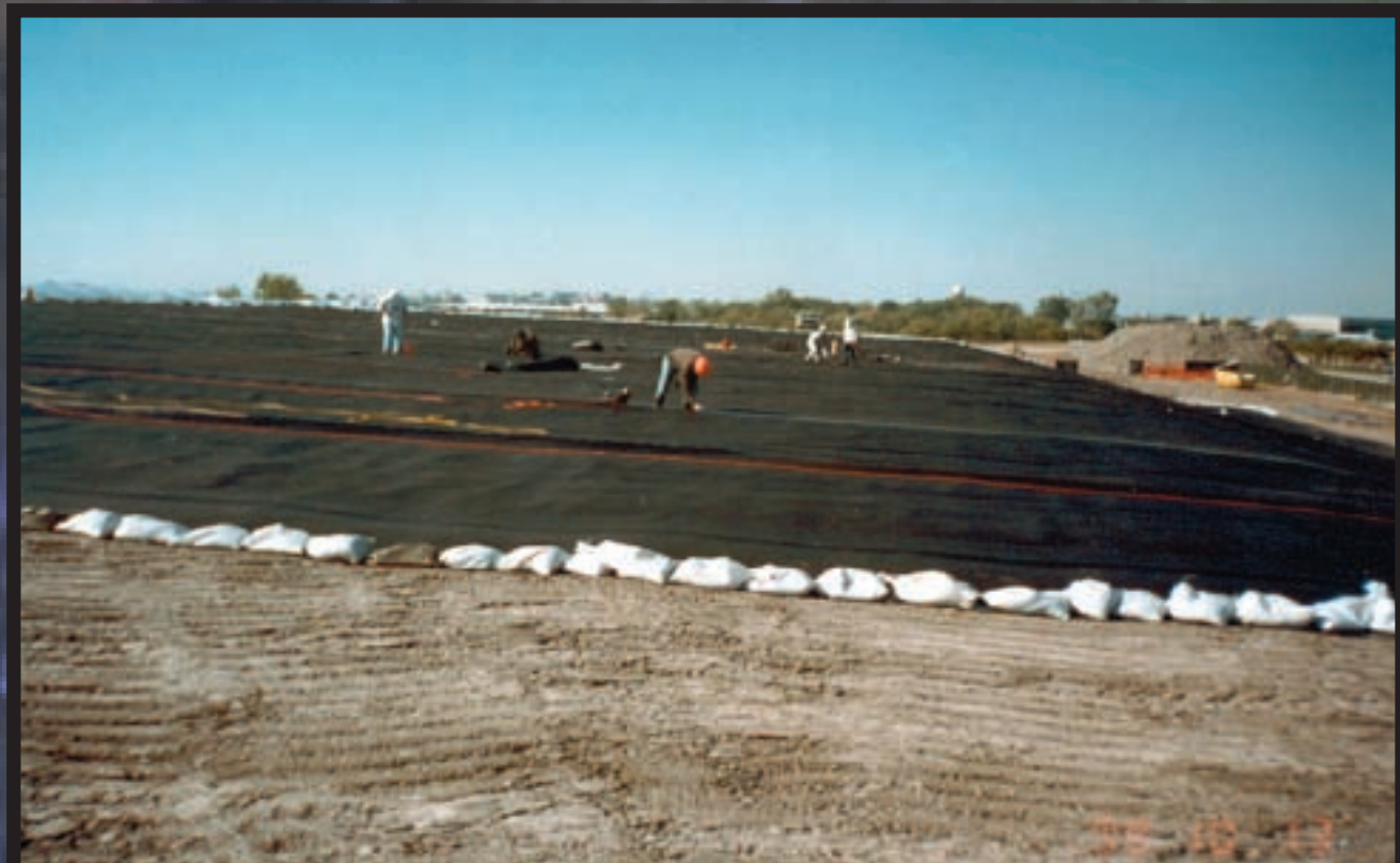
Placement of HDPE Liner as Part of Vault Cap
