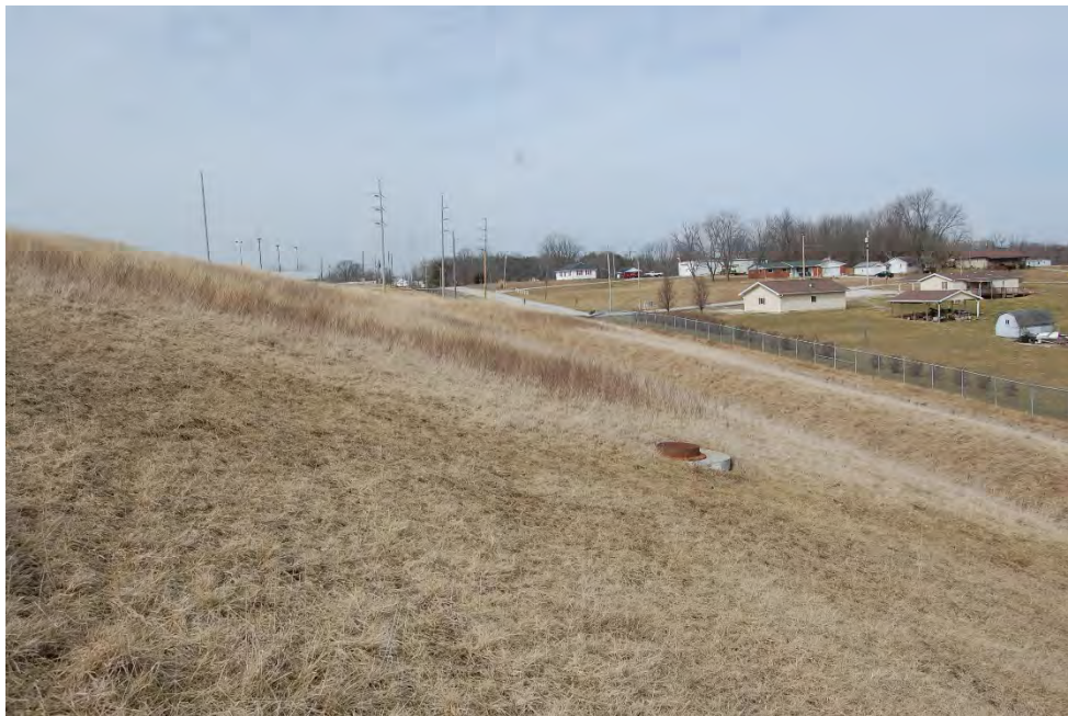
Photo 18: ES5 drainage swale on north cover facing west
