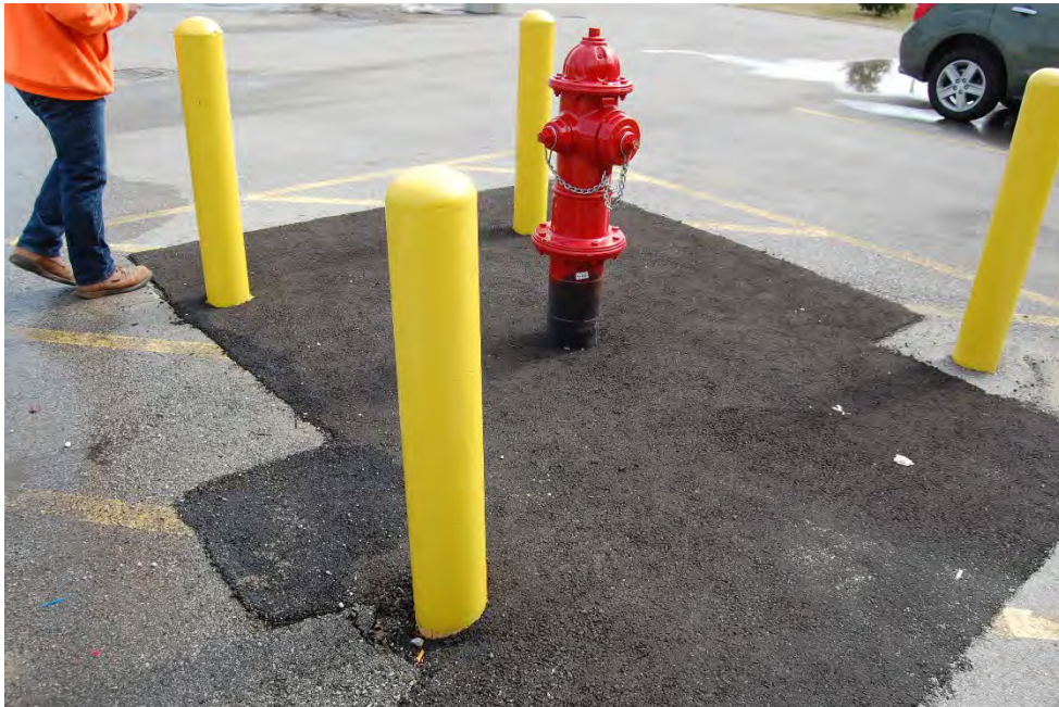
Photo 29: WA West Plant fire hydrant repair asphalt patch 2
