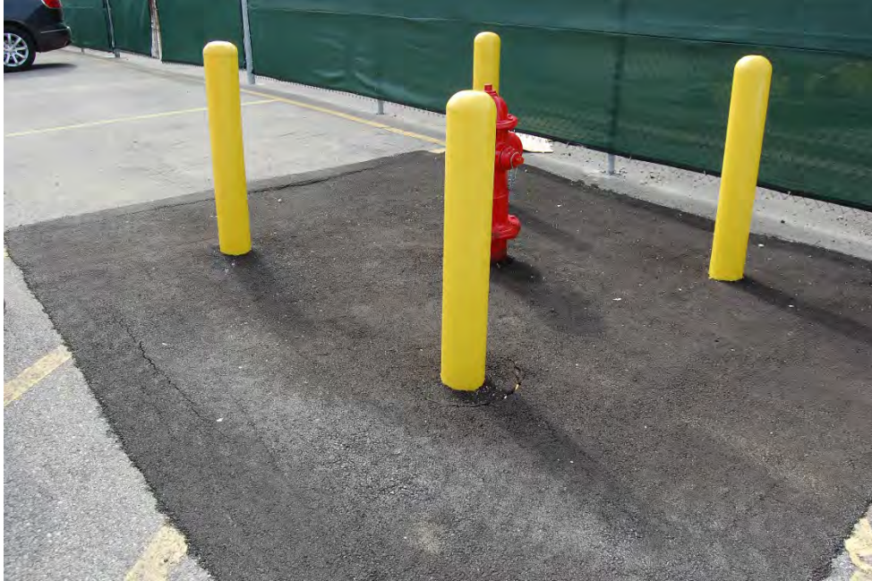
Photo 28: WA West Plant fire hydrant repair asphalt patch 1
