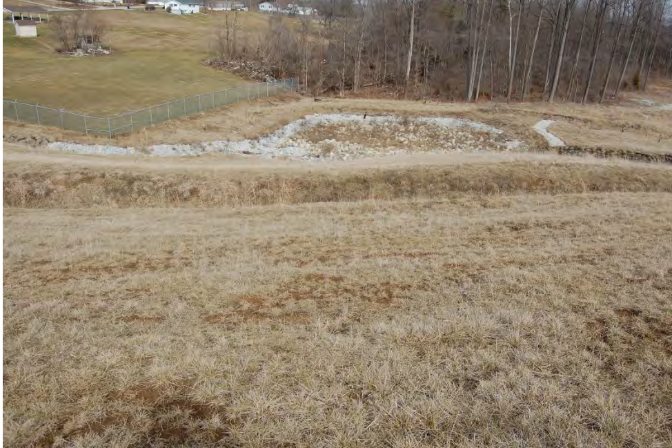
Photo 19: ES6 drainage swale on north cover facing north
