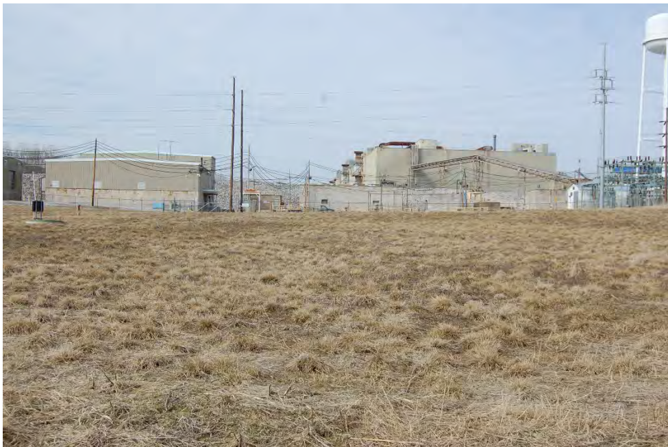
Photo 10: EV7 facing west
