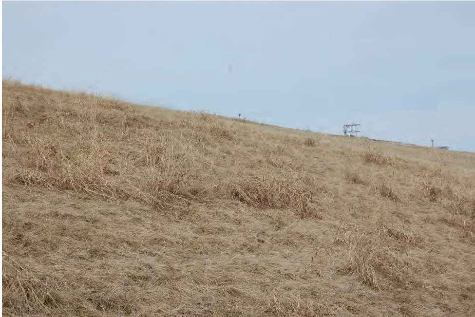
Photo 1: EV1 Vault cover facing northwest
