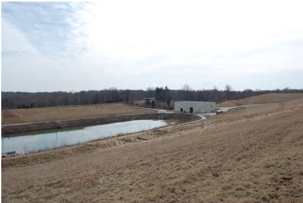
Photo 2: EV1 Vault cover (and East Plant Area cover beyond) facing southeast
