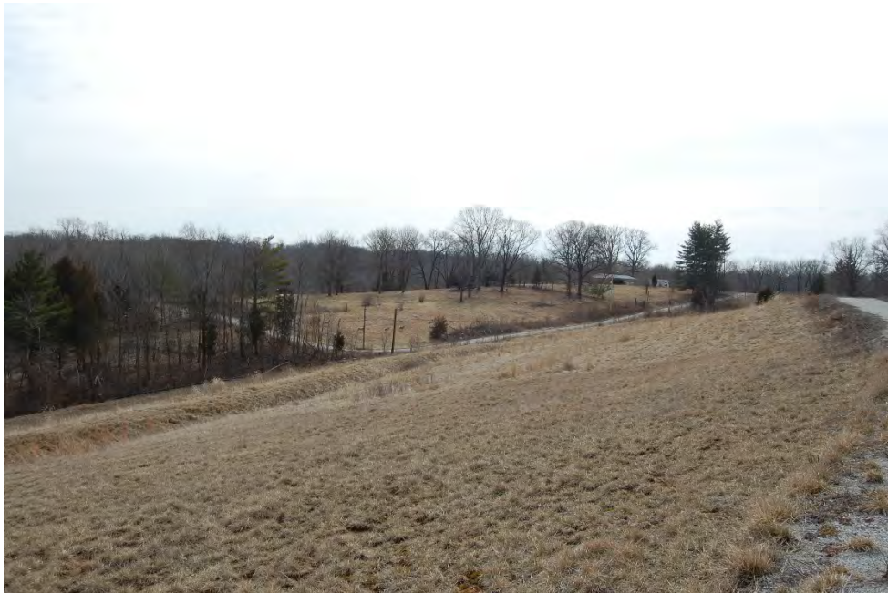
Photo 20: ES6 drainage swale on east cover facing southeast
