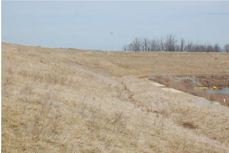
Photo 17: ES1 facing north along ditch around stormwater pond
