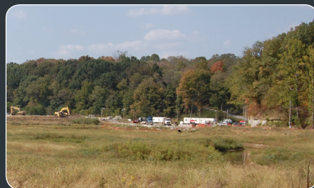
SOIL PILE REMOVAL ACTIVITIES WEST OF PEERLESS ROAD.
