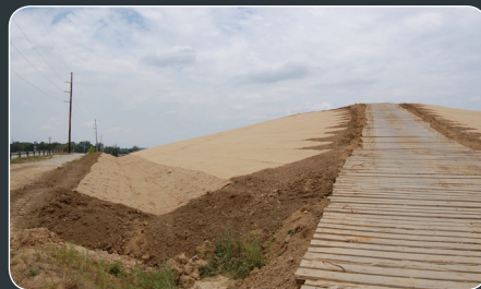
COVER SYSTEM CONSTRUCTION NEARING COMPLETION ALONG GM DRIVE.
