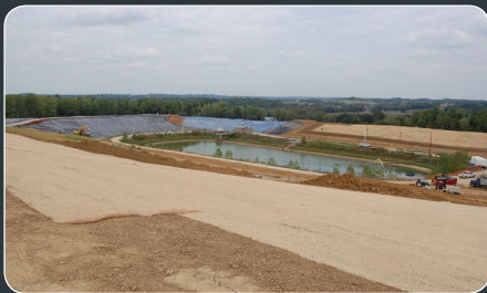
LOOKING NORTHEAST AT THE STORM WATER MANAGEMENT POND.
