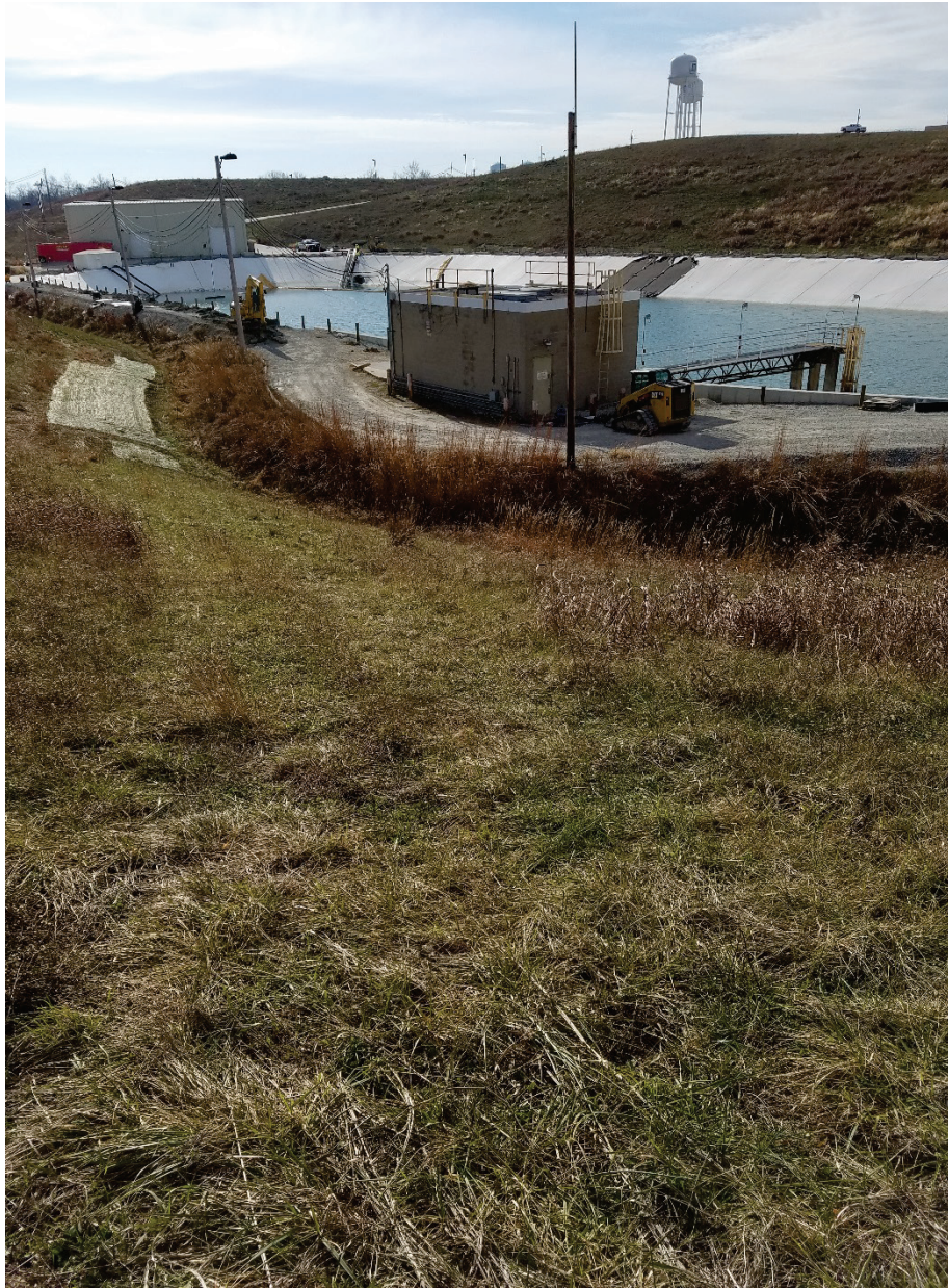
Photo 10: Vegetation along EV4 East Plant Area Cover facing southwest
