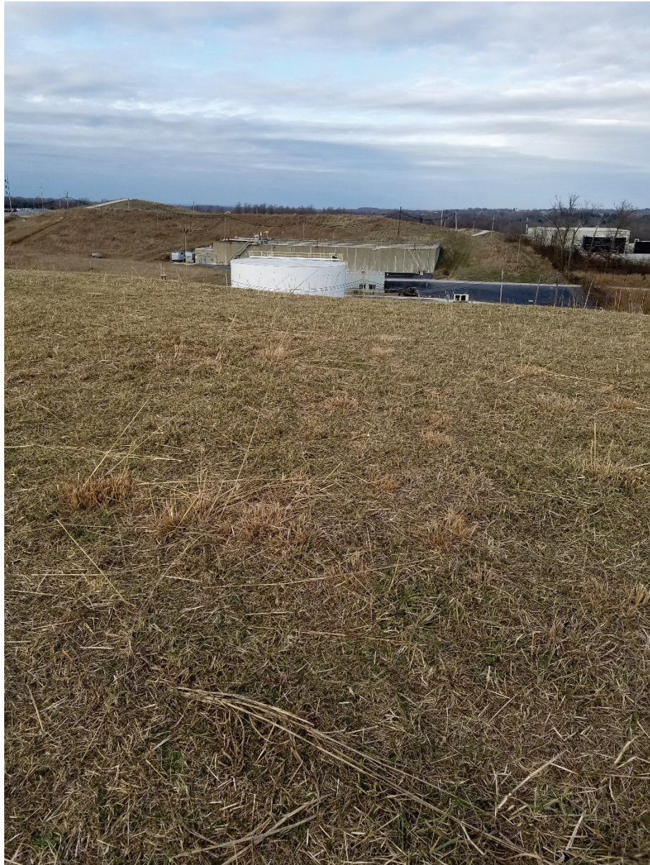
Photo 18: East Plant Area Cover overview facing north.
