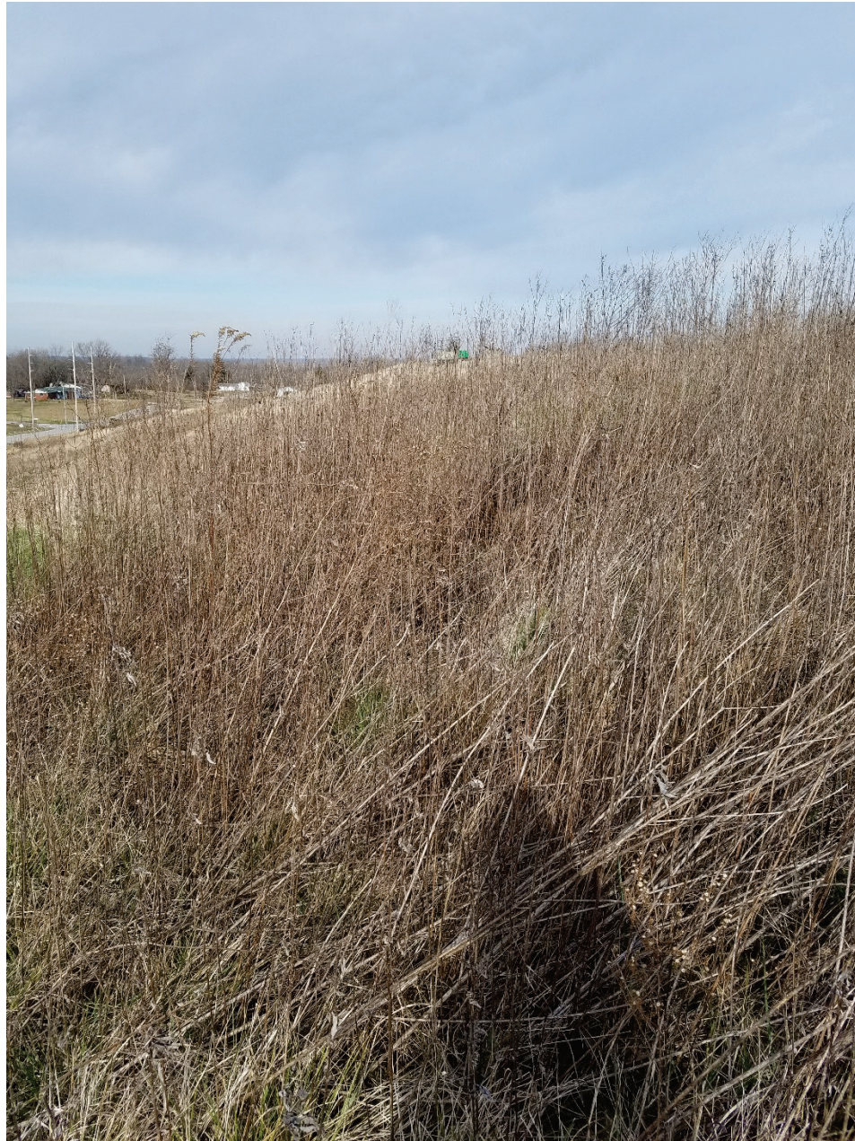
Photo 11: ES3 East Plant Cover System facing north
