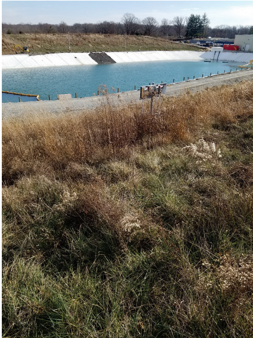
Photo 6: EV2 East Plant Area Cover facing southeast towards pond
