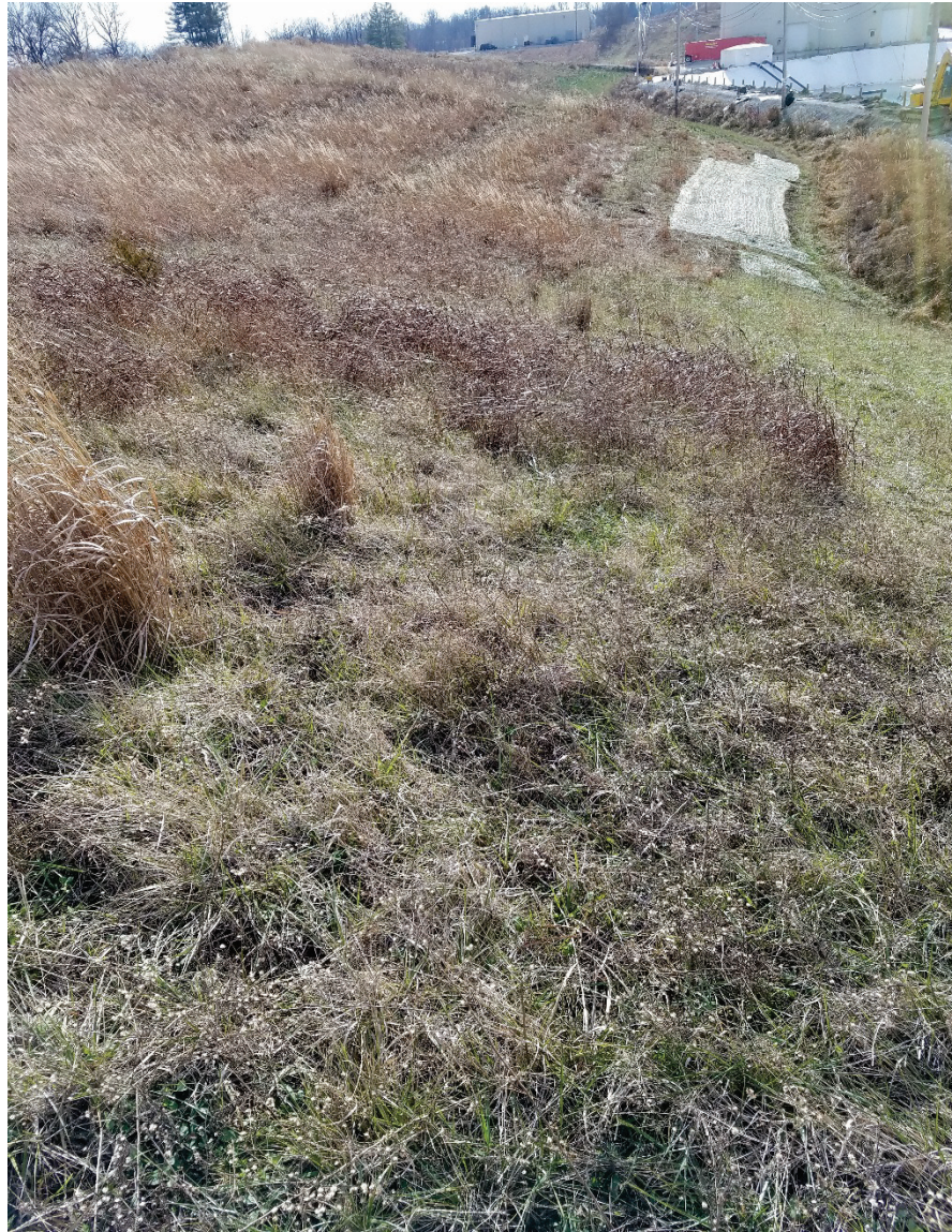
Photo 12: EV4 East Plant Area Cover erosion repairs.
