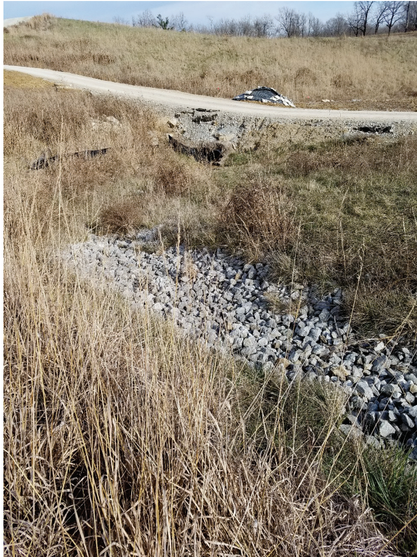
Photo 7: Drainage at ES12 facing northeast.
