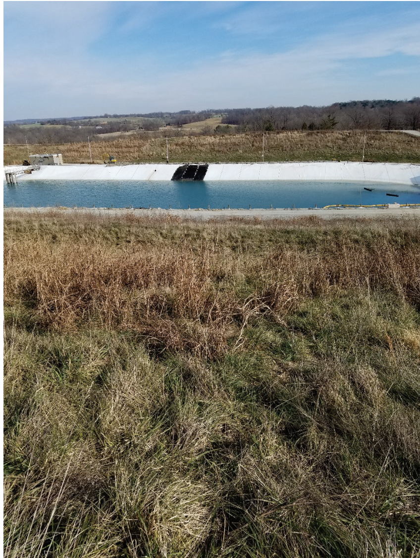
Photo 2: EV1 Vault Cover facing east toward pond
