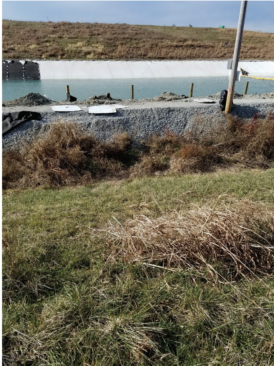
Photo 13: Vegetation south of EV5, facing pond
