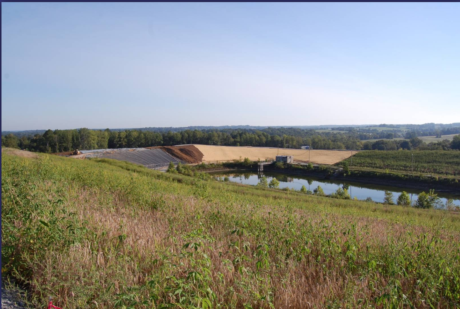
Completed and partially completed cover work around the storm water pond.
