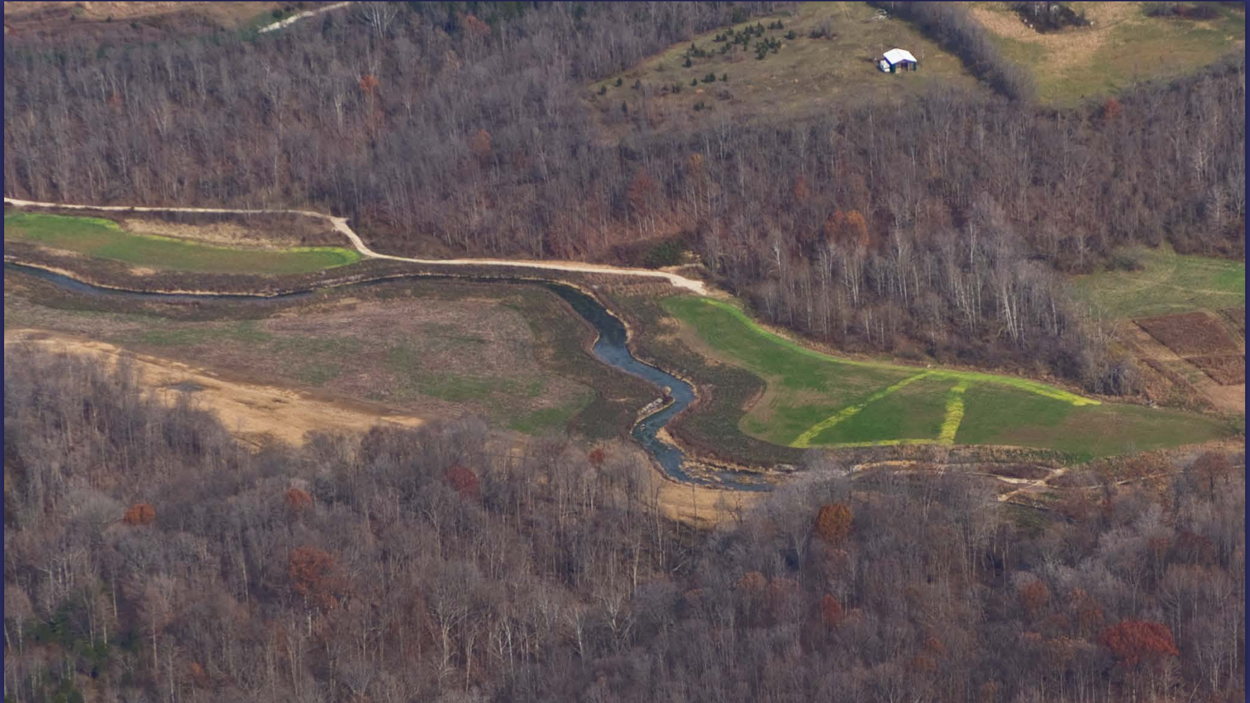
Restoration east of Peerless Road
