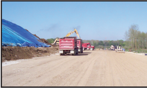
Truck Load-Out At Area G
