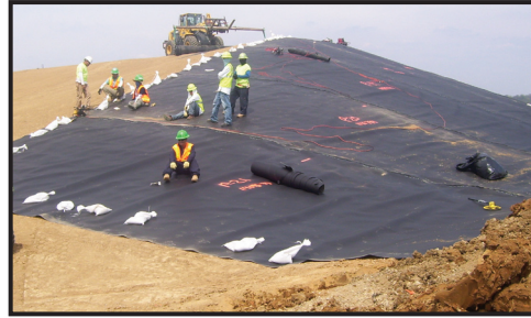
Vault Cover Liner Placement
