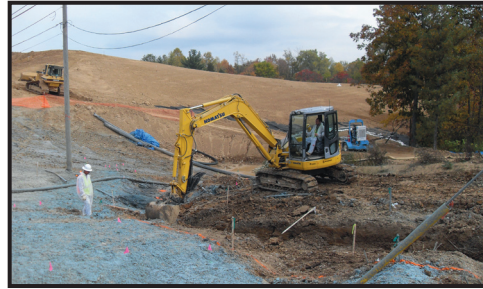
Drainage Ditch Installation
