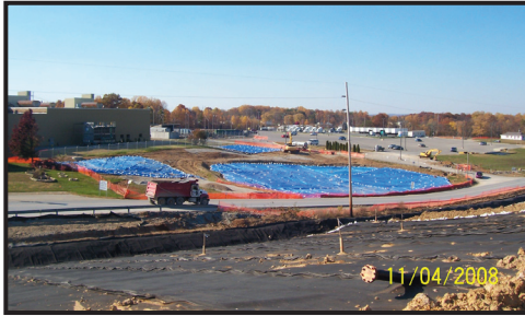
Backfilled West Plant Area Removal
