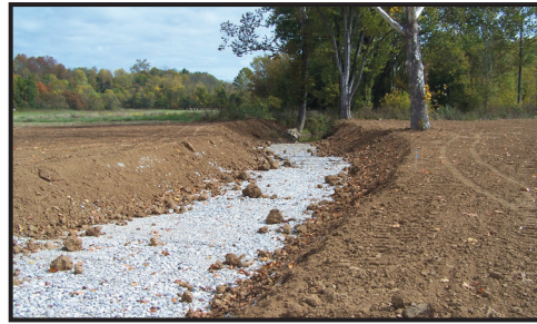
Channel Restoration Upstream of Peerless Road
