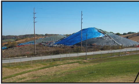
Restored Sewer Abandonment Area
