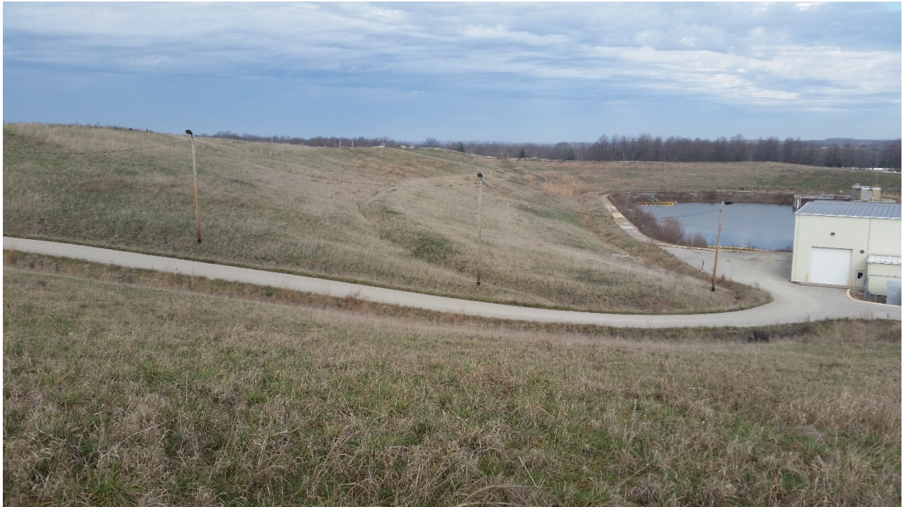
Photo 20: ES1 and ES2 drainage swale facing north.
