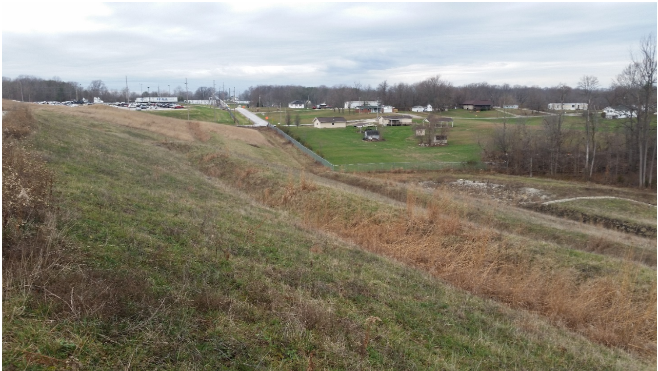
Photo 22: ES4 drainage swale facing west.
