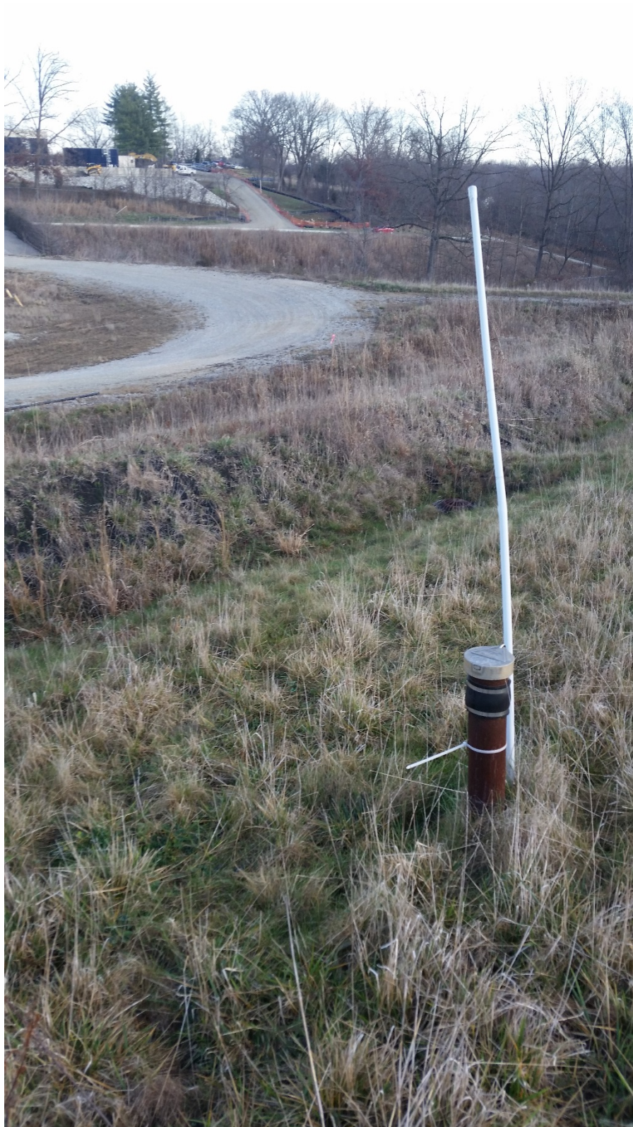
Photo 32: ES14 drainage swale facing northeast.
