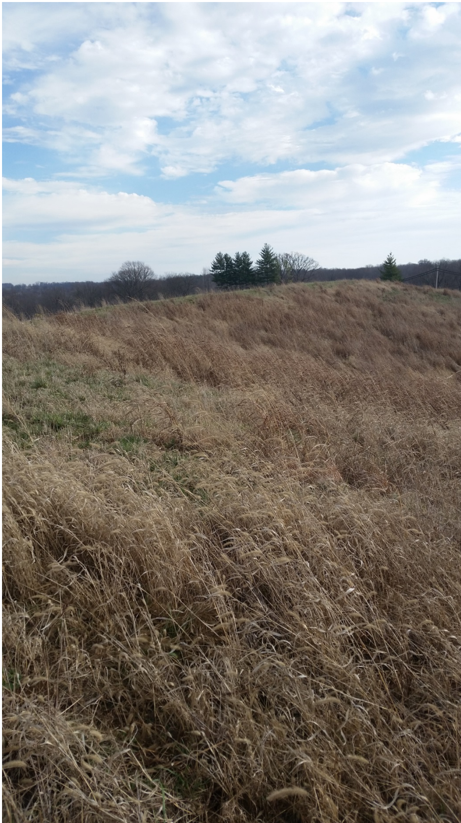
Photo 9: EV6 East Plant Area cover facing east.
