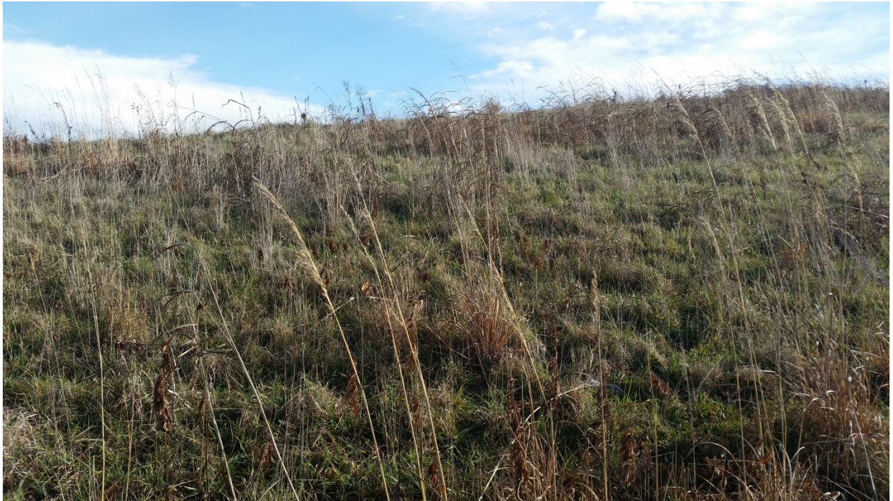
Photo 17: EV9 East Plant Area cover facing south.
