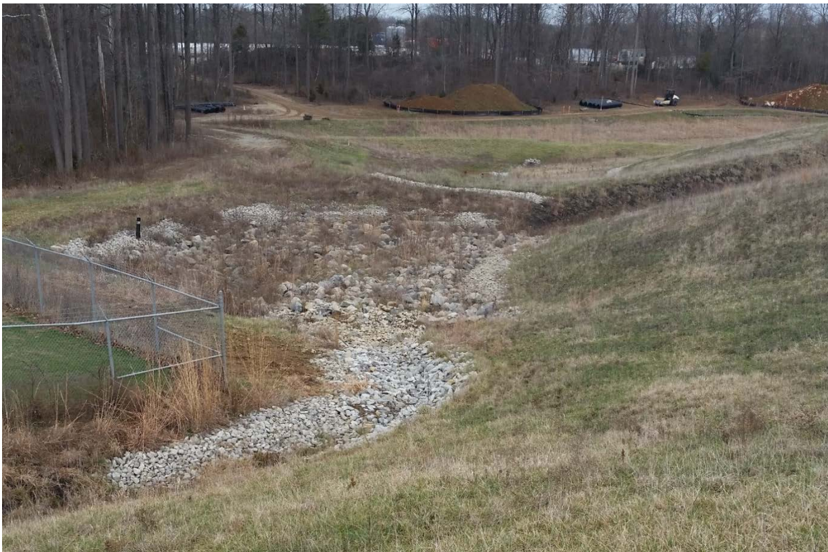
Photo 27: ES6 drainage swale facing east, repaired channel erosion.
