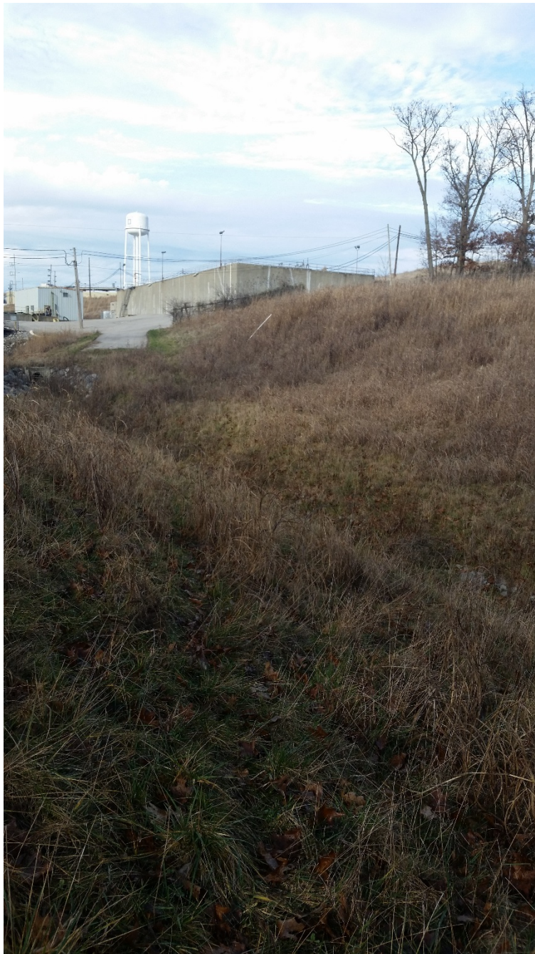
Photo 30: ES13 detention basin 6 facing west.
