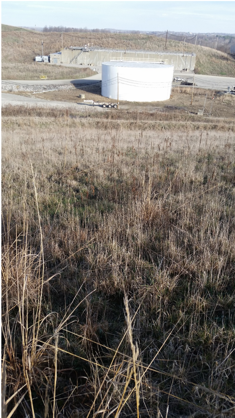
Photo 18: EV9 East Plant Area cover facing north.
