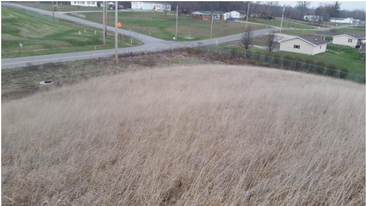
Photo 4: EV2 East Plant Area cover facing northwest.
