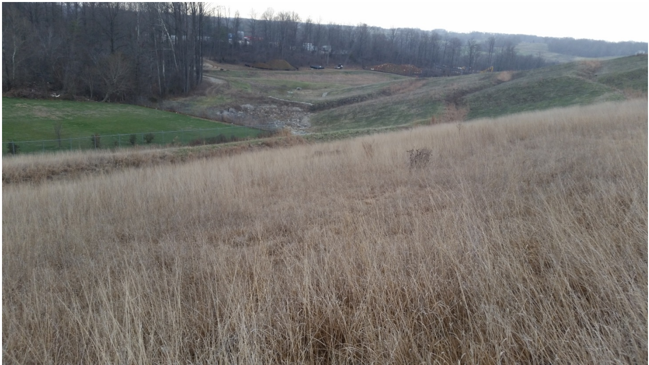
Photo 24: ES5 drainage swale facing northeast.
