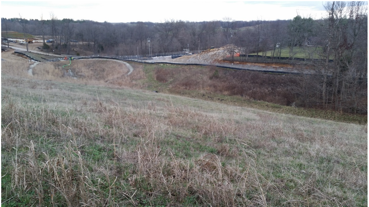
Photo 8: EV5 East Plant Area cover facing northeast.
