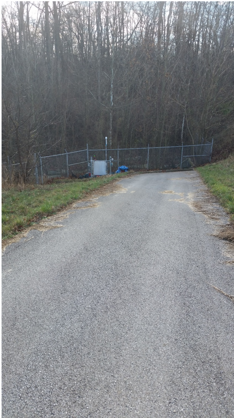
Photo 15: EV8 East Plant Area cover (Parcel 205) facing south.
