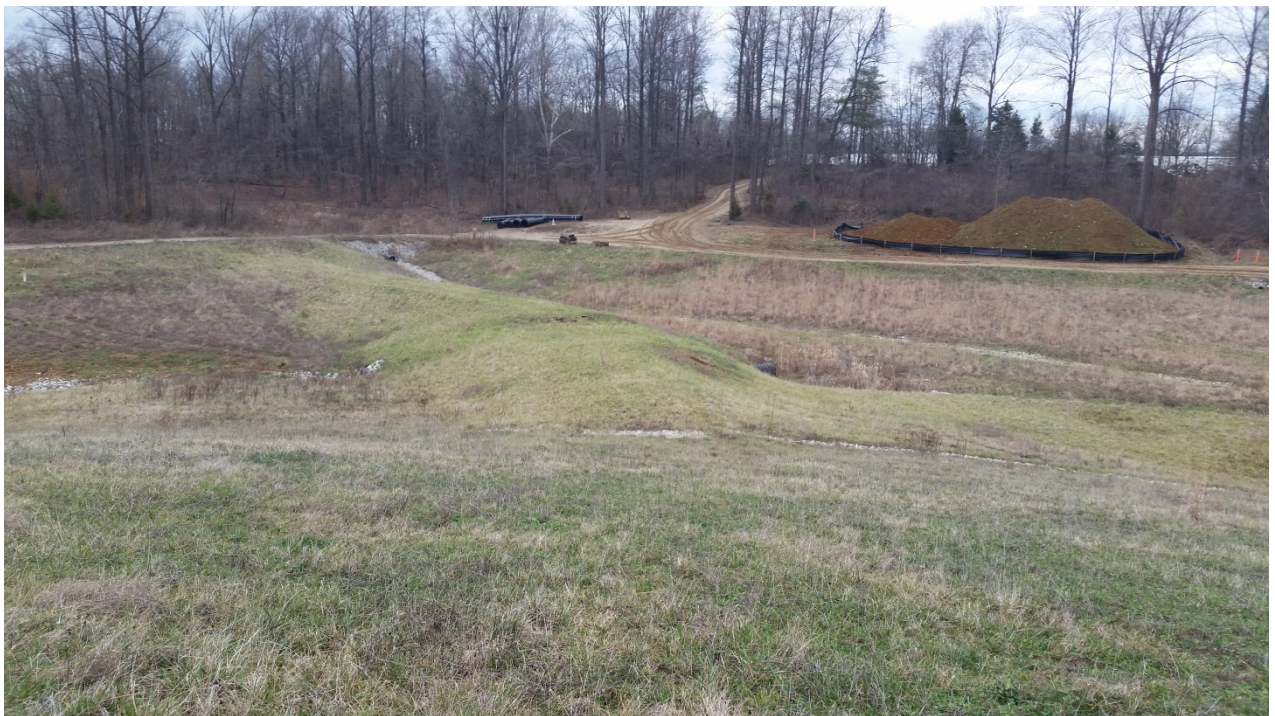
Photo 5: EV3 East Plant Area cover facing north.
