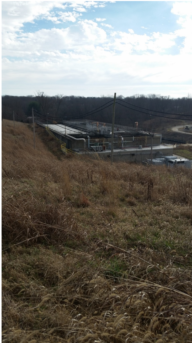
Photo 11: EV6 East Plant Area cover facing southeast.
