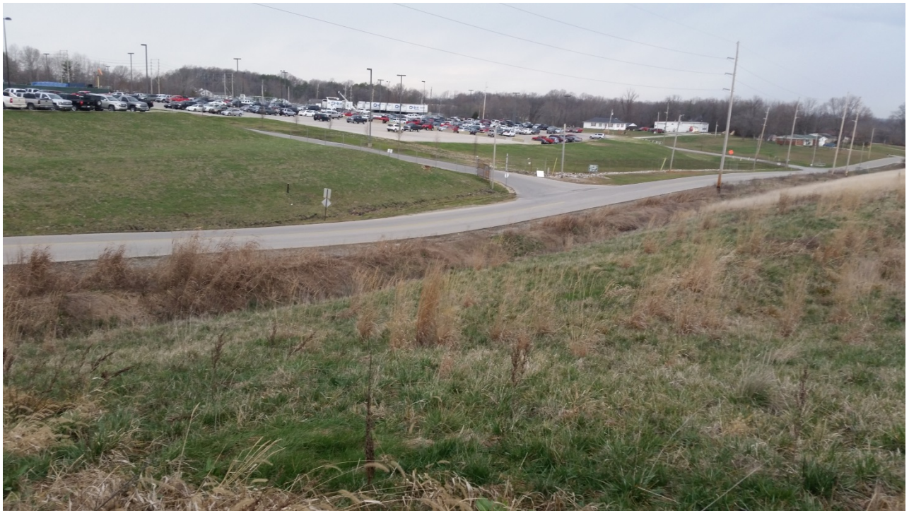
Photo 1: EV1 Vault cover facing northwest.
