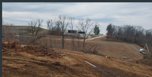
TREE CLEARING FOR PHASE 2 OF TRENCH ALIGNMENT
