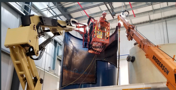
OLD GROUNDWATER TREATMENT SYSTEM DECOMMISSIONING WORK
