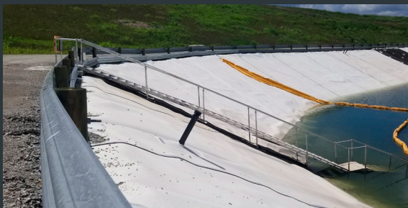
GUARD RAIL AT STORMWATER POND
