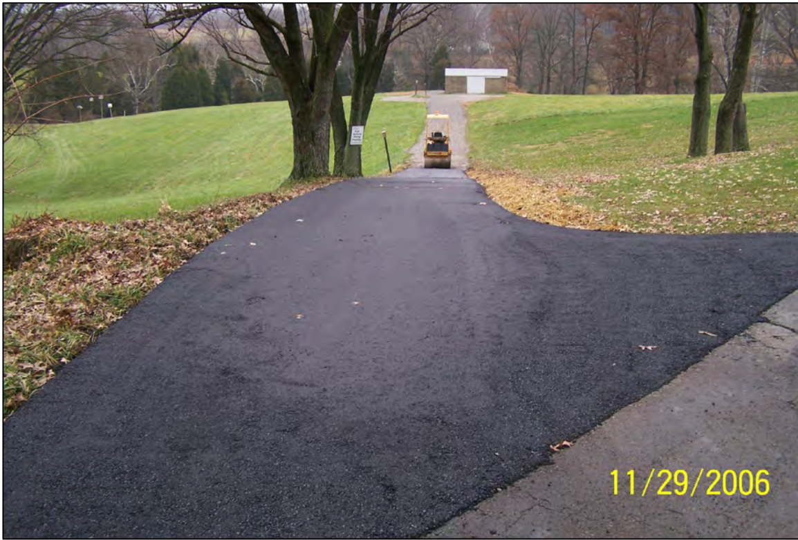
PHOTO 41: PARCEL 60 - REPAVED DRIVEWAY (FACING NORTH). NOVEMBER 2006
