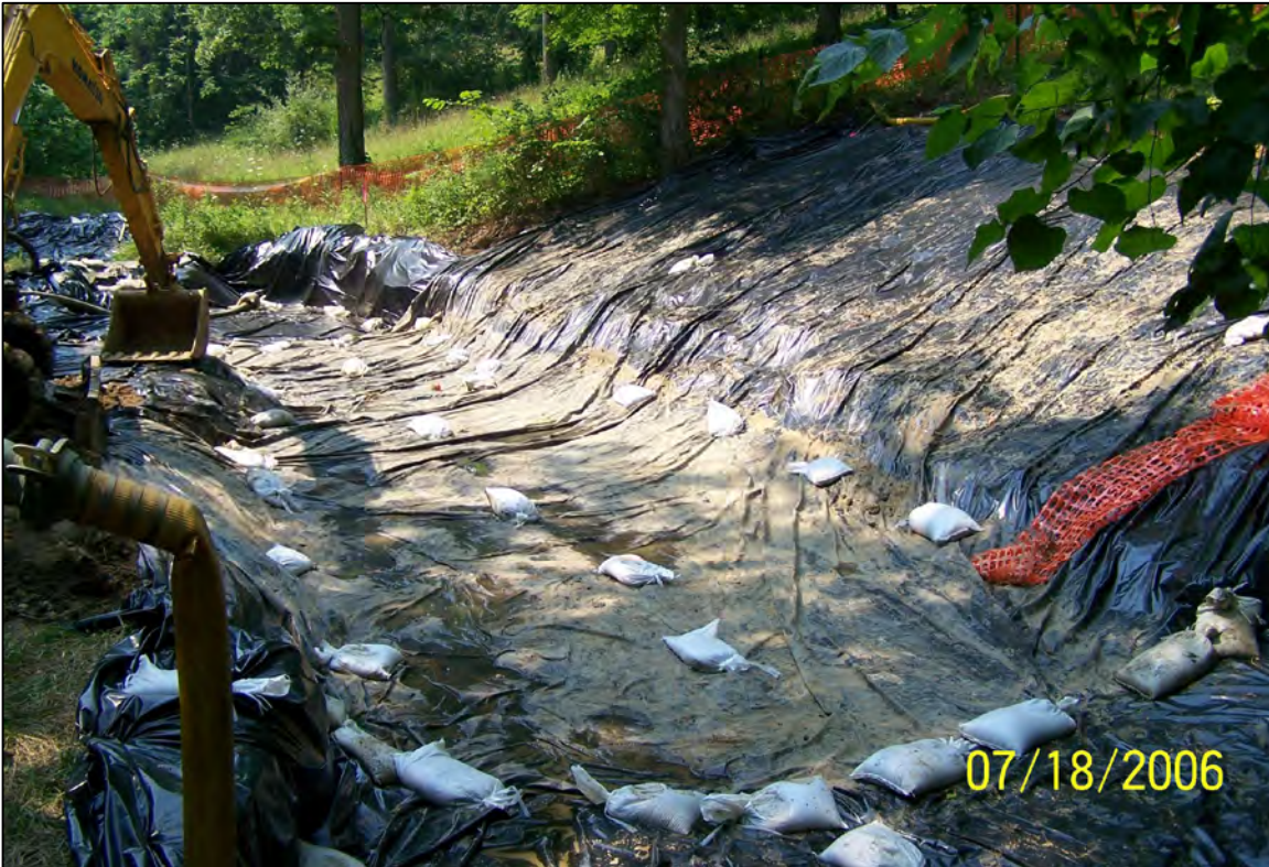
PHOTO 30: PARCEL 60 & 61 - EXCAVATION AREA TARPED (FACING WEST). JULY 2006
