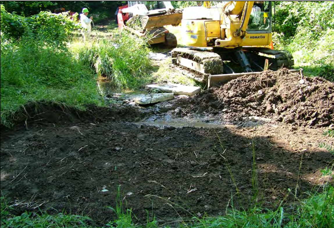
PHOTO 26: PARCEL 60 - EXCAVATION PROGRESS IN STREAM (FACING SOUTHEAST). JUNE 2006
