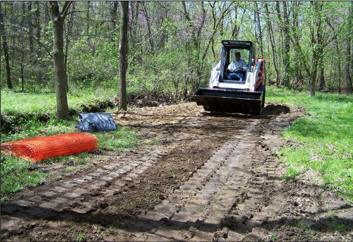
PHOTO 23: PARCEL 57 - GRADING THE RESTORED AREA PRIOR TO SEEDING (FACING WEST). APRIL 2006
