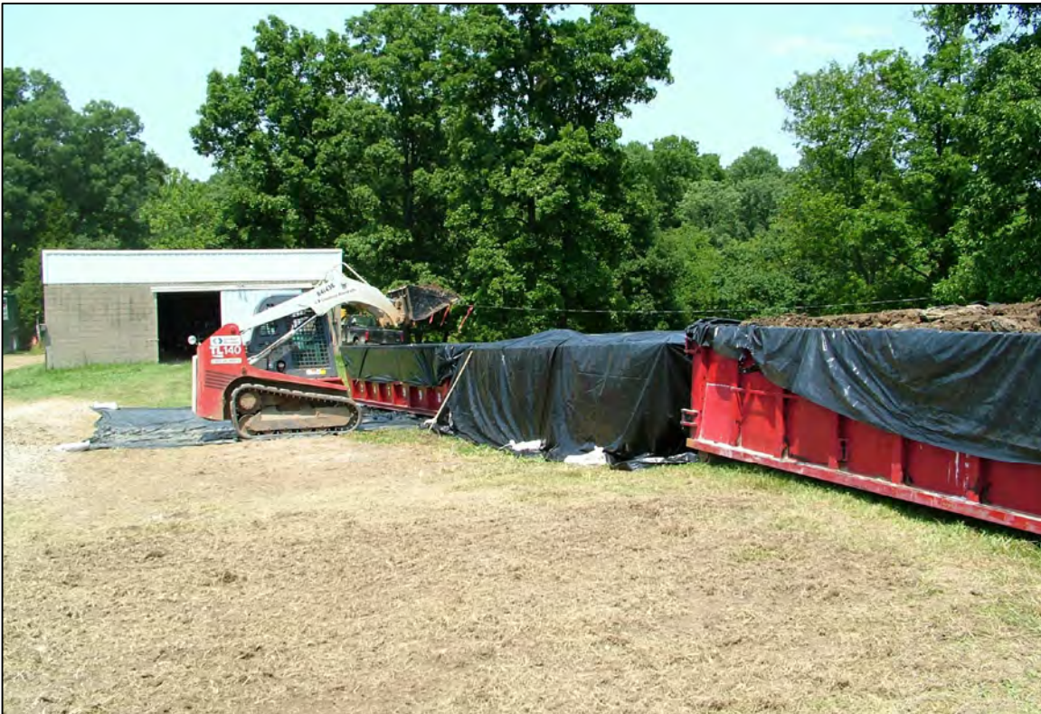
PHOTO 28: PARCEL 61 - LOADING ROLL-OFF BOX WITH EXCAVATED CREEK MATERIAL (FACING NORTH) JULY 2006
