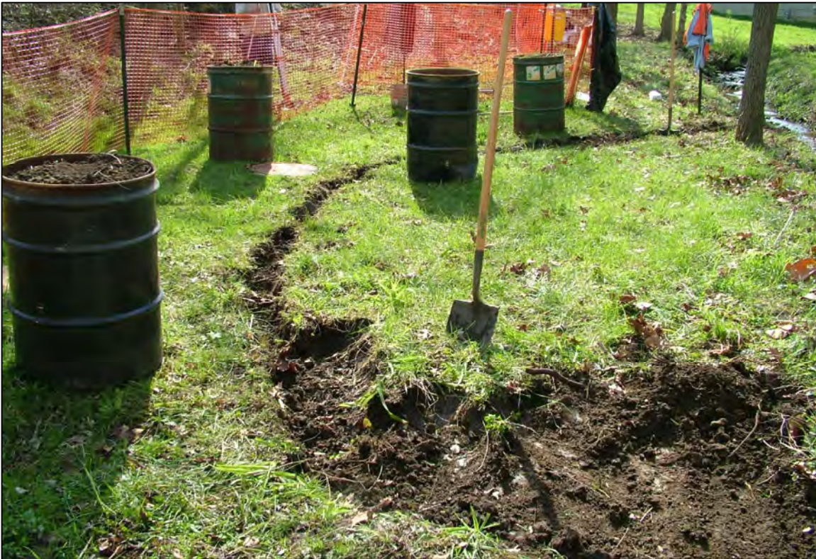
PHOTO 20: PARCEL 57 - LIMITS OF INITIAL EXCAVATION (FACING EAST). APRIL 2006
