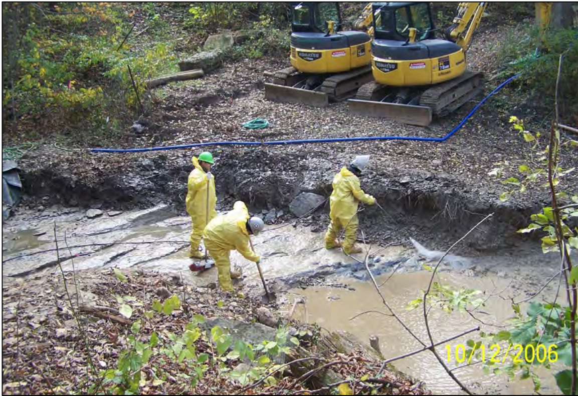
PHOTO 33: PARCEL 60 - POWERWASHING THE EXPOSED BEDROCK ALONG THE CREEK (FACING EAST). OCTOBER 2006
