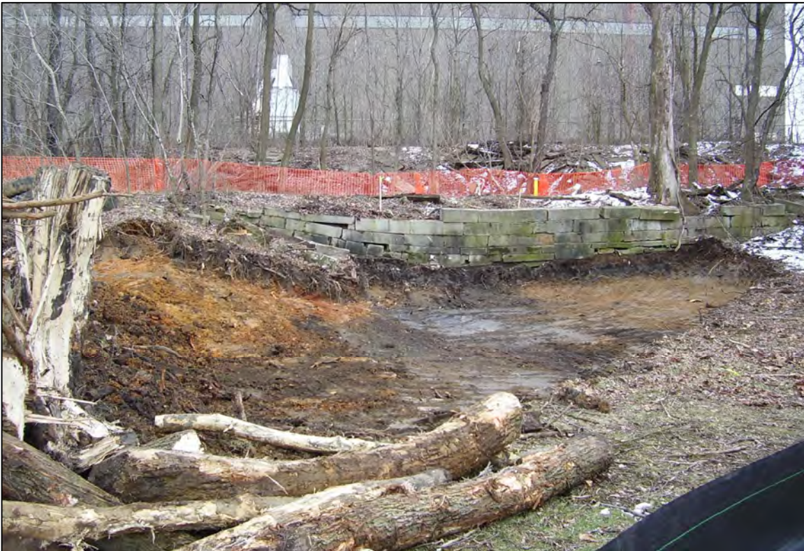
PHOTO 06: PARCEL 2 - EXCAVATION PROGRESS (FACING EAST). FEBRUARY 2006
