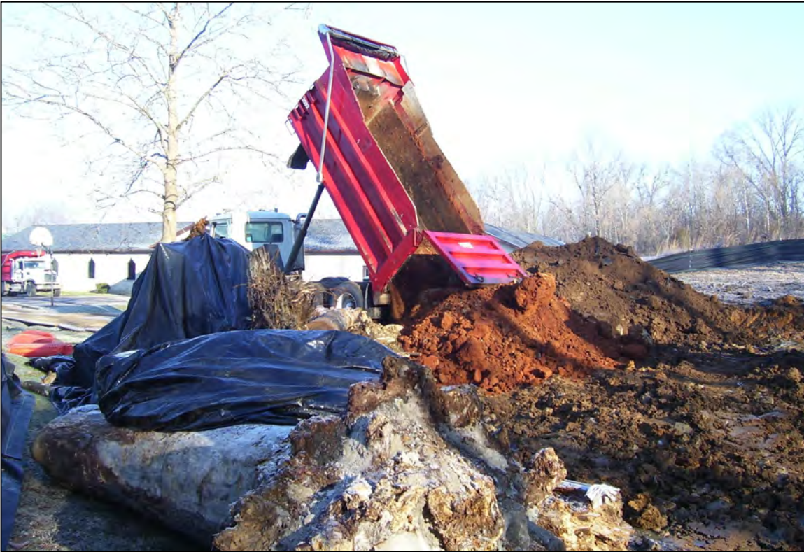
PHOTO 09: PARCEL 2 - IMPORTED FILL MATERIAL FOR RESTORATION (FACING WEST). FEBRUARY 2006
