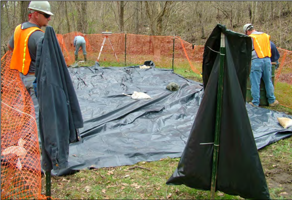
PHOTO 22: PARCEL 57 - TARPING OF THE EXCAVATION (FACING WEST). APRIL 2006
