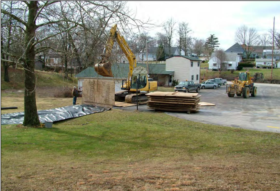
PHOTO 03: PARCEL 2 - EXCAVATION PREPARATION TO PROTECT THE LAWN (FACING WEST). FEBRUARY 2006
