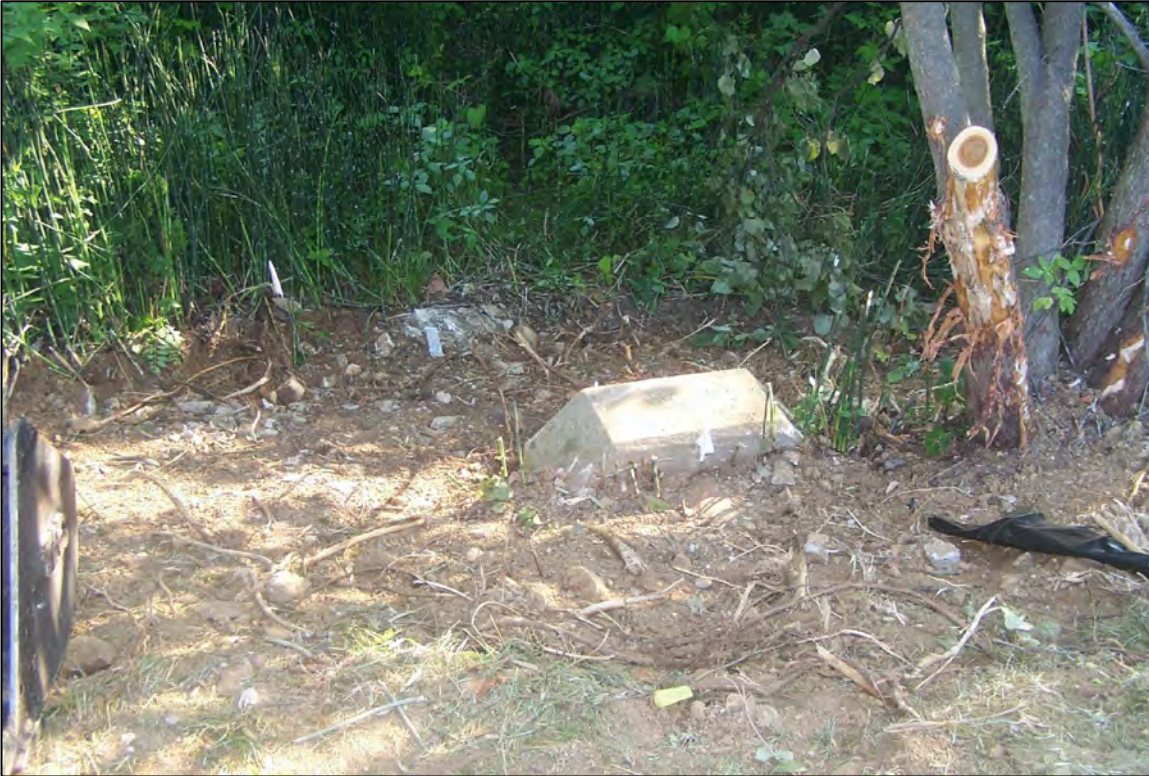
PHOTO 13: PARCEL 53 - EXCAVATION AREA (FACING NORTH). JUNE 2007
