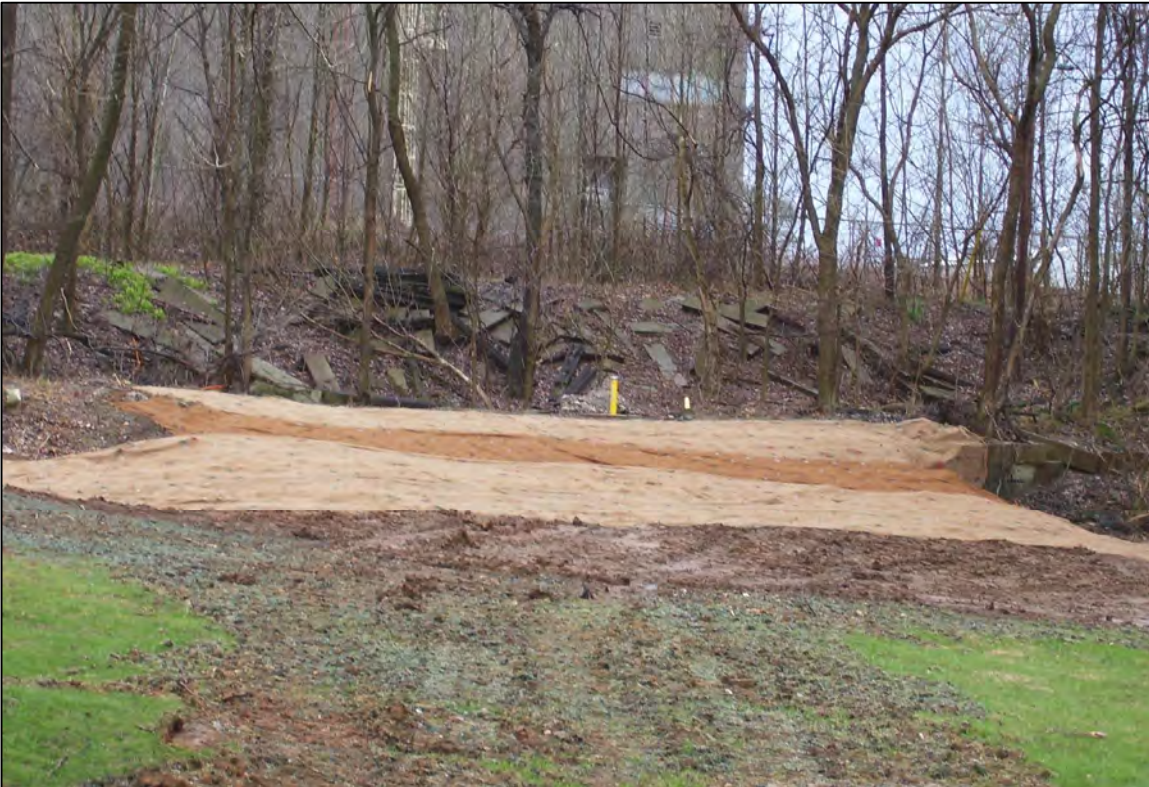
PHOTO 11: PARCEL 2 - EROSION CONTROL MATING PLACED OVER RESTORATION (FACING EAST). MARCH 2006
