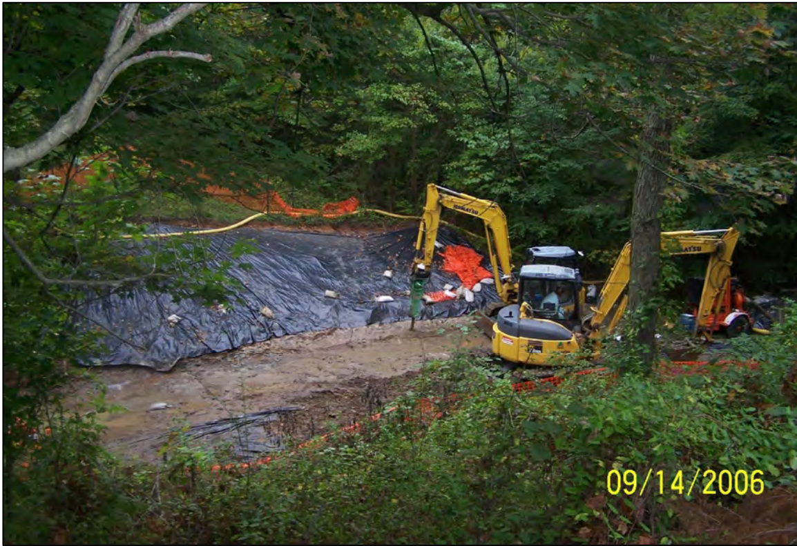
PHOTO 31: PARCEL 60 - BREAKING OUT ROCK IN THE CREEK (FACING NORTHEAST) SEPTEMBER 2006
