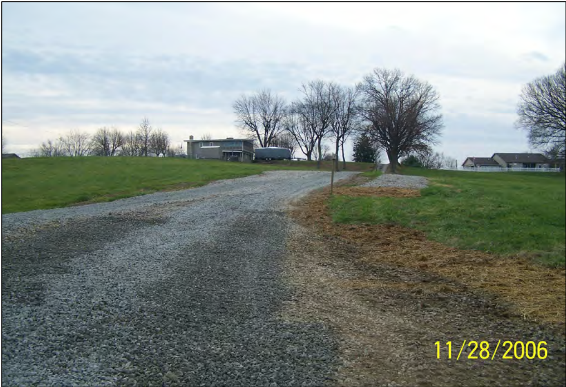
PHOTO 40: PARCEL 60 - RESTORED DRIVEWAY (FACING SOUTH). NOVEMBER 2006
