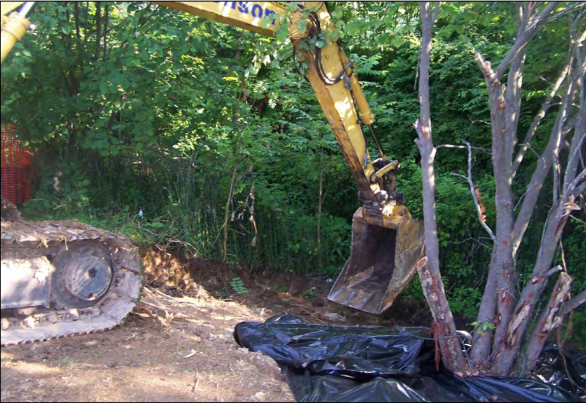
PHOTO 14: PARCEL 53 - EXCAVATION PROGRESS (FACING NORTHWEST). JUNE 2007
