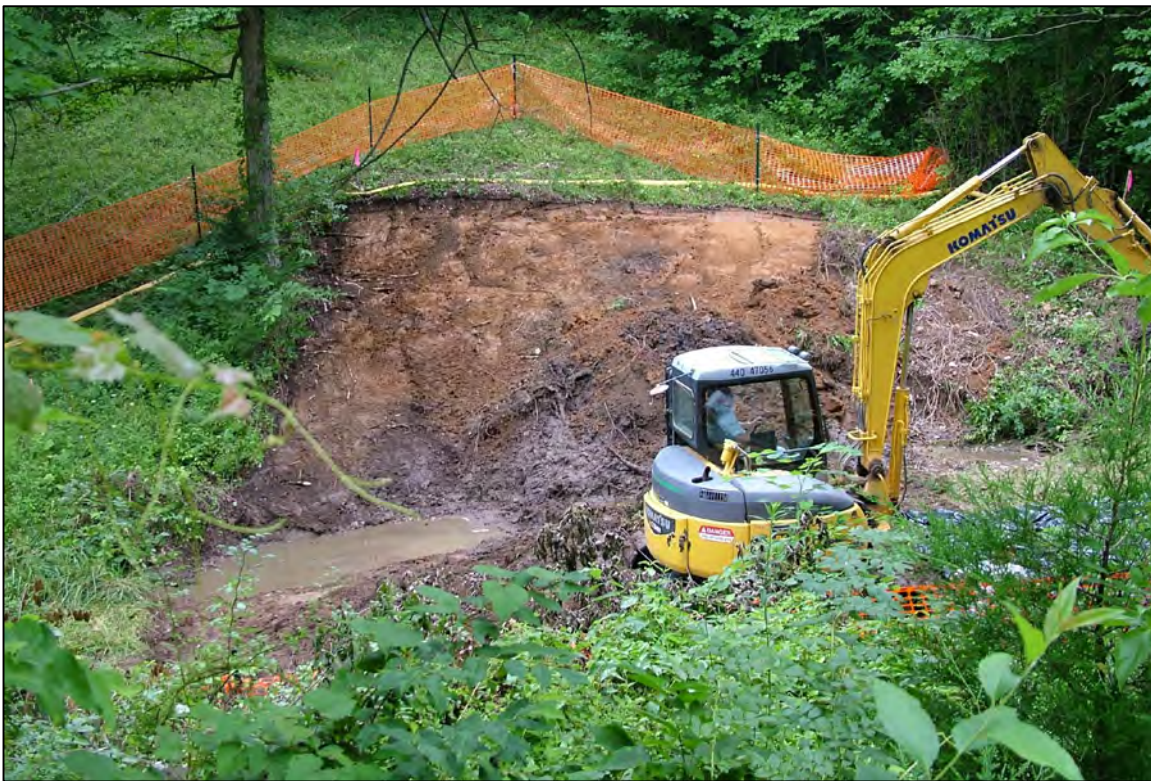
PHOTO 27: PARCEL 60 - EXCAVATION PROGRESS ON BANK (FACING NORTH). JULY 2006
