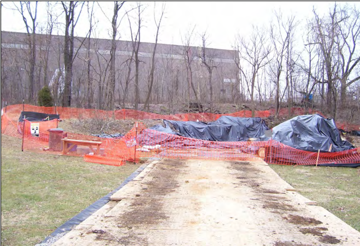
PHOTO 08: PARCEL 2 - TARPED EXCAVATION AREA (FACING EAST). FEBRUARY 2006
