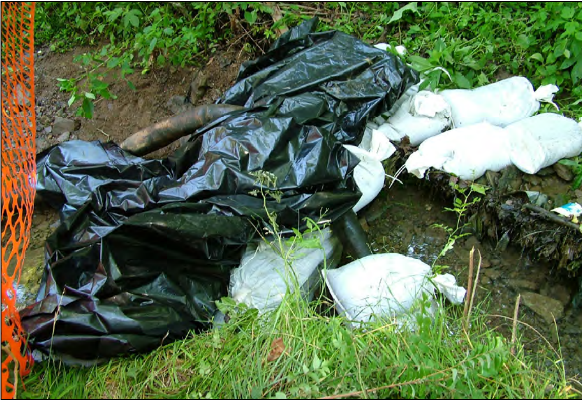
PHOTO 25: PARCEL 60 - PRE-EXCAVATION PREPARATIONS. DAMMING UPSTREAM WATERS FOR DIVERSION (FACING NORTH). JUNE 2006
