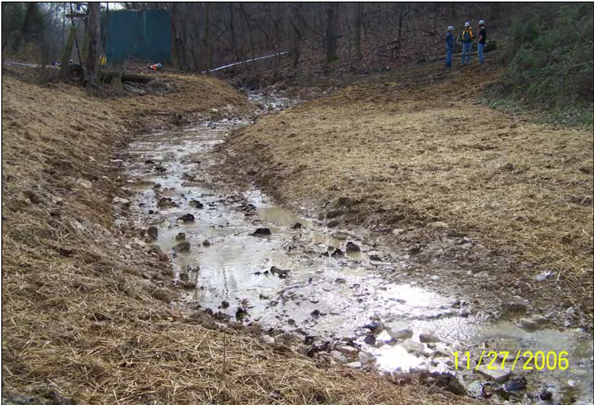
PHOTO 38: PARCEL 60 - RESTORED CREEK CHANNEL. STRAW IN PLACE FOR EROSION CONTROL (FACING EAST). NOVEMBER 2006
