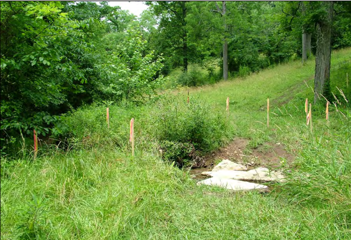
PHOTO 24: PARCEL 60 & 61 - PRE-EXCAVATION PREPARATIONS. STAKING THE EXCAVATION LIMIT (FACING NORTHWEST). JUNE 2006
