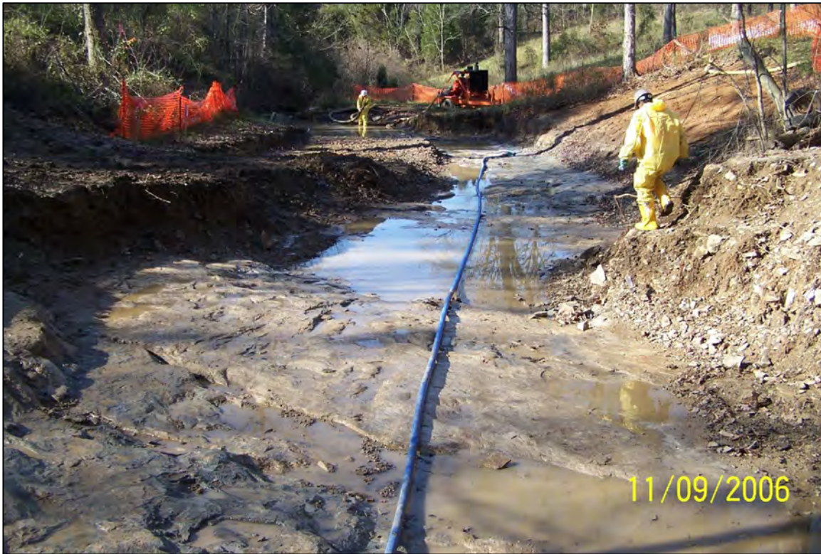
PHOTO 35: PARCEL 60 - LOOKING ALONG THE CLEAN CREEK EXCAVATION (FACING WEST). NOVEMBER 2006
