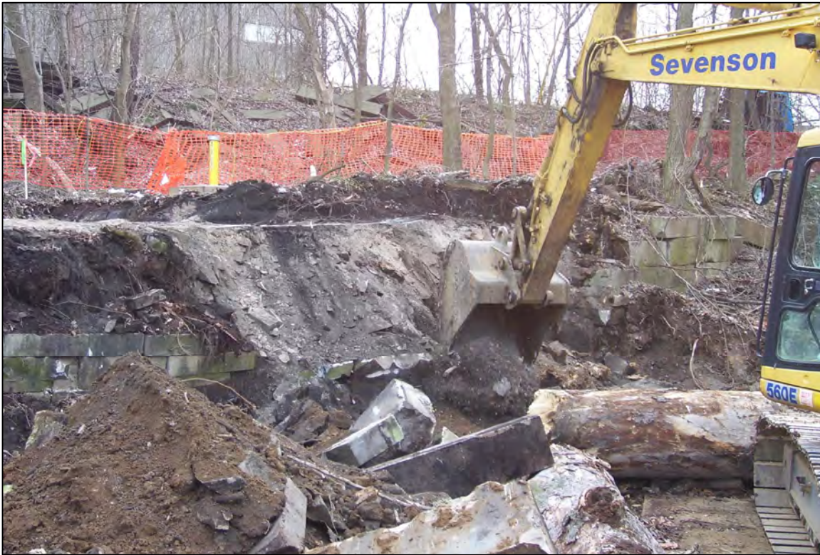
PHOTO 07: PARCEL 2 - RETAINING WALL EXCAVATION (FACING SOUTHEAST). FEBRUARY 2006
