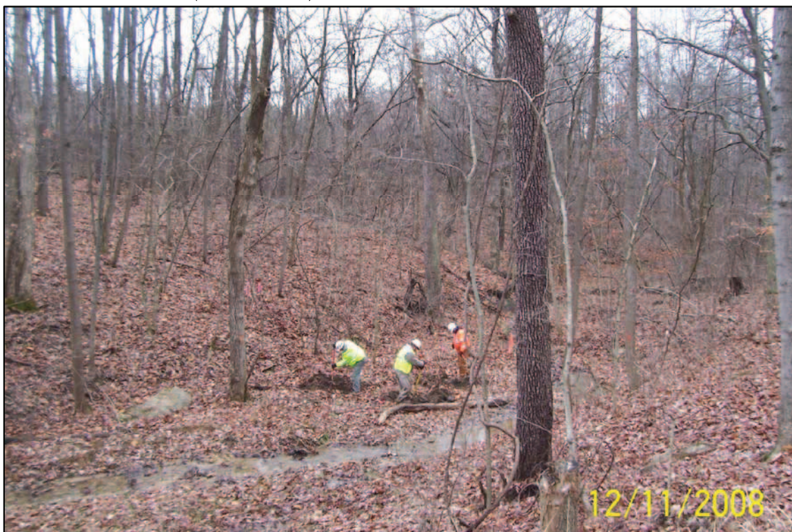
PHOTO 06: PARCEL 387/389 - PREPARING FOR INSTALLATION OF FOUR NEW TREES (FACING NORTH). DEC-08
