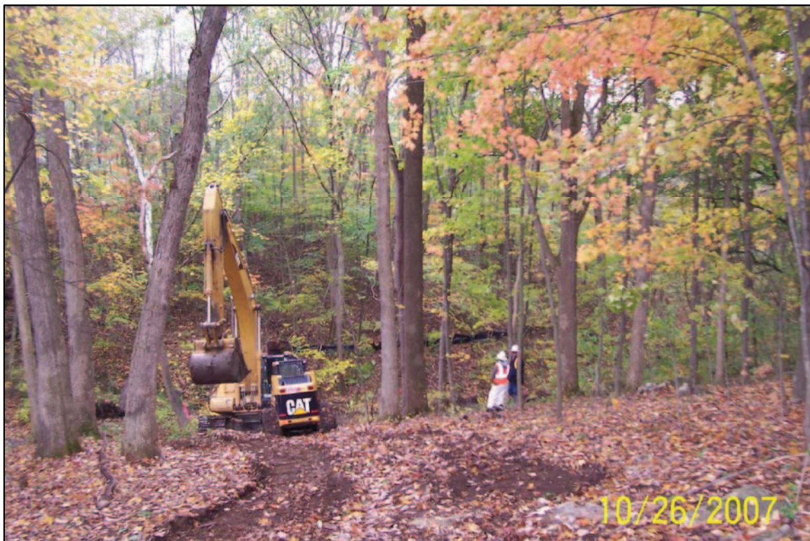
PHOTO 02: PARCEL 387/389 - CONTRACTOR PERFORMING EXCAVATION ACTIVITIES (FACING NORTH). OCT-07
