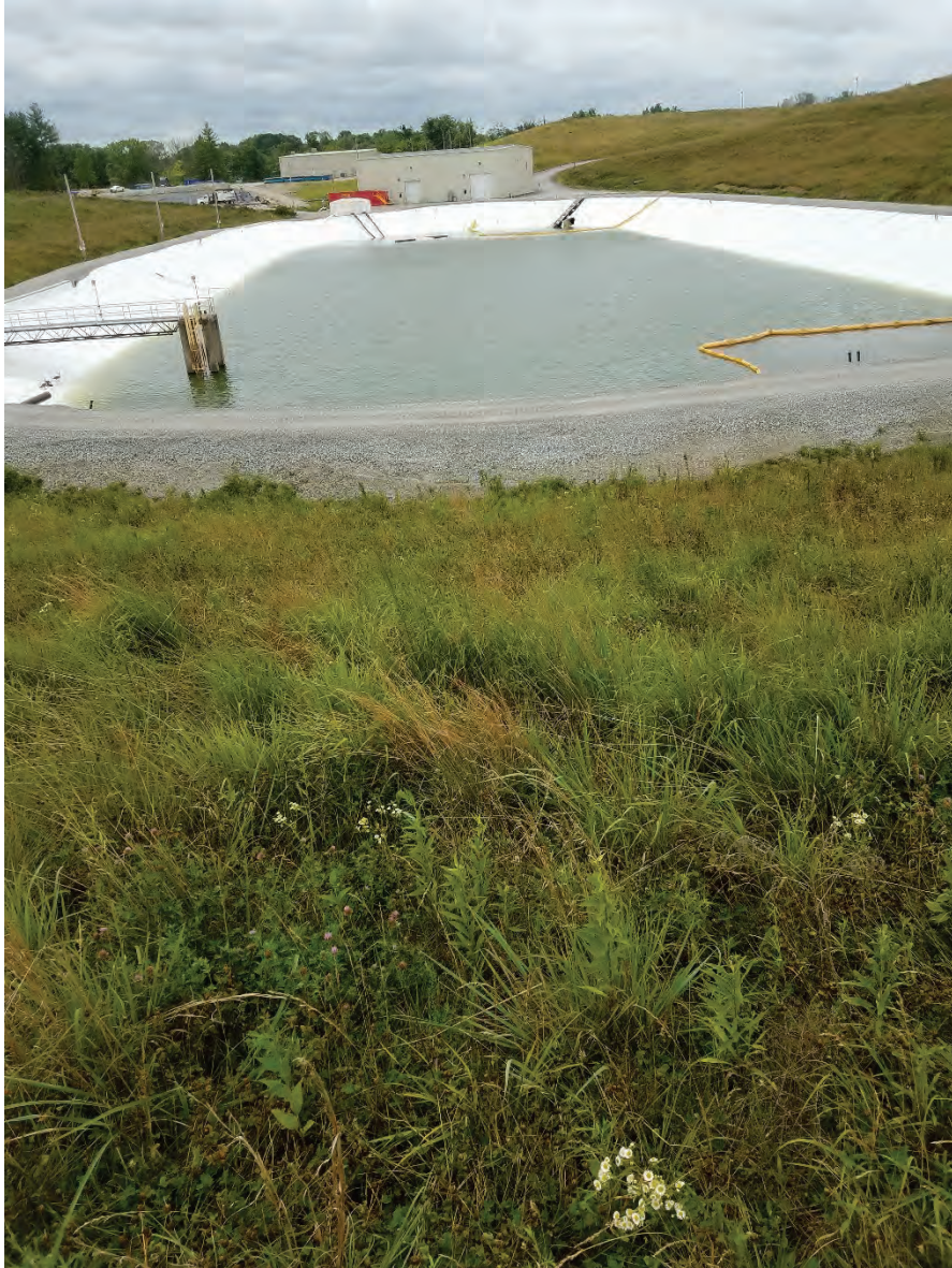
Photo 7: EV3 East Plant Area Cover facing south.
