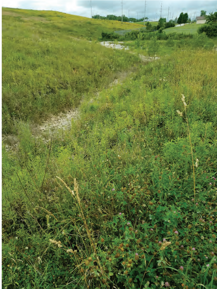
Photo 10: ES9 East Plant Cover System facing southwest
