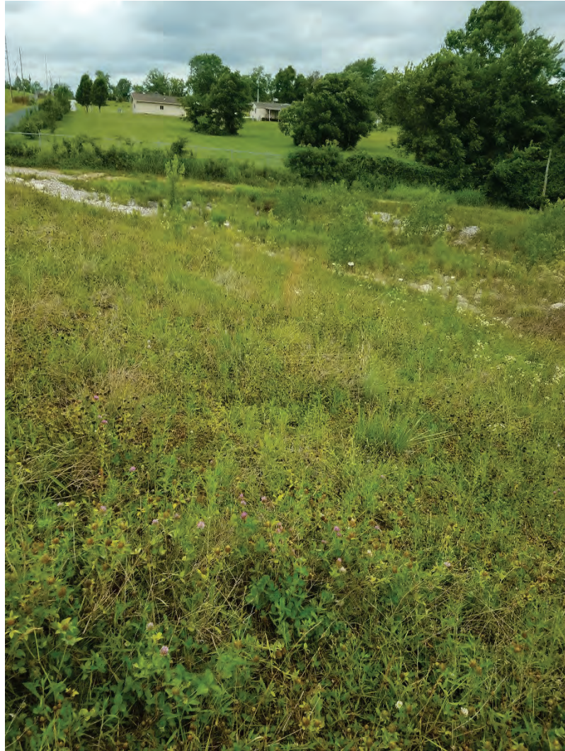
Photo 6: Drainage channel at ES6 East Plant Area Cover facing west.
