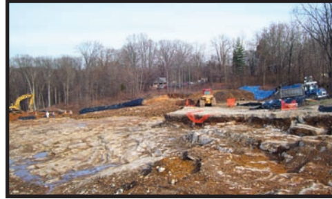
Excavation of Northern Tributary Parcels
