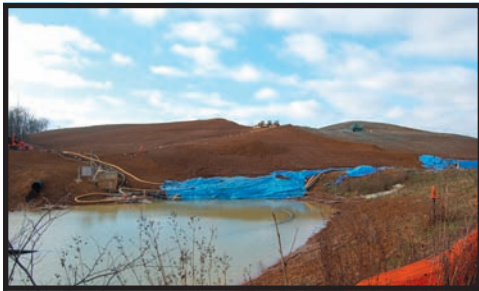
East Plant Area Grading Activities Near Bailey Scales Road
