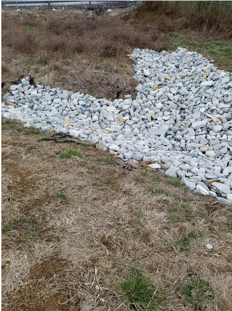
Photo 1: EV2 Drainage along ES6 facing west
