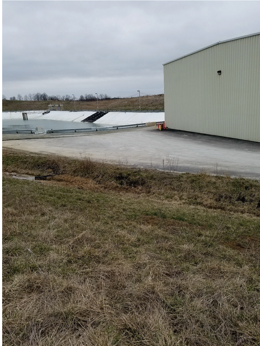
Photo 5: ES2 East Plant Area Cover facing north
