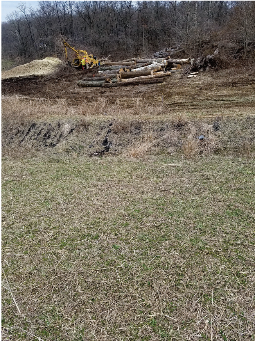
Photo 18: ES14 East Plant Area Cover facing east
