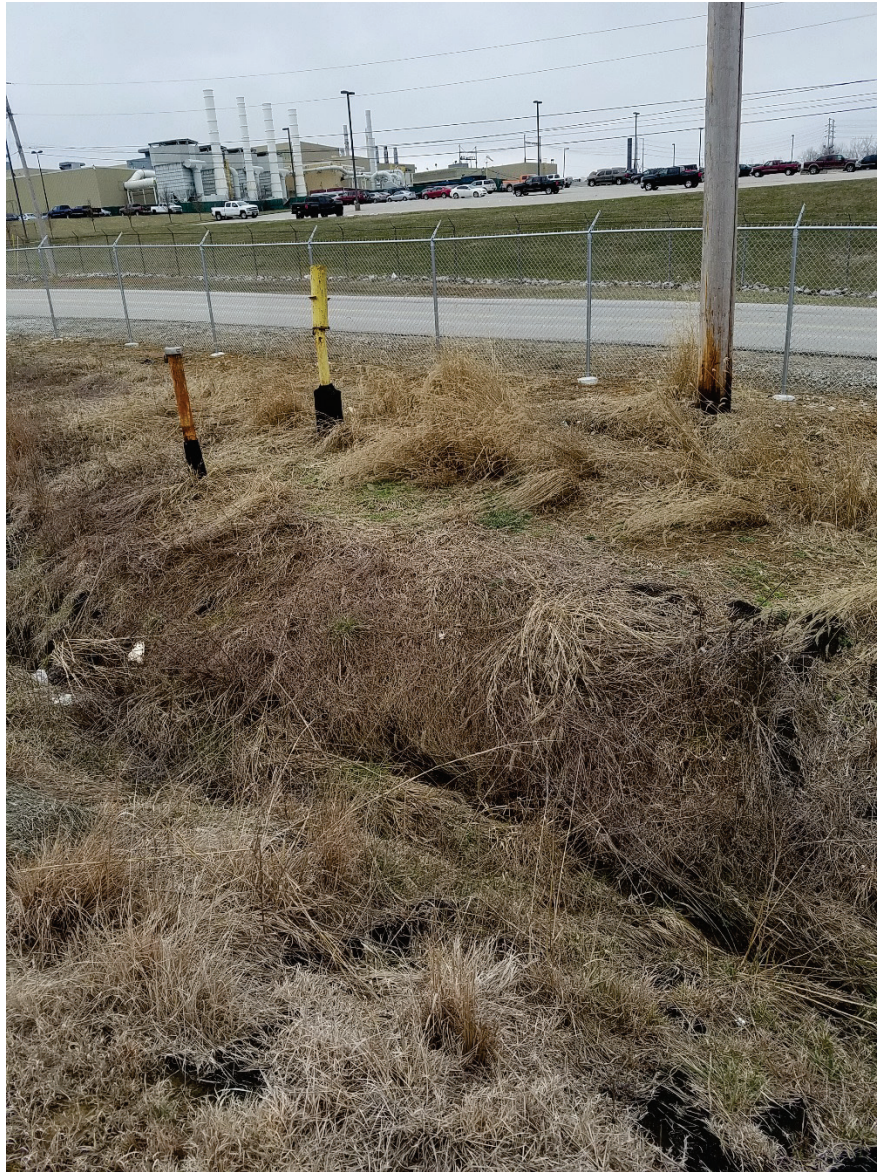
Photo 14: EV7 East Plant Cover facing southwest
