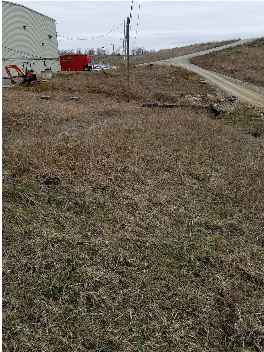
Photo 16: ES12 East Plant Area Cover facing north
