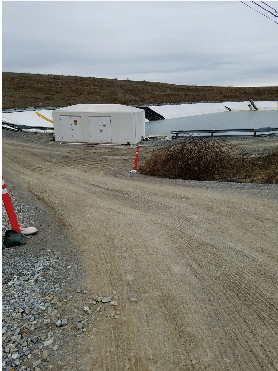
Photo 9: Stormwater pond facing northwest
