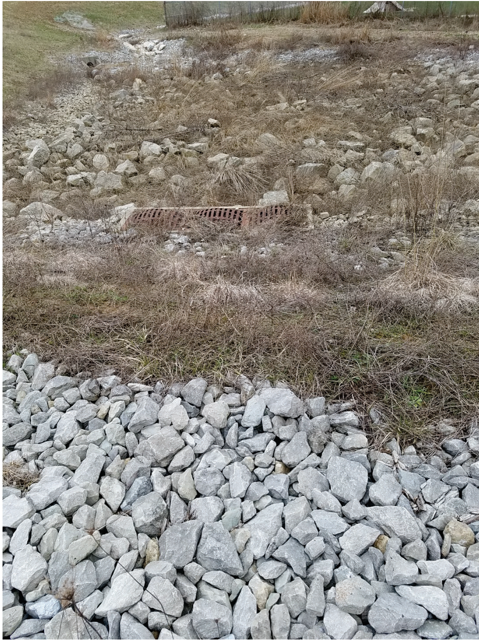
Photo 7: Drainage at ES6 facing west
