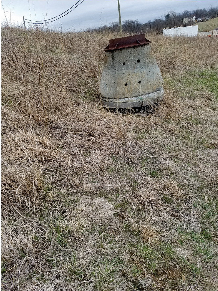
Photo 15: EV6 East Plant Area Cover area facing south
