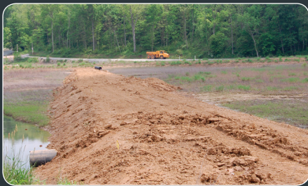
CLEAN CLAY BERM OVER THE NORTH LAWRENCE WATER AUTHORITY WATERLINE
