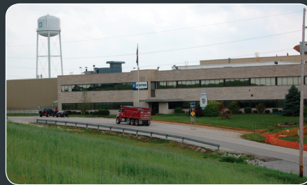
TRUCK TRAFFIC TO SUPPORT REMOVAL AND RESTORATION WORK
