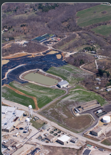
EAST PLANT AREA - APRIL 2011
