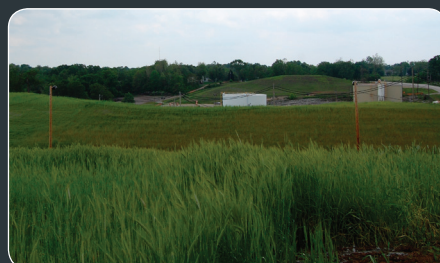
GRASS GROWTH ON COMPLETED AREAS OF THE COVER SYSTEM
