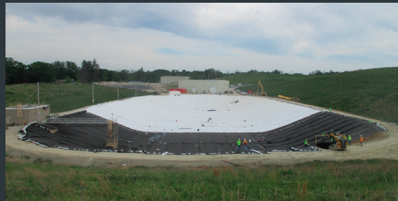
OVERVIEW OF STORMWATER MANAGEMENT FACILITY MAINTENANCE
