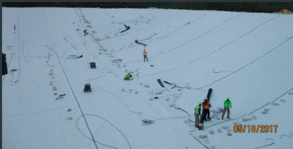
INSTALLATION OF HDPE LINER – STORMWATER MANAGEMENT FACILITY
