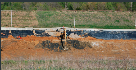
DRY DREDGING OF THE STORMWATER MANAGEMENT FACILITY
