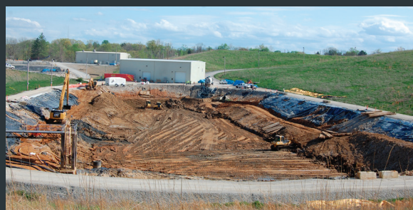
REMOVAL OF IMPACTED MATERIAL – STORMWATER MANAGEMENT FACILITY
