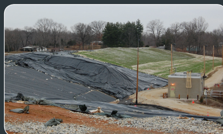
EAST PLANT AREA TEMPORARY LINER AND COMPLETED COVER
