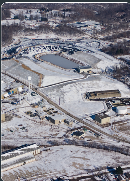
EAST PLANT AREA - DECEMBER 2010
