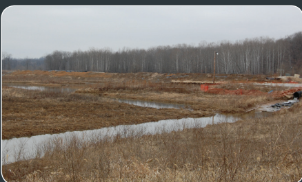
REMAINING REMOVAL SITE - AREA 'G'
