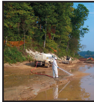
Creek Bed Power Washing
