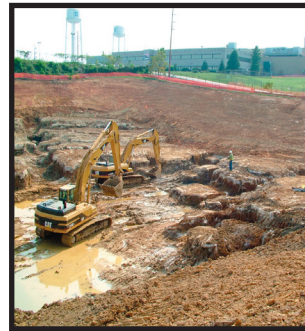
East Plant Vault Excavation
