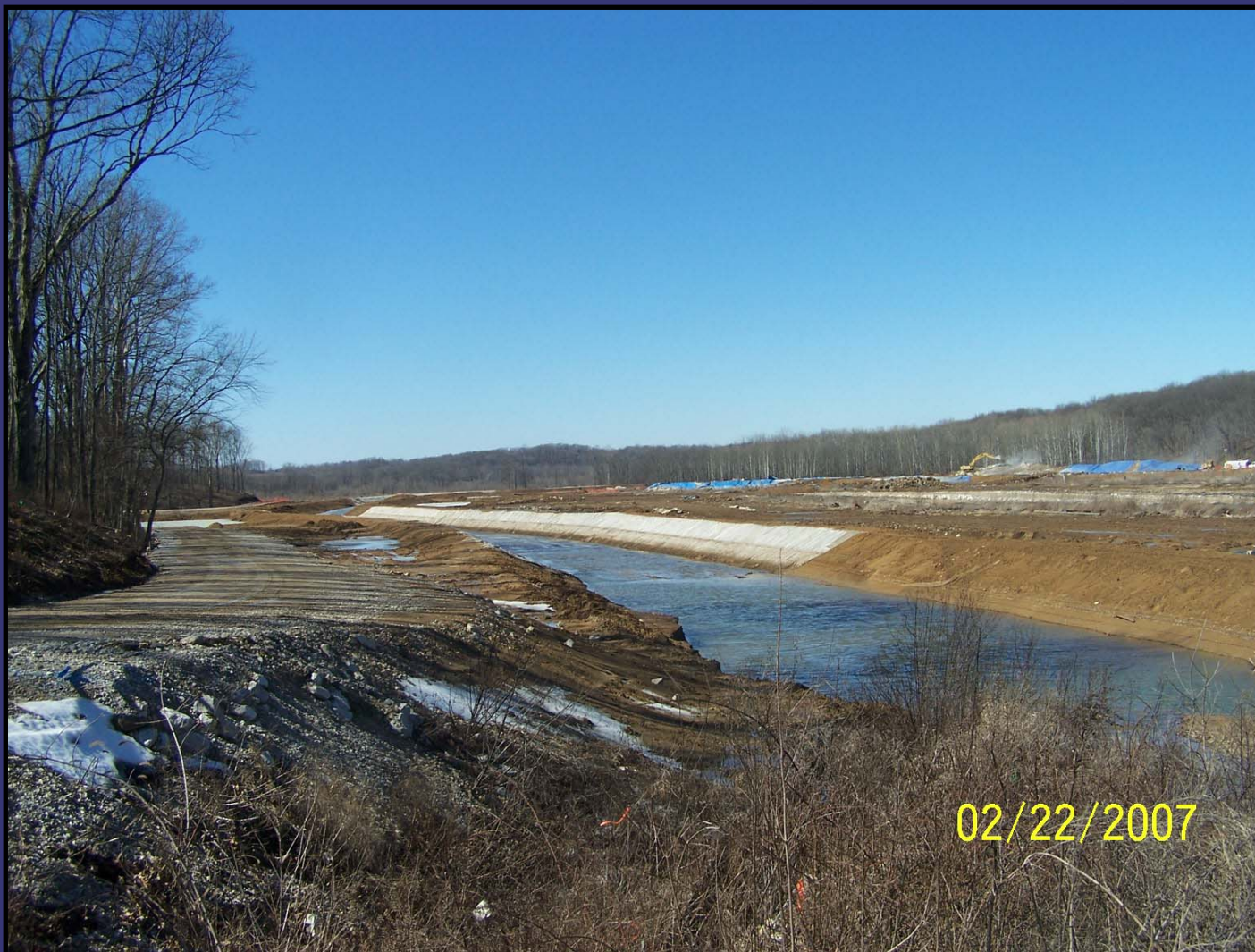
Diversion Channel No. 3
