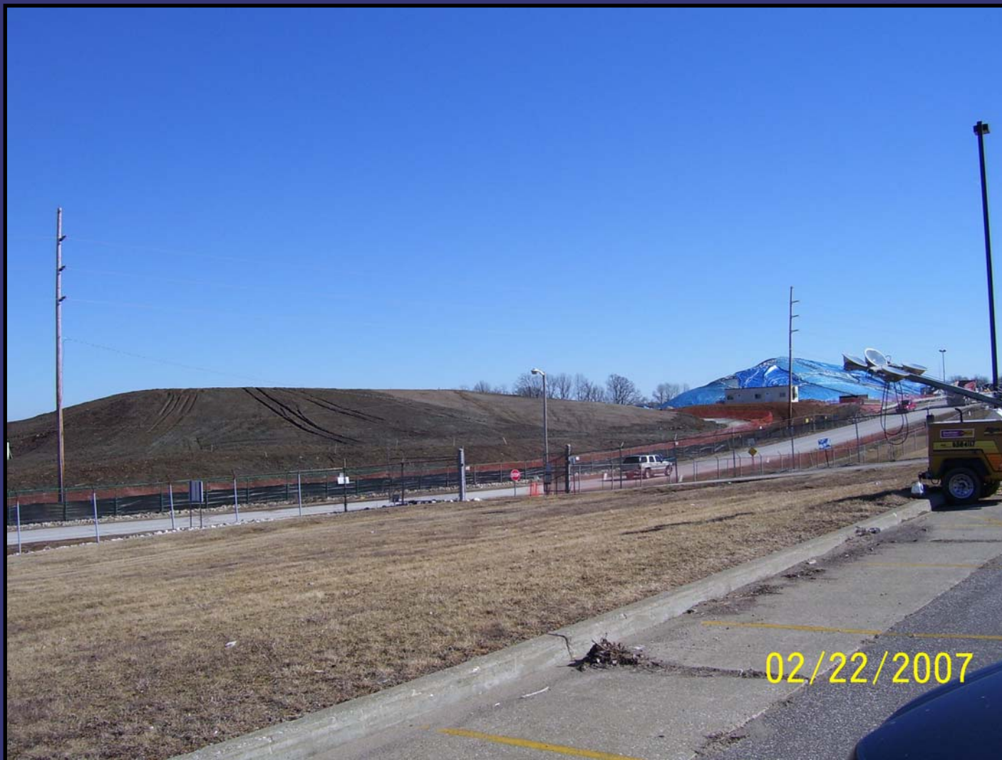
East Plant Area Vault
