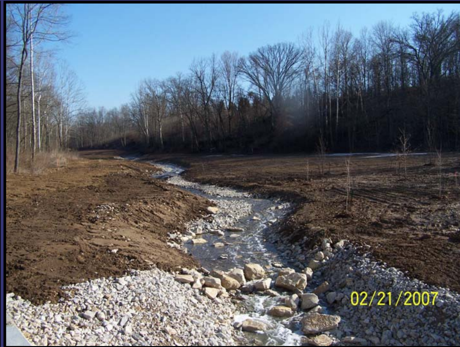
Property south of Broomsage Road
