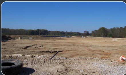
SOIL STOCKPILE REMOVAL COMPLETED ON PEERLESS ROAD.
