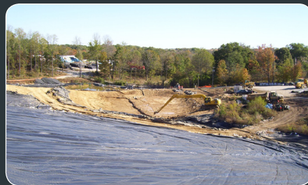
CLEANING OUT THE DETENTION BASINS WEST OF BAILY SCALES ROAD.
