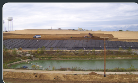
BACKFILLING OVER COMPLETED LINER IN THE EAST PLANT AREA.
