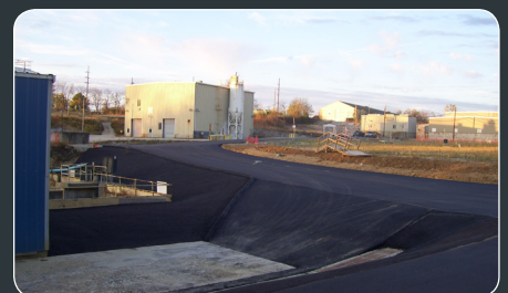
ASPHALT COVER COMPLETED NEAR THE WATER TREATMENT PLANT.
