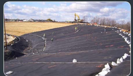
LINER INSTALLATION NORTH OF THE STORMWATER POND.
