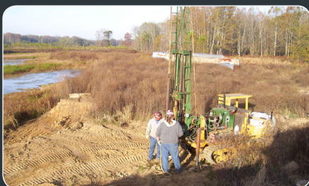
INSTALLING BOREHOLES NEAR THE FORMER STOCKPILE OFF OF PEERLESS ROAD.
