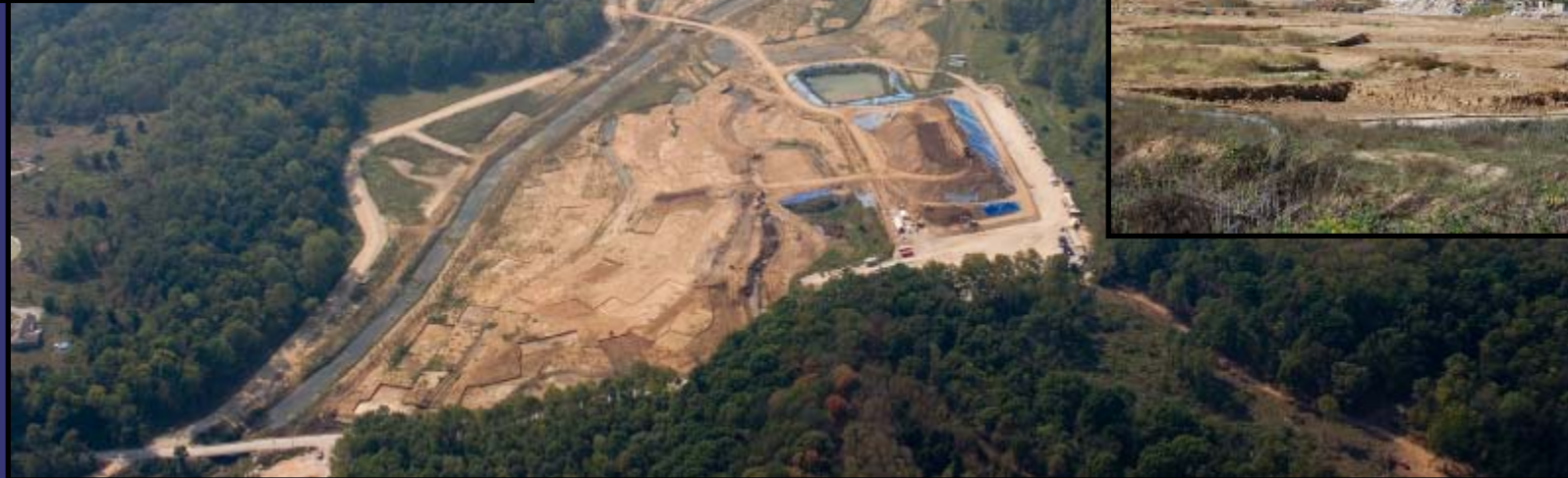
Excavation west of Peerless Road
