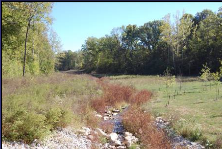
Property south of Broomsage Road restoration
