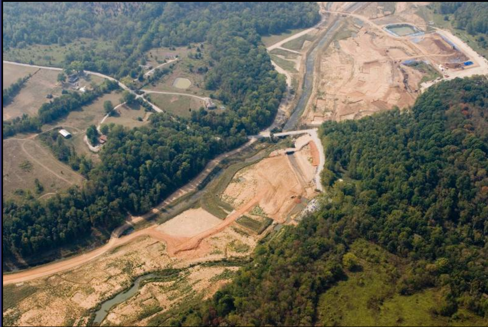
Excavation east and west of Peerless Road
