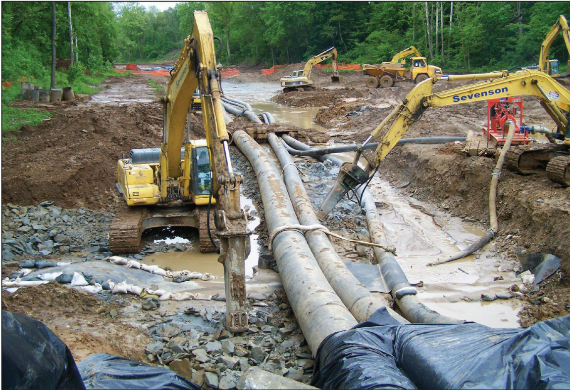
PHOTO No. 19, PARCEL 22: ROCK BREAKING ACTIVITIES SOUTH OF THE CULVERT. (MAY 2006)
