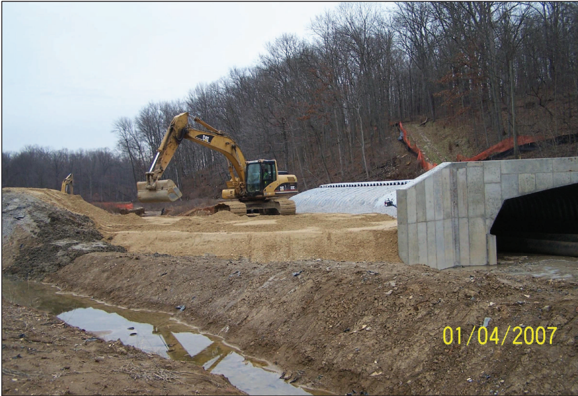
PHOTO No. 25, PARCEL 22: BACKFILLING AGAINST THE CULVERT TO GRADE. (JAN. 2007)
