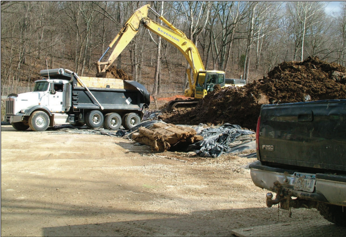
PHOTO No. 10, PARCEL 22: LOADING HAUL TRUCK WITH LESS THAN 50 MG/KG PCB SOIL MATERIAL DESTINED FOR THE EAST PLANT AREA. (JAN. 2006)
