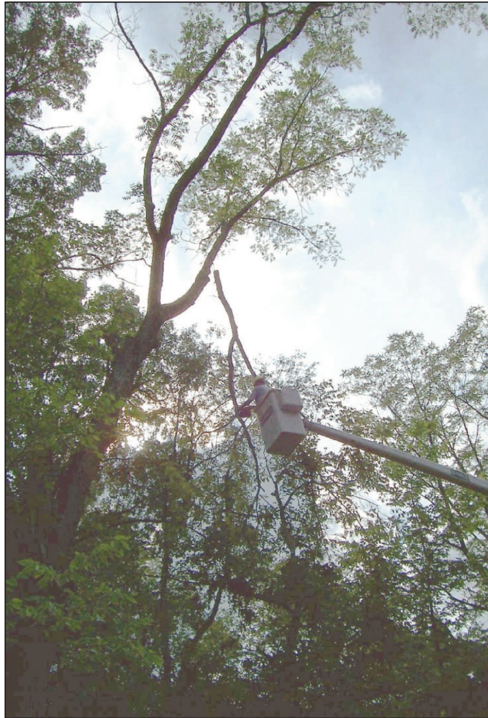
PHOTO No. 6, PARCEL 22: TREE CUTTING OVER THE HOUSE ON PARCEL 22. (AUG. 2004)
