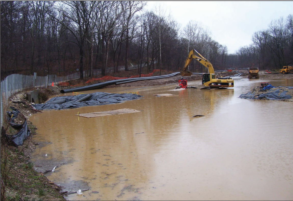
PHOTO No. 15, PARCEL 22: EXCAVATION DURING HEAVY RAIN EVENT. (MAR. 2006)
