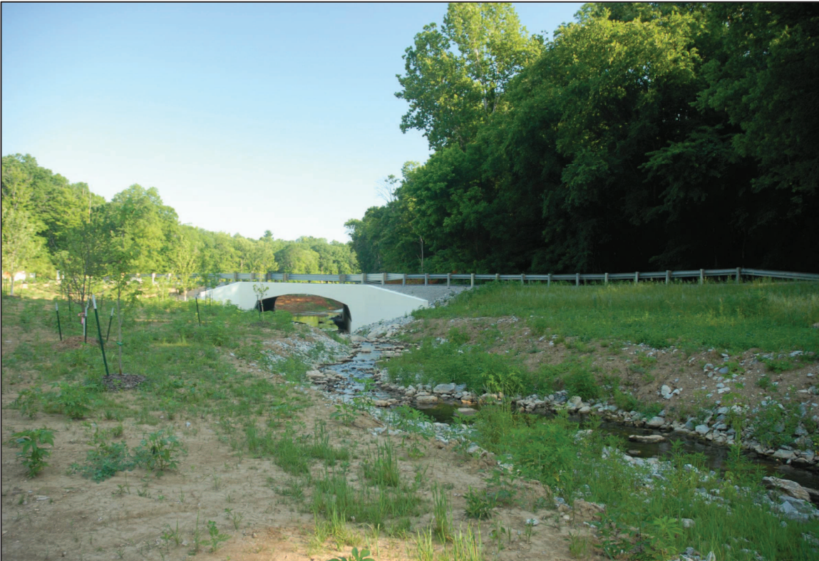
PHOTO No. 28, PARCEL 22: RESTORED CREEK CHANNEL AND STREAM BANKS FACING THE NEW BROOMSAGE ROAD CULVERT. (JUN. 2007)
