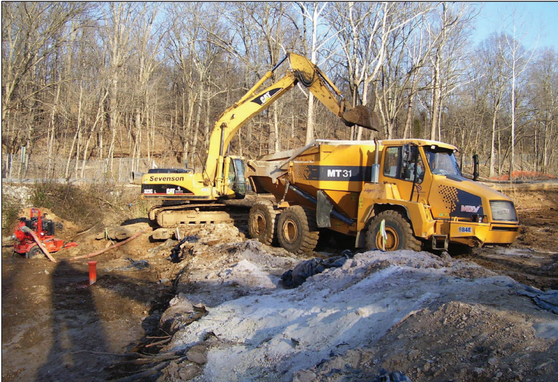
PHOTO No. 13, PARCEL 22: EXCAVATION NEAR THE BROOMSAGE ROAD CULVERT. (FEB. 2006)
