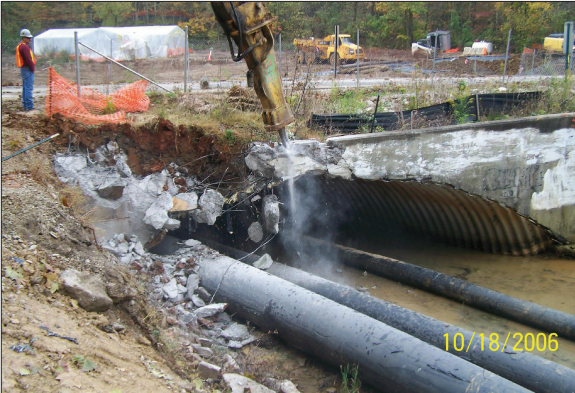
PHOTO No. 20, PARCEL 22: REMOVAL OF THE BROOMSAGE ROAD CULVERT HEADWALL. (OCT. 2006)
