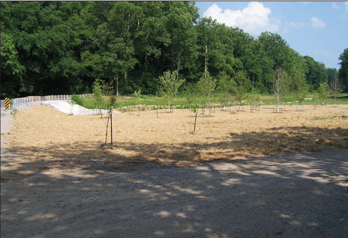
PHOTO No. 29, PARCEL 22: STRAW USED FOR EROSION CONTROL AFTER SEEDING LAWN. (JUN. 2007)
