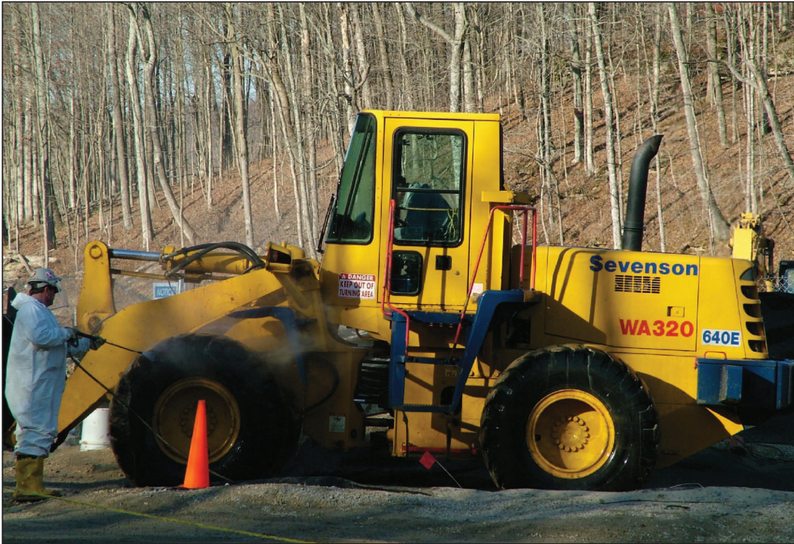
PHOTO No. 9, PARCEL 22: DECONTAMINATION OF FRONT-END LOADER WHEELS. (JAN. 2006)
