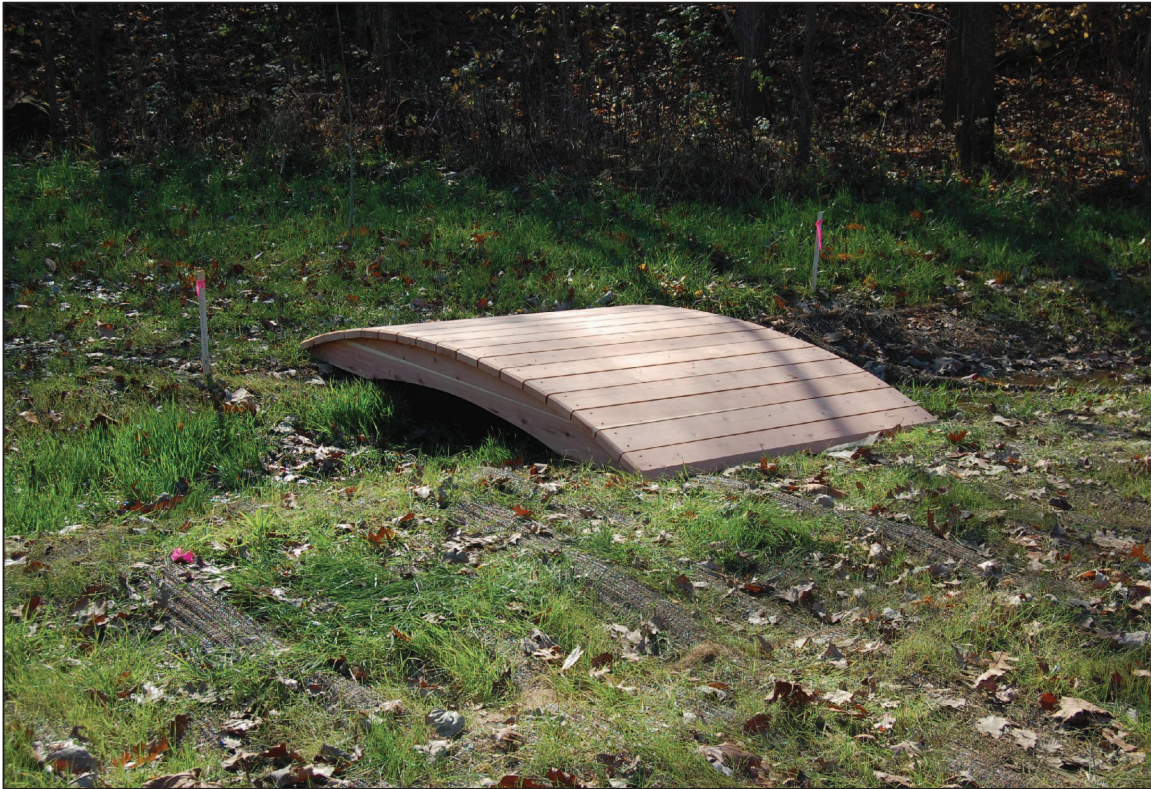
PHOTO No. 34, PARCEL 22: FOOT BRIDGE OVER SWALE. (NOV. 2009)
