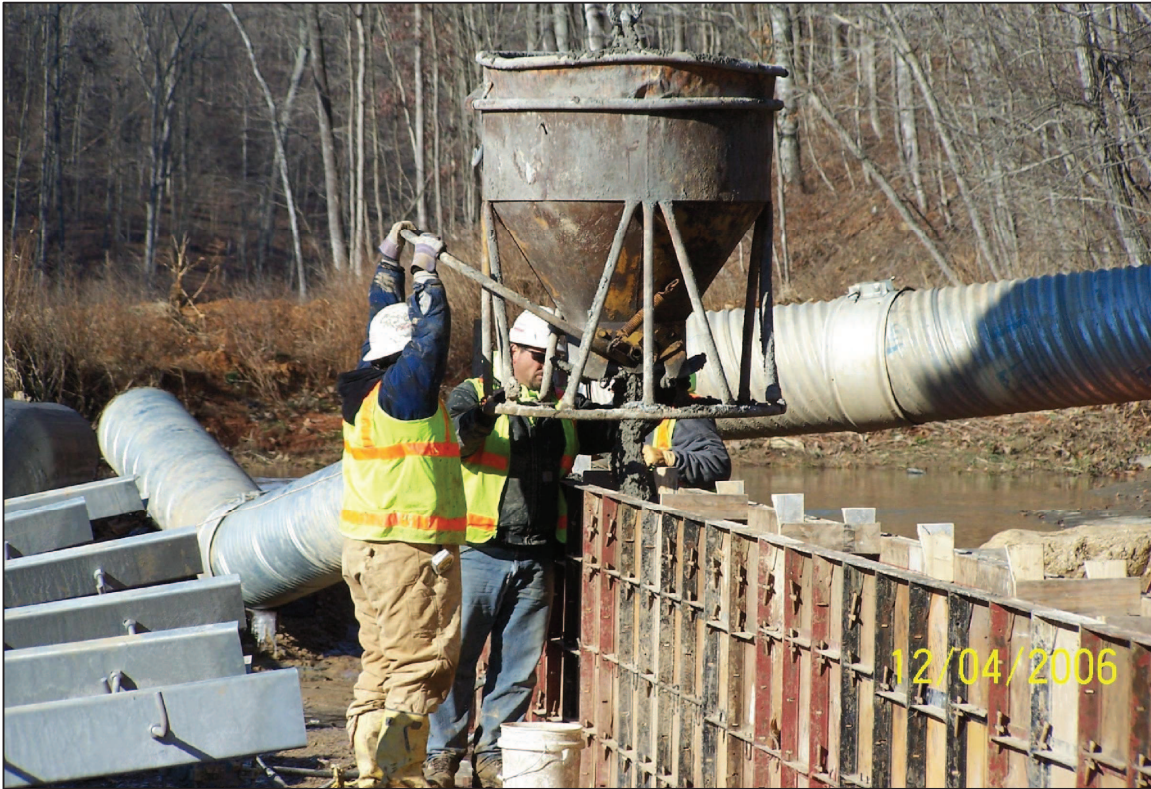
PHOTO No. 23, PARCEL 22: POURING CONCRETE FOR THE STEM WALLS. (DEC. 2006)
