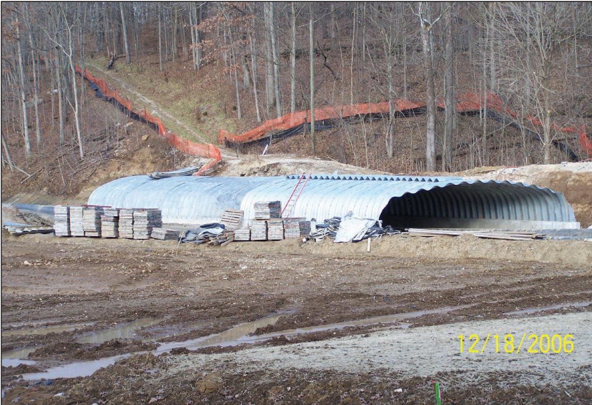
PHOTO No. 24, PARCEL 22: OVERLOOKING THE ASSEMBLED CULVERT PRIOR TO BACKFILLING. (DEC. 2006)
