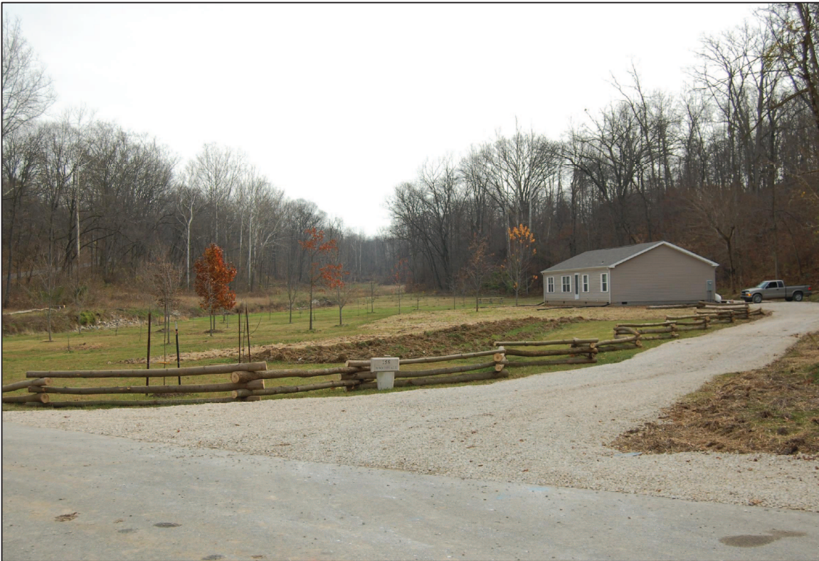
PHOTO No. 35, PARCEL 22: COMPLETED RESTORATION INCLUDING NEW HOUSE, SEPTIC, FENCE, AND RESEDED LAWN. (NOV. 2009)
