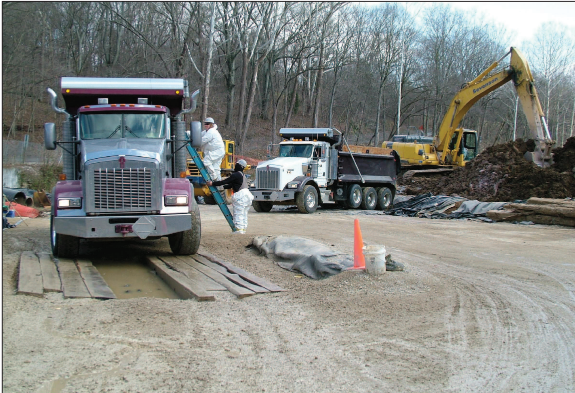
PHOTO No. 12, PARCEL 22: TRUCK PREPARATION OF TARPS PRIOR TO ENTERING PUBLIC ROADS. (JAN. 2006)
