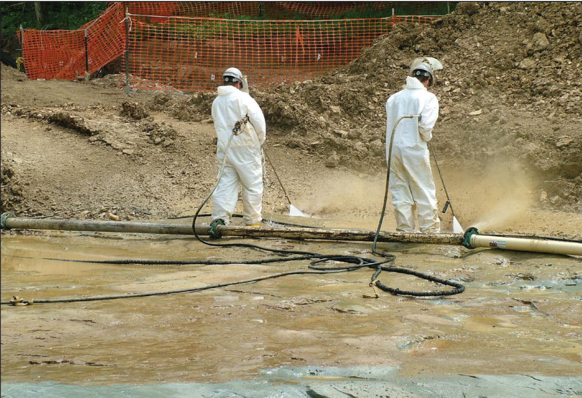
PHOTO No. 18, PARCEL 22: POWERWASHING THE BEDROCK SURFACE. (MAY 2006)
