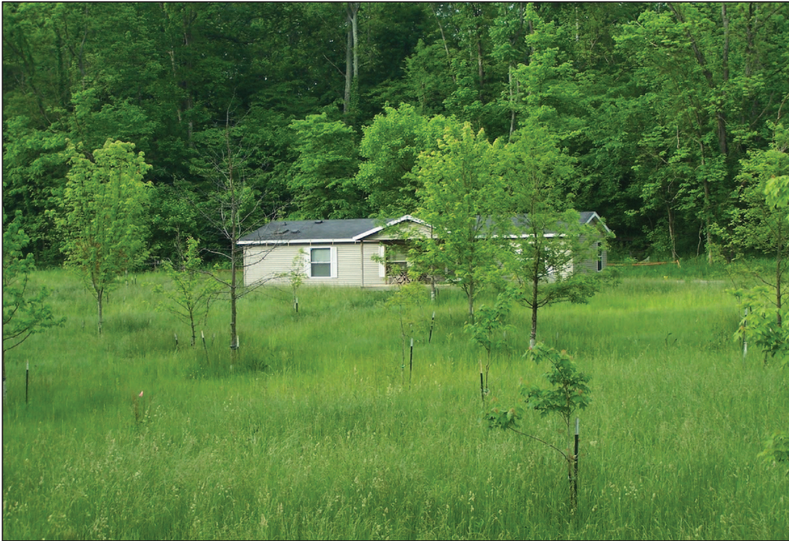
PHOTO No. 30, PARCEL 22: RESTORED PARCEL 22 LAWN AREA LOOKING WEST. (APR. 2008)
