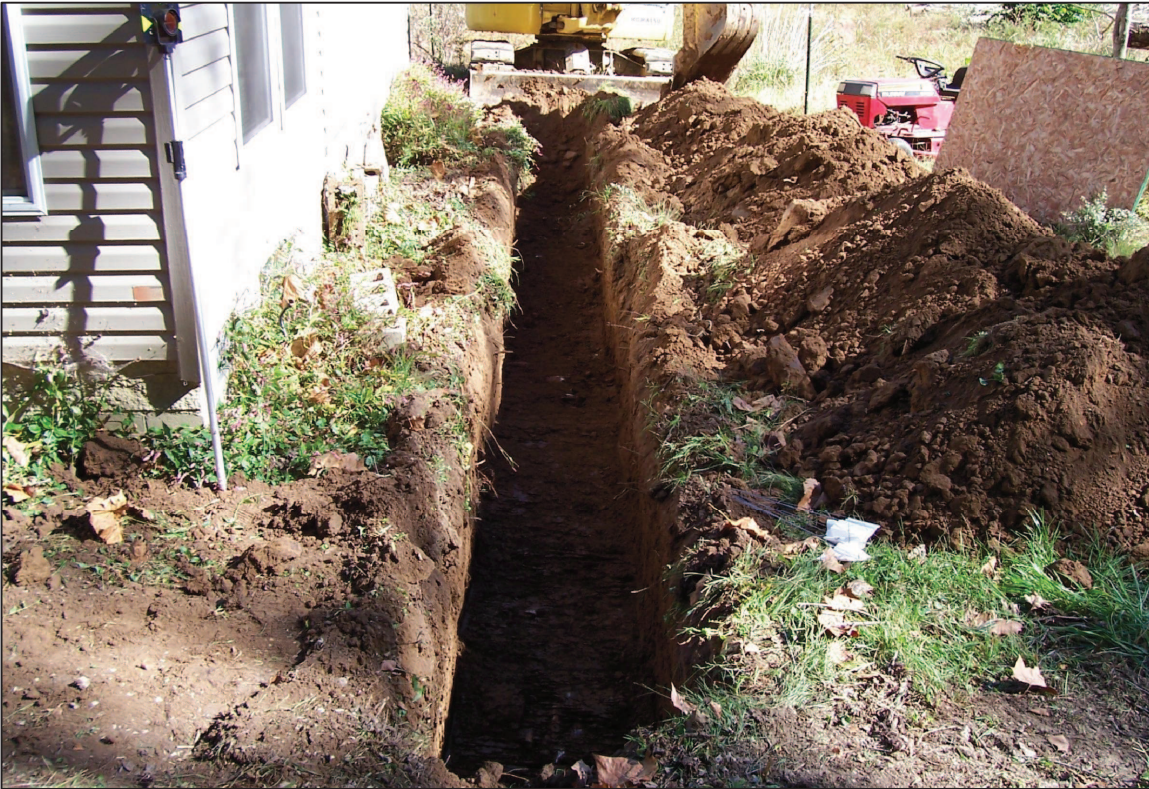
PHOTO No. 7, PARCEL 22: DELINEATION SAMPLING NEXT TO THE HOUSE FOUNDATION. (OCT. 2004)
