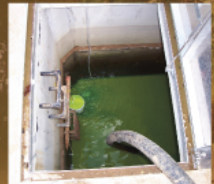
Site Source Control collection system where most dye was detected. Dye visible in this photo.
