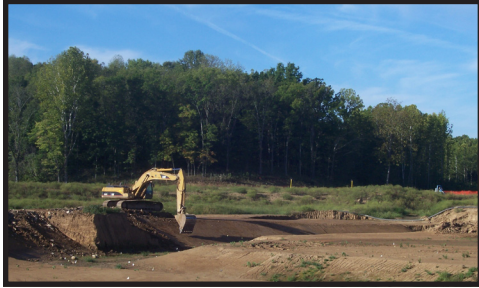
Excavation Progress West of Peerless Road
