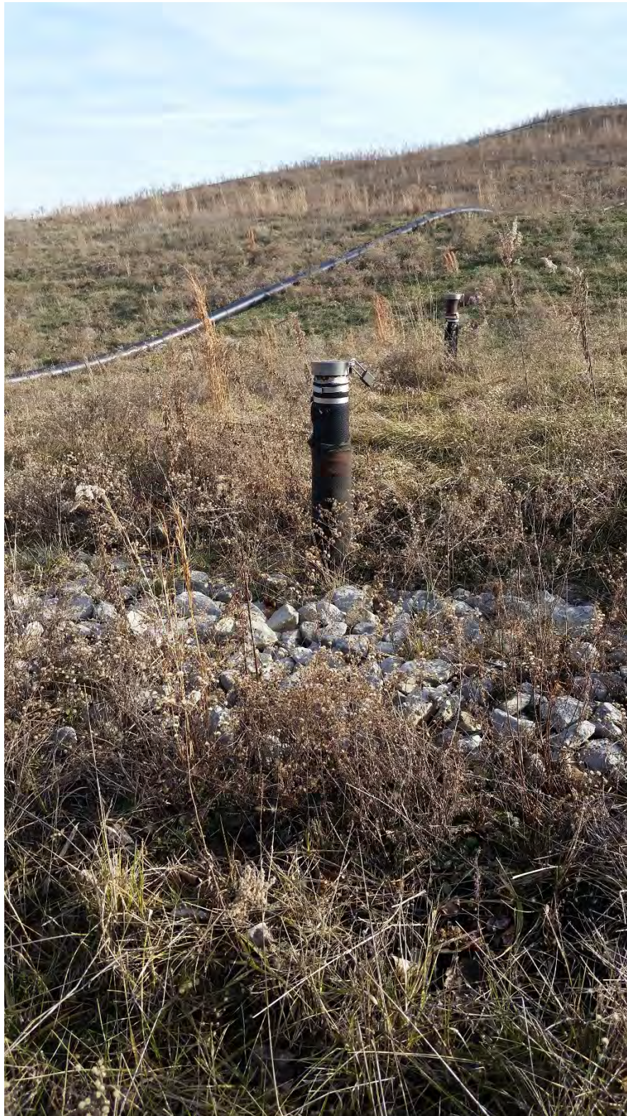
Photo 8: EV3 East Plant Area Cover facing north (CH-29D)
