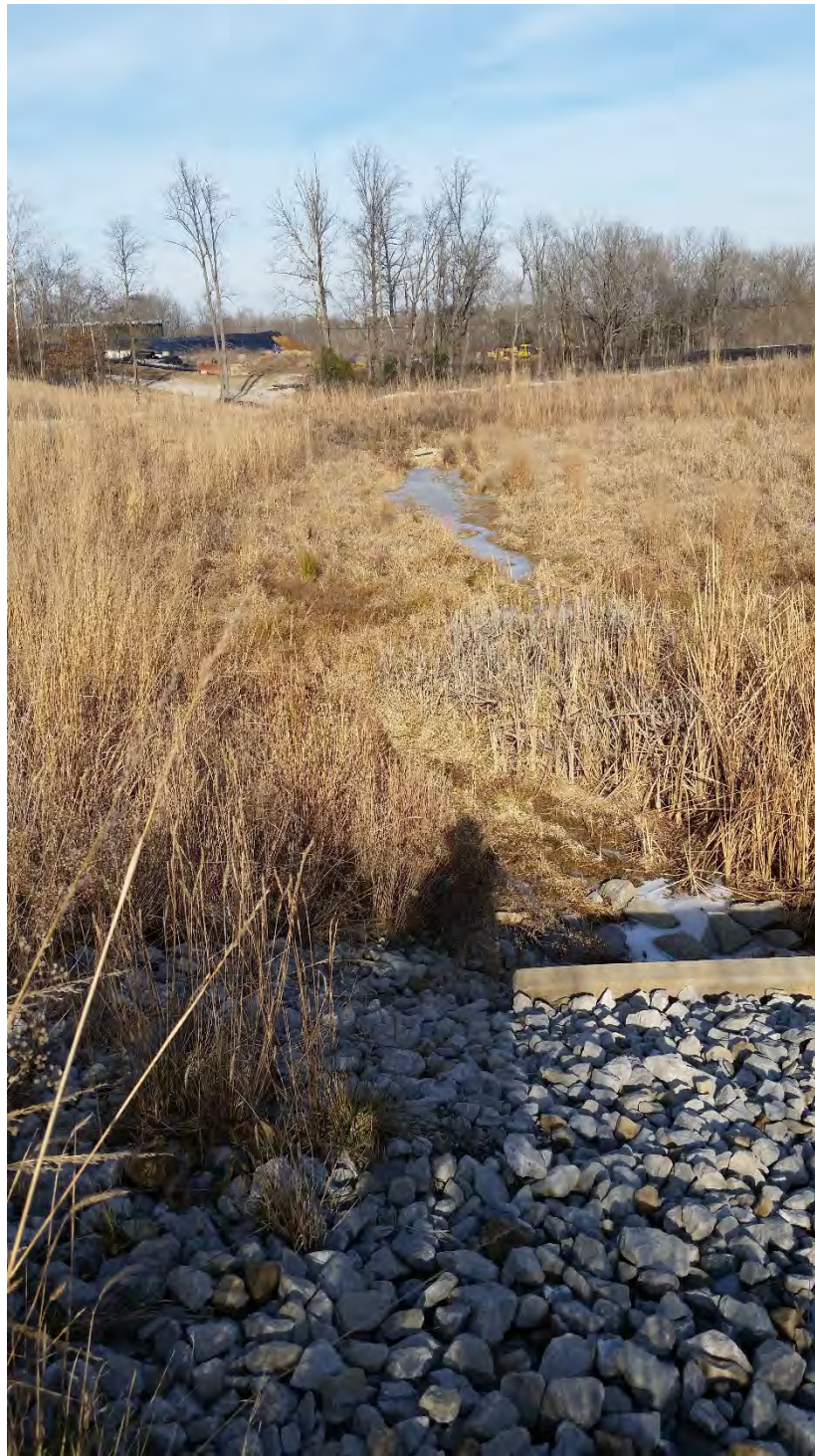
Photo 13: Looking north along ES11 East Plant Area Cover
