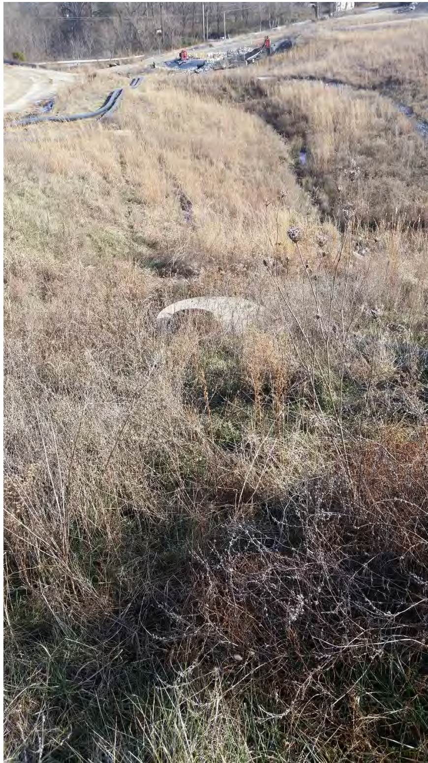
Photo 11: ES9 East Plant Cover System facing east through detention basins
