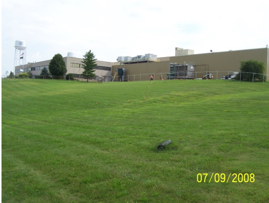
Photo No. 30: AOI 21-2 – Pre-construction conditions, facing southwest. July 2008
