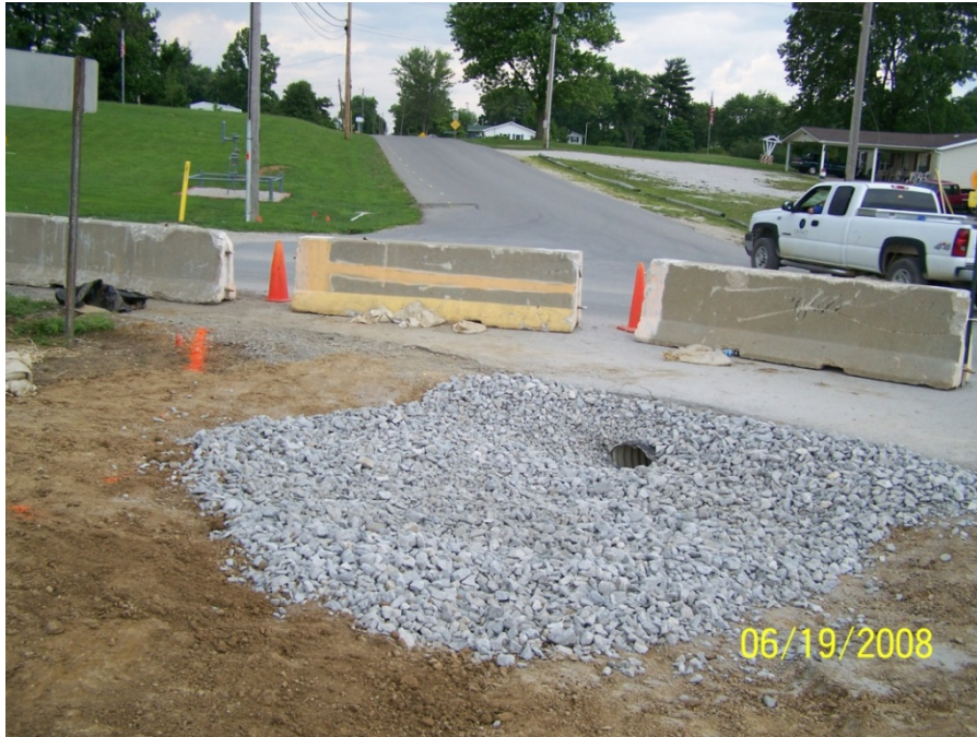
Photo No. 7: MH-ST-43 – Placement of stone around culvert, facing north. June 2008.
