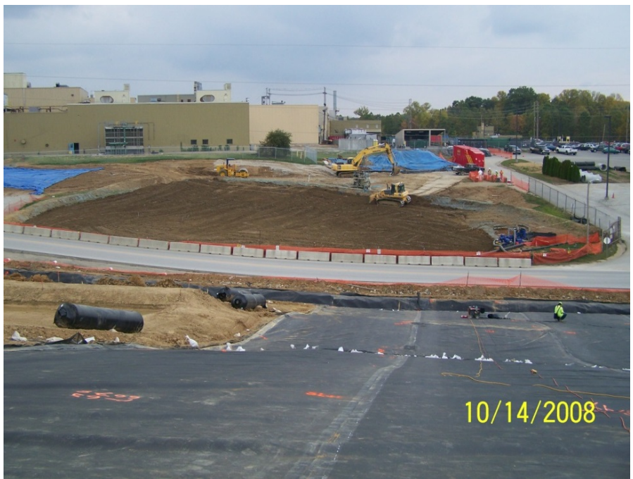
Photo No. 41: AOI 21-2 - Backfilling with <50 mg/kg PCBs material, facing west. October 2008.
