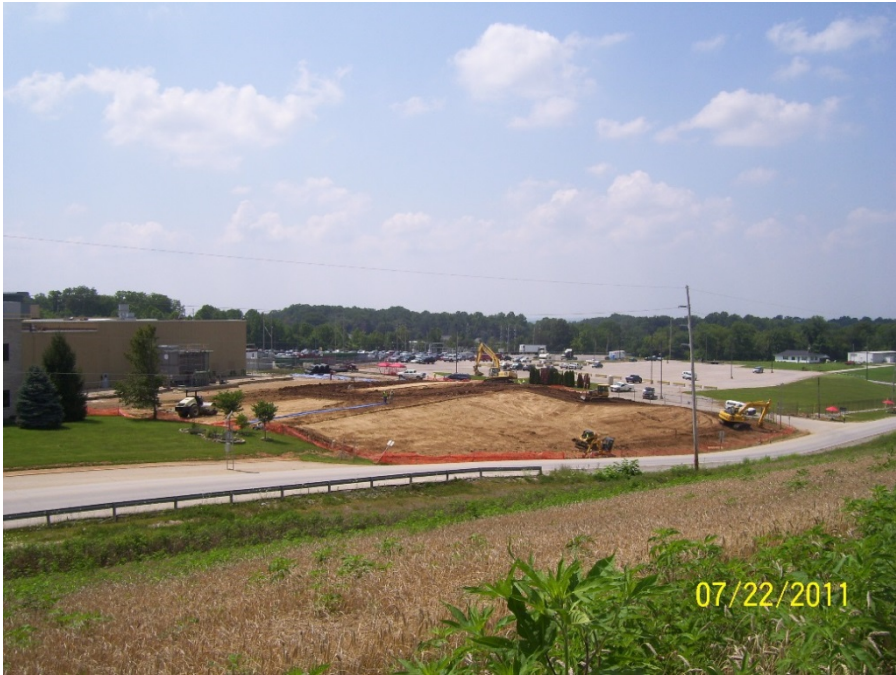
Photo No. 51: AOI 21-2 – Installation of clay barrier layer, facing northwest. July 2011.
