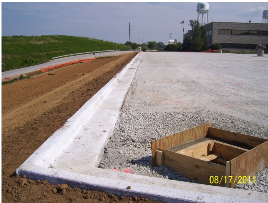
Photo No. 59: AOI 21-2 – Parking lot curbing, facing south. August 2011.
