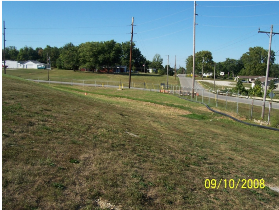
Photo No. 13: MH-ST-43 – Restored embankment, facing north. September 2008.
