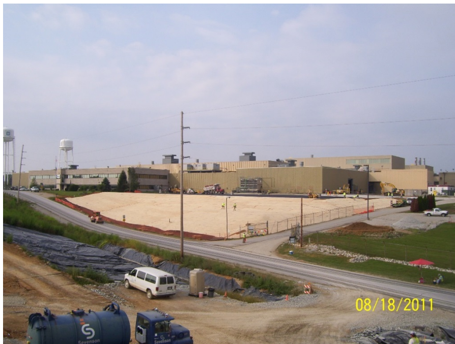
Photo No. 61: Installation of seeding and erosion control, facing southwest. August 2011.
