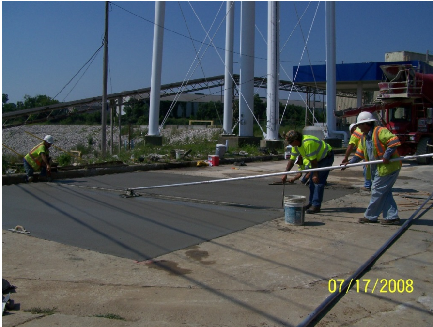
Photo No. 22: AOI 18 – Installation of expansion joint, facing southwest. July 2008.
