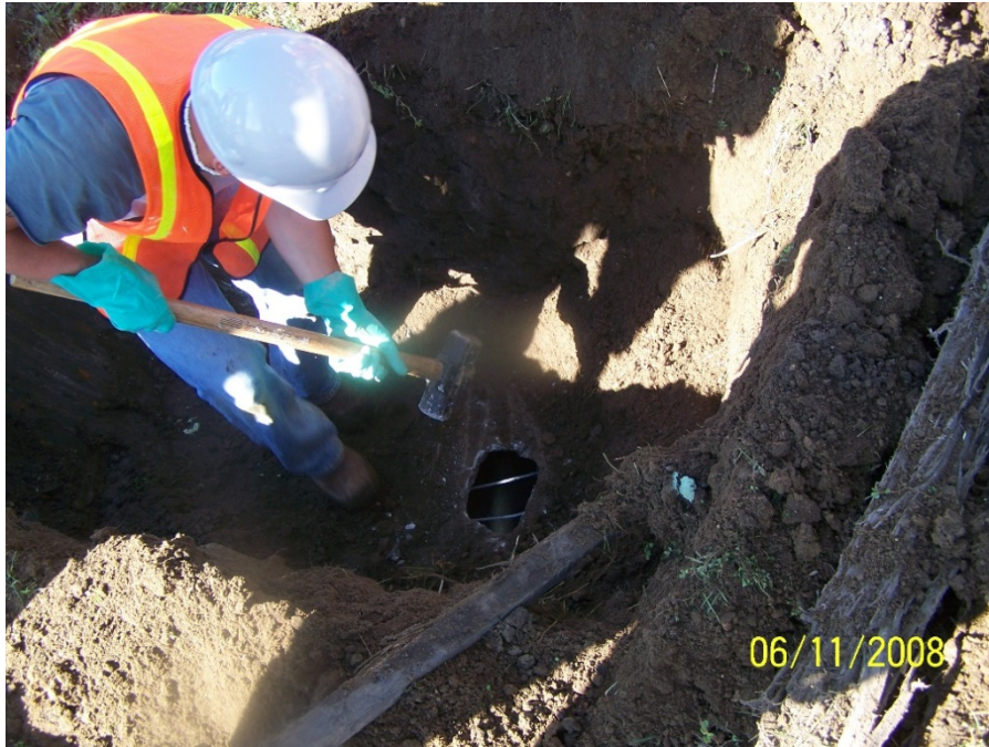
Photo No. 5: MH-ST-43 – Viewing port, facing down. June 2008.
