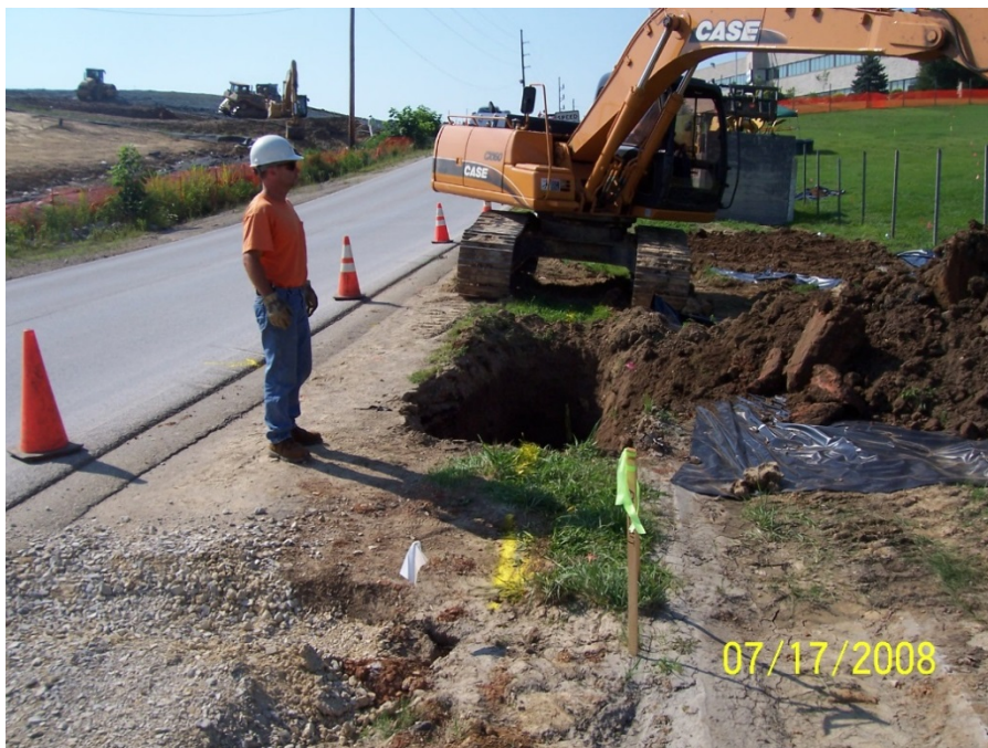
Photo No. 31: AOI 21-2 – Vectren gas line locating, facing south. July 2008.
