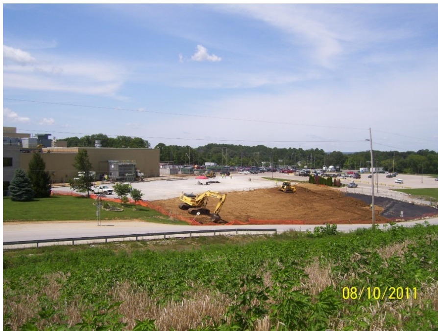
Photo No. 57: Placement of common fill material, facing northwest. August 2011.
