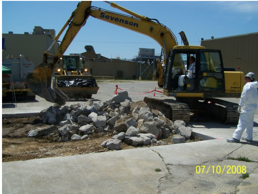
Photo No. 16: AOI 18 – Removal of concrete slab, facing west. July 2008.
