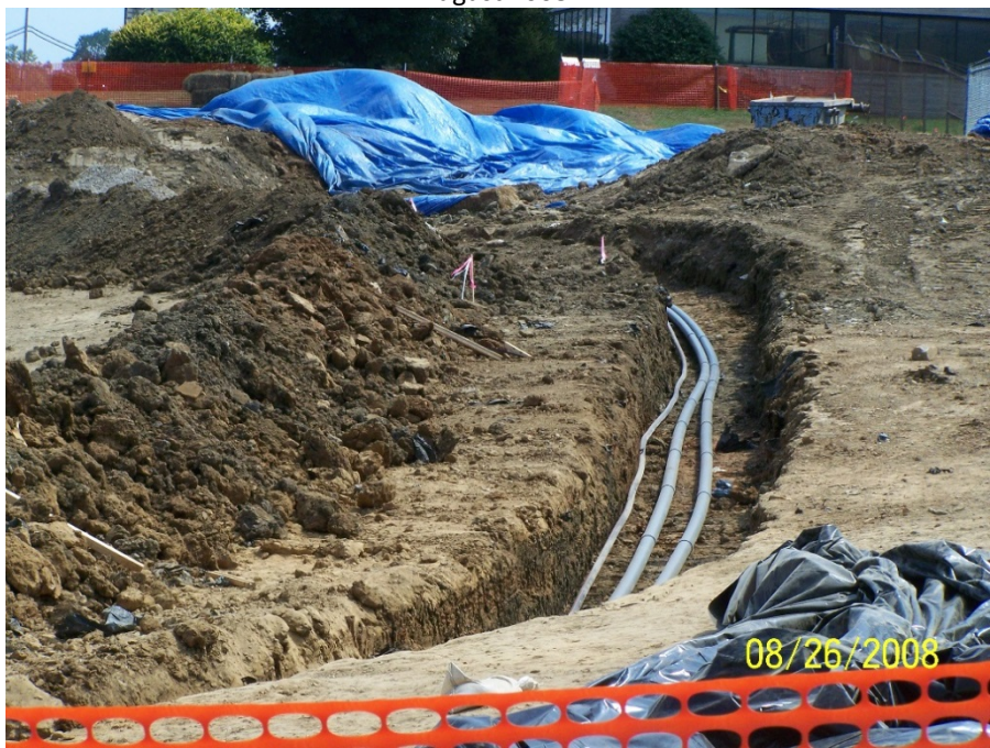
Photo No. 37: AOI 21-2 – Installation of AT&T cable conduit, facing south. August 2008.
