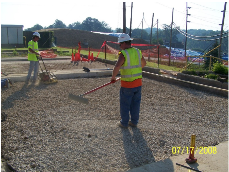
Photo No. 19: AOI 18 – Backfilling with clean stone, facing southeast. July 2008.
