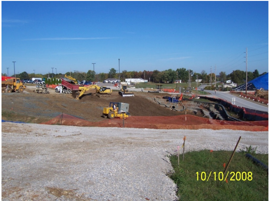
Photo No. 40: AOI 21-2 – Backfilling with < 50 mg/kg PCBs material, facing north. October 2008.
