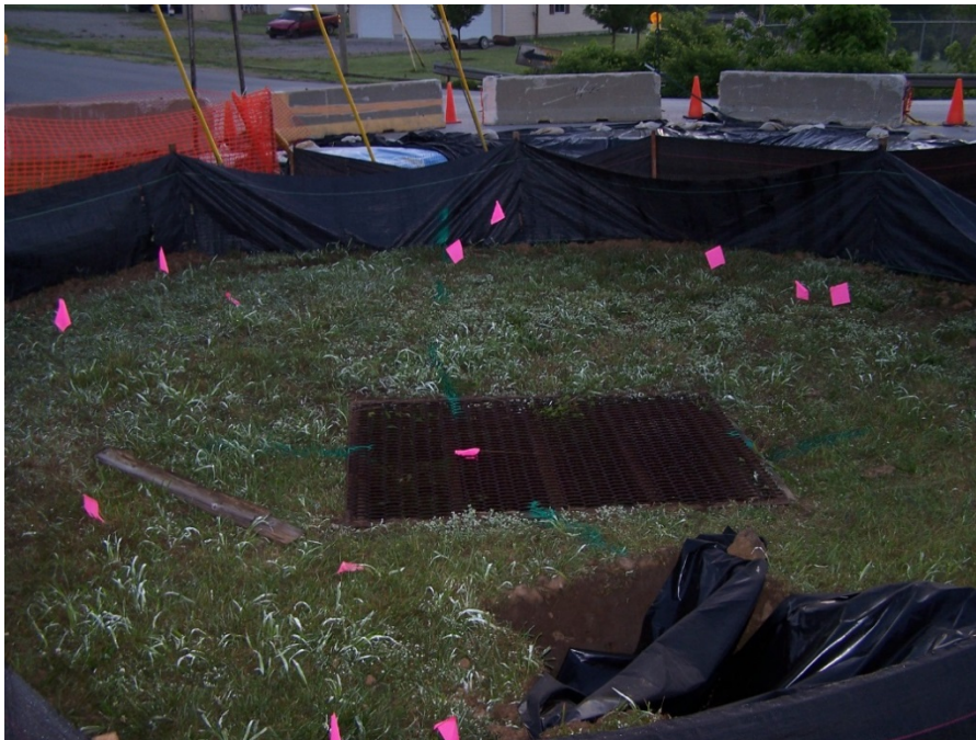
Photo No. 2: MH-ST-43 – Pre-excavation, facing northeast. May 2008.
