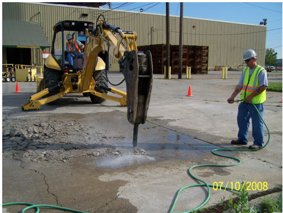
Photo No. 15: AOI 18 - Breaking concrete using hoe ram, facing northeast. July 2008.
