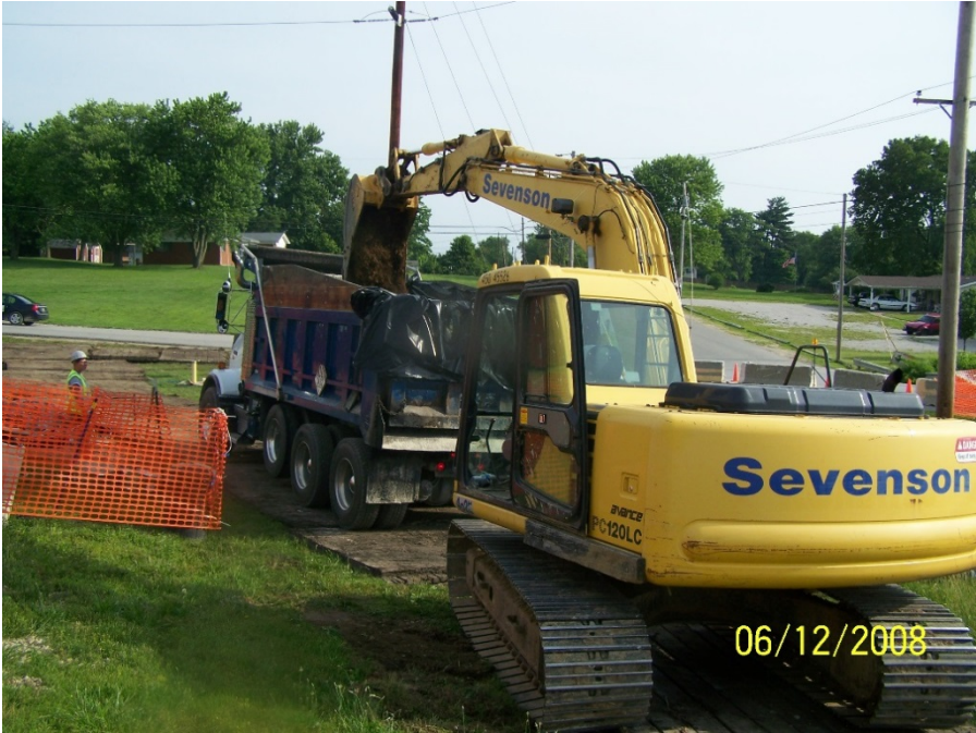
Photo No. 27: AOI 21-1 – Material loading for transport, facing north. June 2008.
