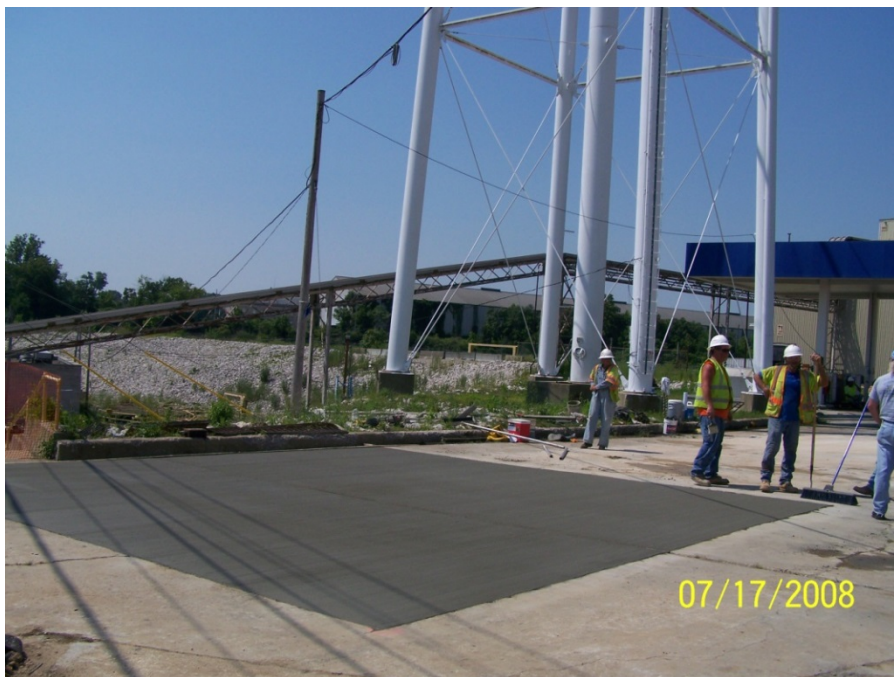
Photo No. 23: AOI 18 – Restored concrete slab, facing southwest. July 2008.
