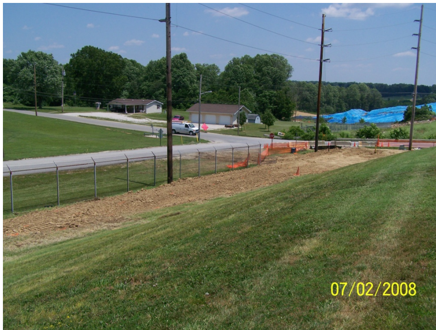
Photo No. 10: MH-ST-43 - Embankment grading, facing northeast. July 2008.
