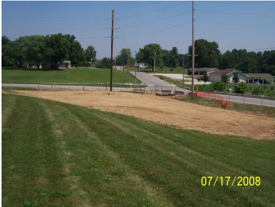
Photo No. 11: MH-ST-43 – Embankment grading, facing north. July 2008.
