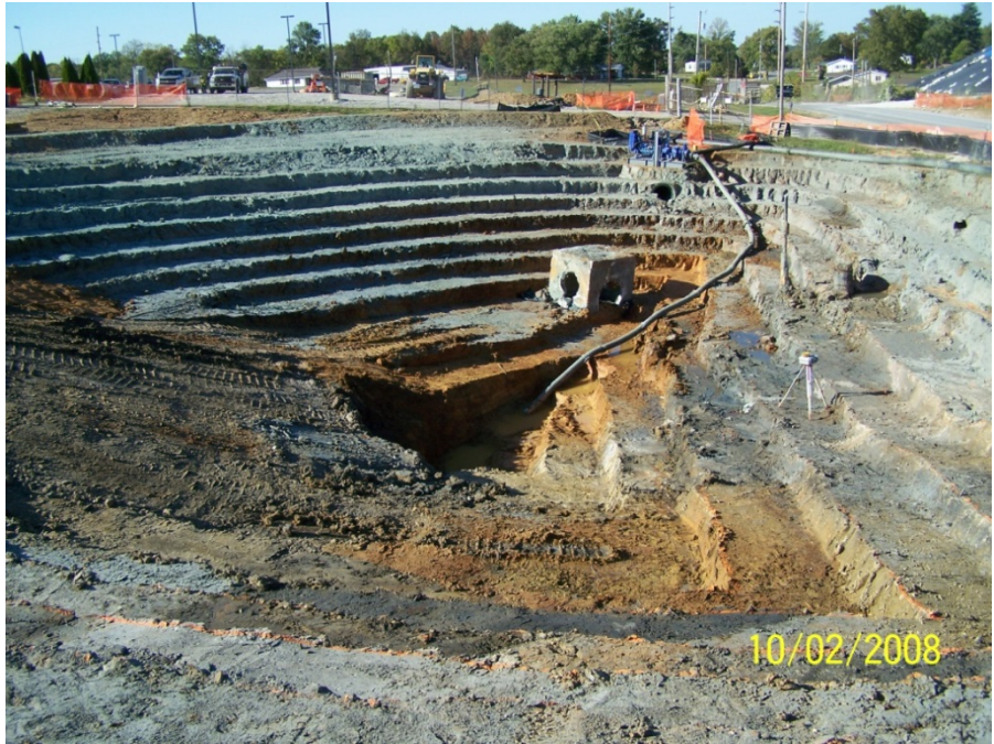
Photo No. 39: AOI 21-2 Excavation completion, facing north. October 2008.
