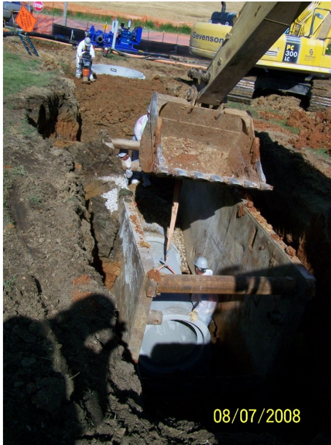
Photo No. 33: AOI 21-2 – Installation of storm sewer, facing east. August 2008.
