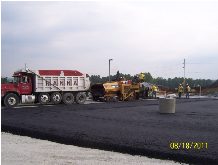
Photo No. 60: AOI 21-2 – Installation of asphalt binder layer, facing northeast. August 2011.
