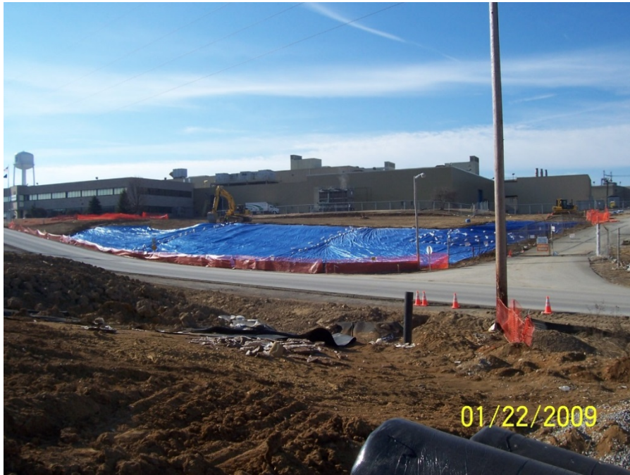
Photo No. 46: AOI 21-2 – Erosion protection for temporary soil cover on slope, facing southwest. January 2009.
