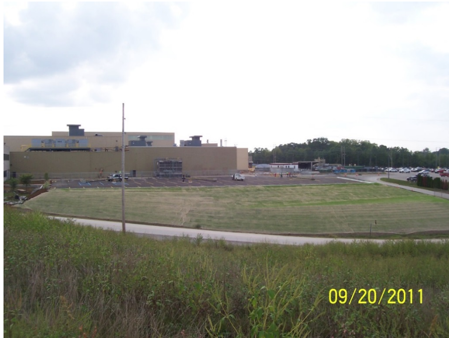
Photo No. 64: AOI 21-2 – Completed cover system, facing west. September 2011.
