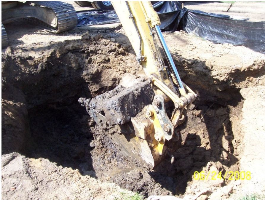
Photo No. 8: MH-ST-43 – Excavation of MH-ST-43, facing southwest. June 2008.
