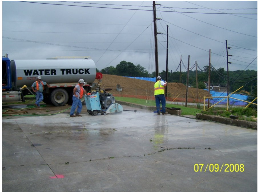
Photo No. 14: AOI 18 – Saw cutting, facing southeast. July 2008.
