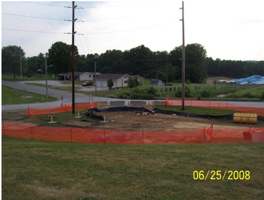
Photo No. 9: MH-ST-43 – Backfilling of MH-ST-43, facing northeast. June 2008.
