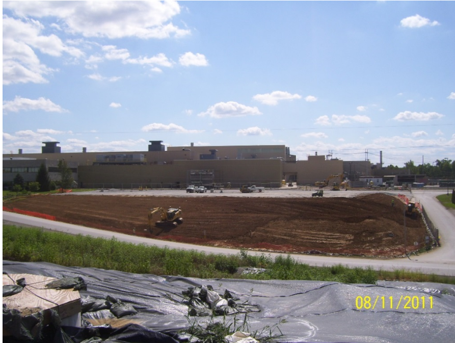
Photo No. 58: AOI 21-2 – Placement of topsoil, facing west. August 2011.
