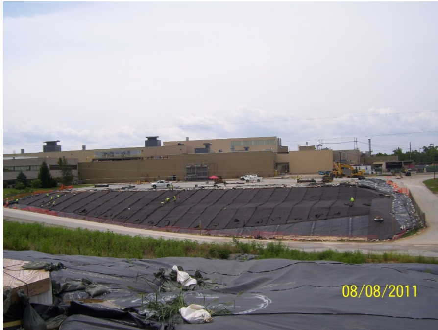
Photo No. 56: AOI 21-2 – Geonet drainage layer installation, facing west. August 2011.
