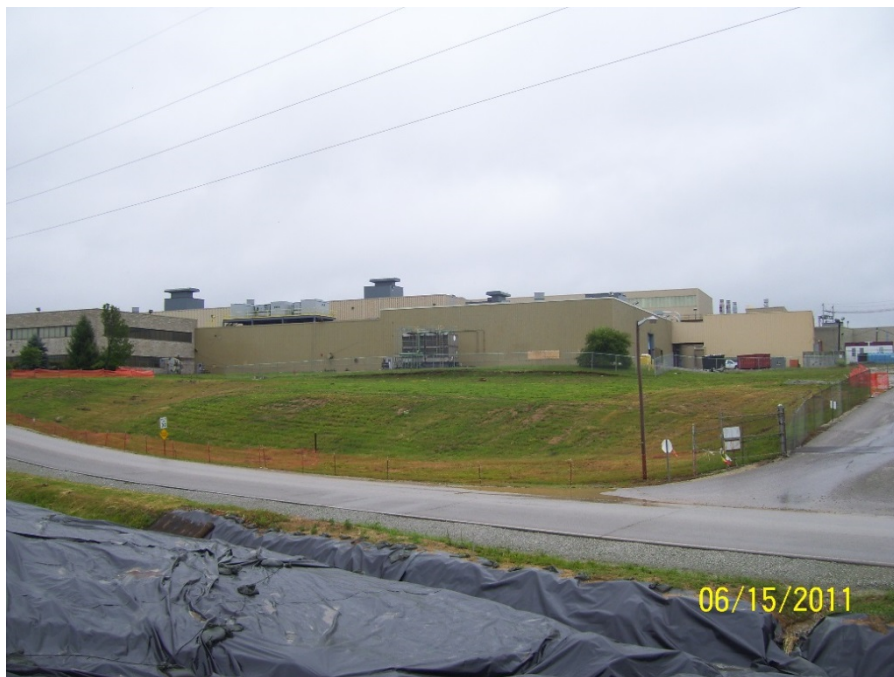
Photo No. 47: AOI 21-2 – Preparation for cover system construction, facing southwest. June 2011.
