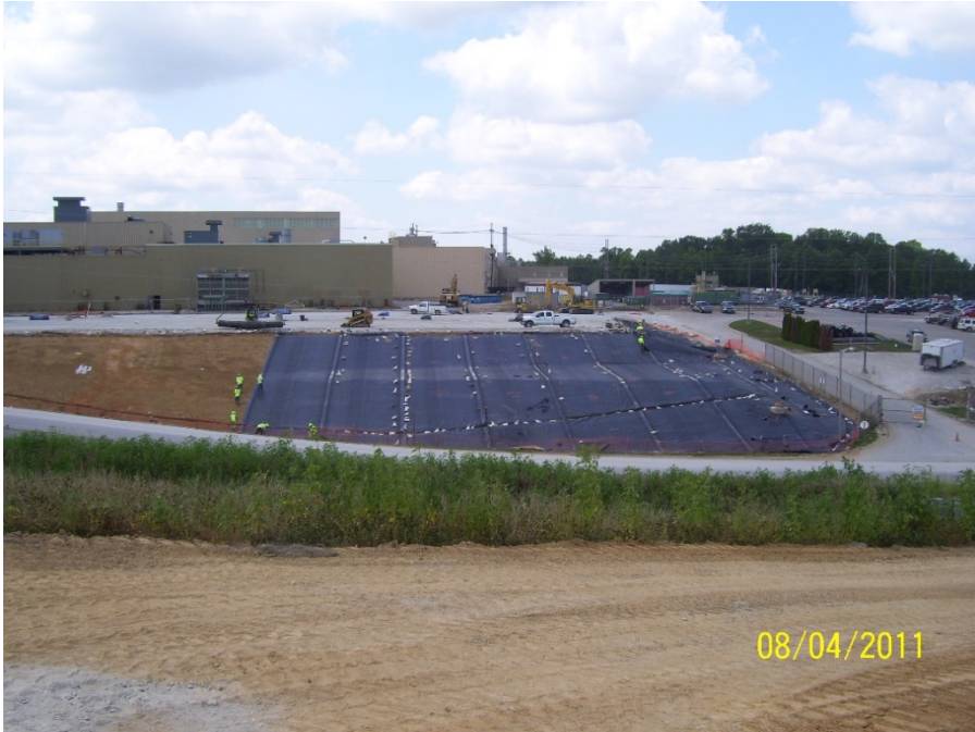
Photo No. 54: AOI 21-2 – Installation of LLDPE liner, facing west. August 2011.
