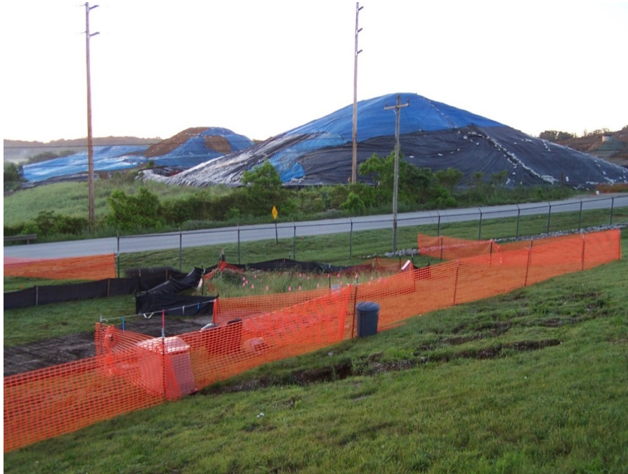
Photo No. 25: AOI 21-1 – Construction preparation, facing southeast. May 2008.
