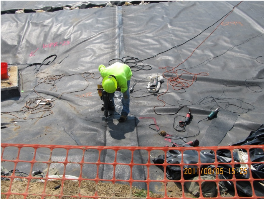
Photo No. 55: AOI 21-2 – Extrusion welding, facing west. August 2011.
