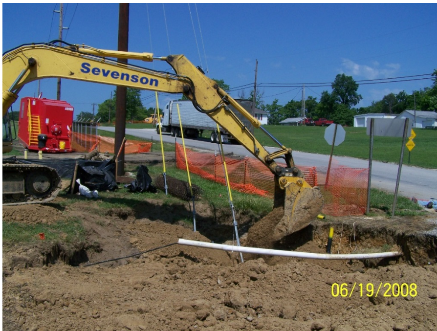
Photo No. 6: MH-ST-43 - Backfilling of sinkhole, facing northwest. June 2008.
