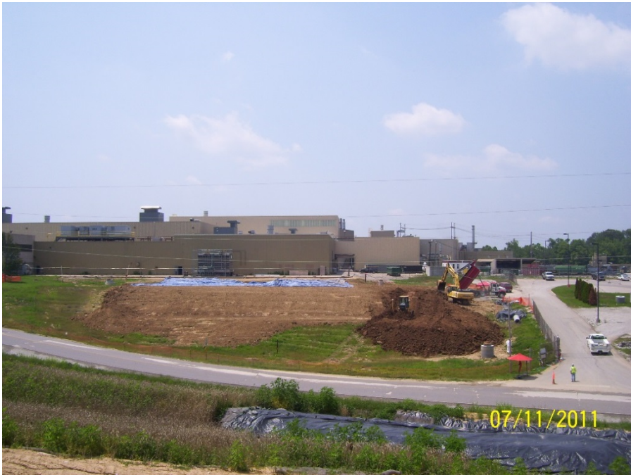
Photo No. 50: AOI 21-2 – Placement of grading fill with <50 mg/kg PCBs soil from CERCLA Removal Action, facing west. July 2011.
