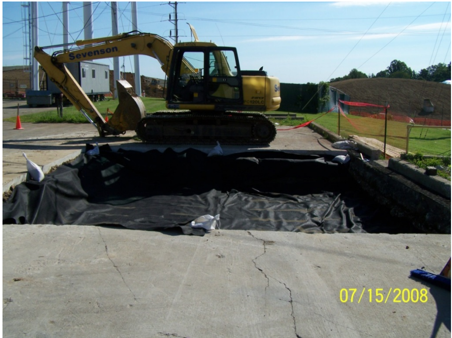
Photo No. 18: AOI 18 - Installation of geotextile, facing east. July 2008.
