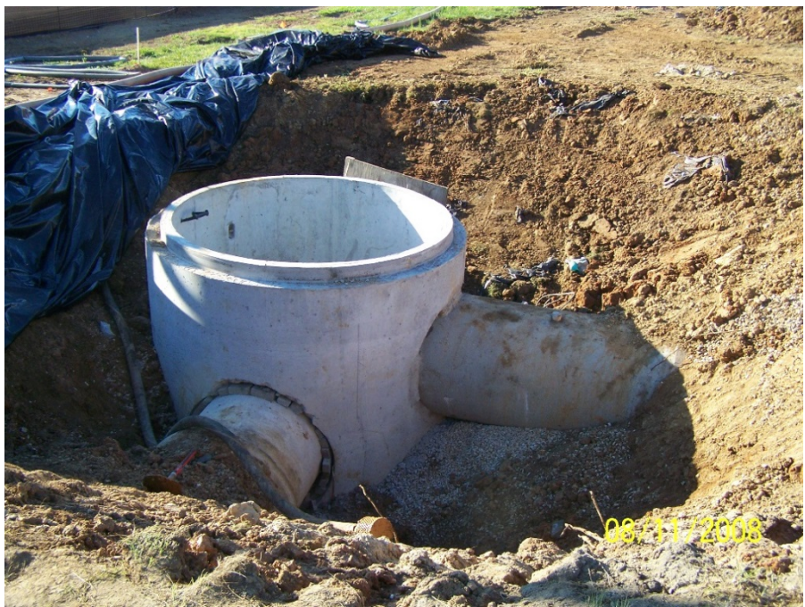
Photo No. 35: AOI 21-2 – Installation of manhole, facing southeast. August 2008.
