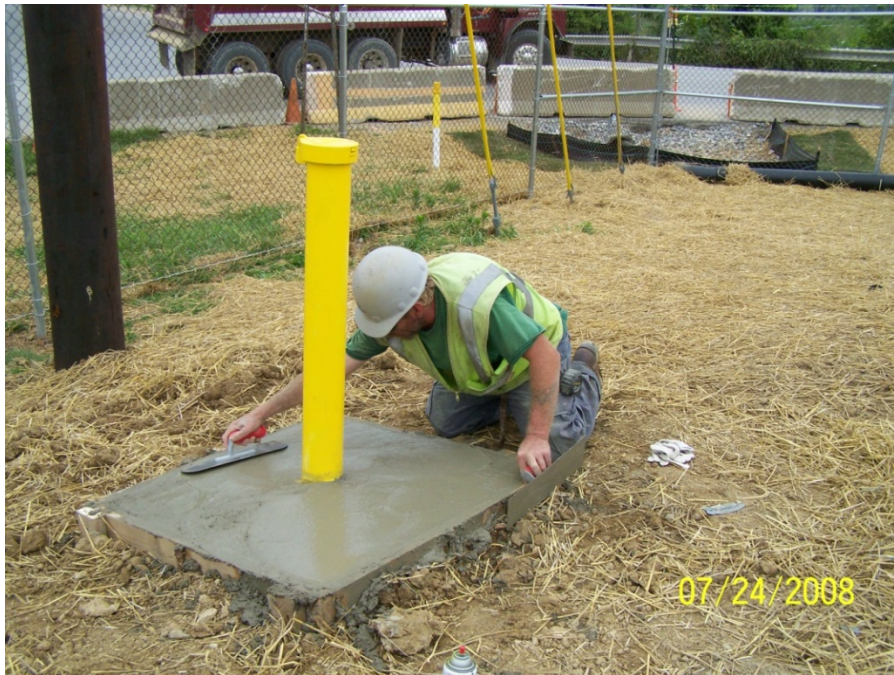
Photo No. 12: MH-ST-43 - Forming concrete around monitoring well, facing northeast. July 2008.
