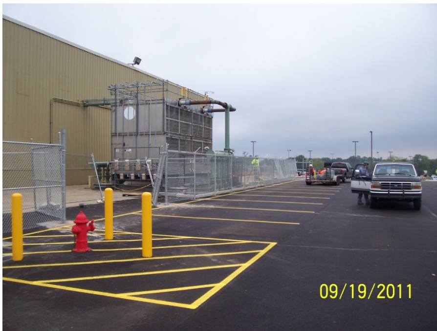
Photo No. 63: Installation of security fence, facing north. September 2011.
