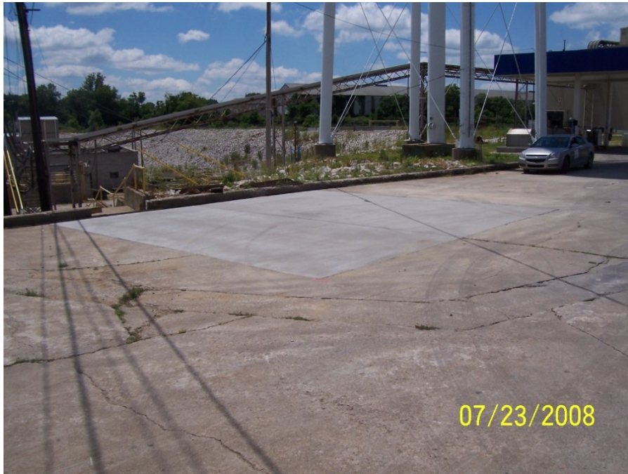
Photo No. 24: AOI 18 – Cured concrete slab, facing southwest. July 2008.
