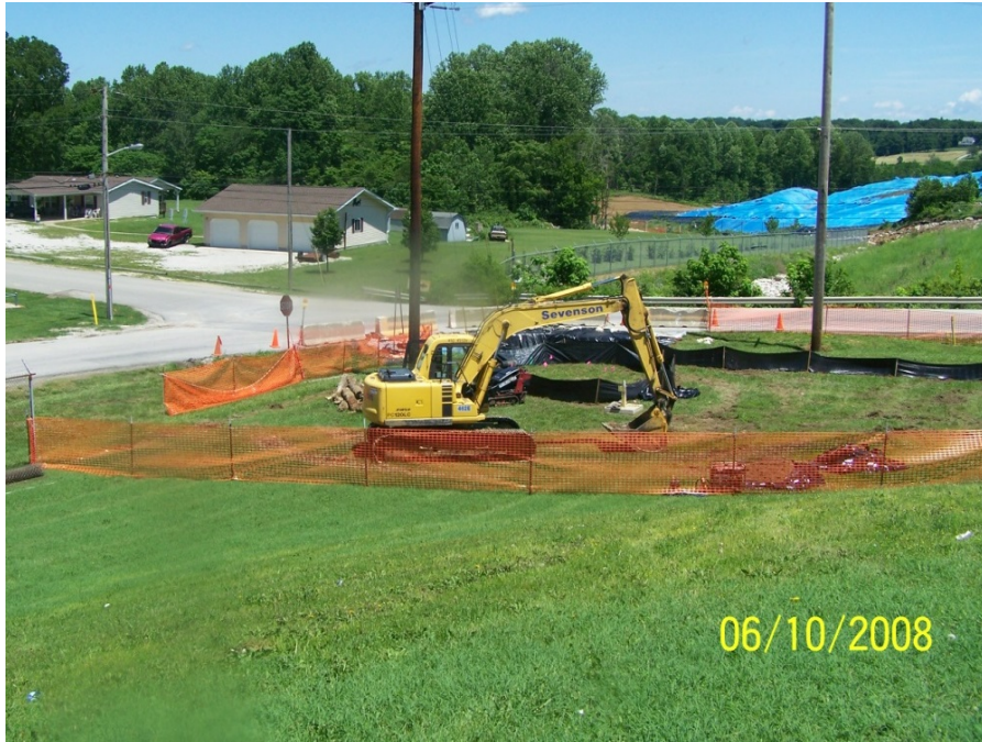
Photo No. 3: MH-ST-43 - Installation of temporary controls, facing northeast. June 2008.
