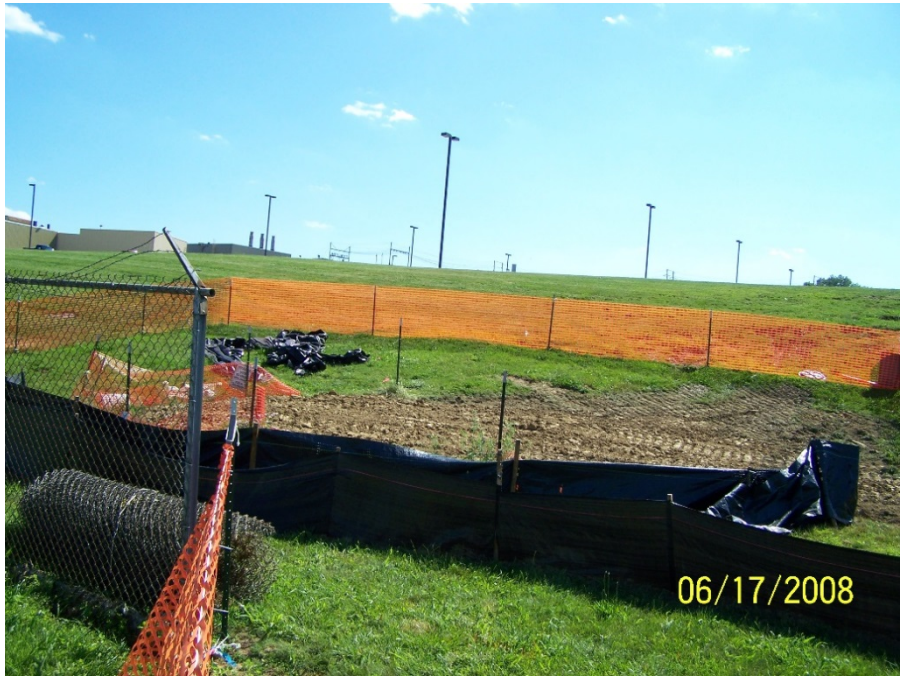
Photo No. 29: AOI 21-1 – Backfilling, facing southwest. June 2008.
