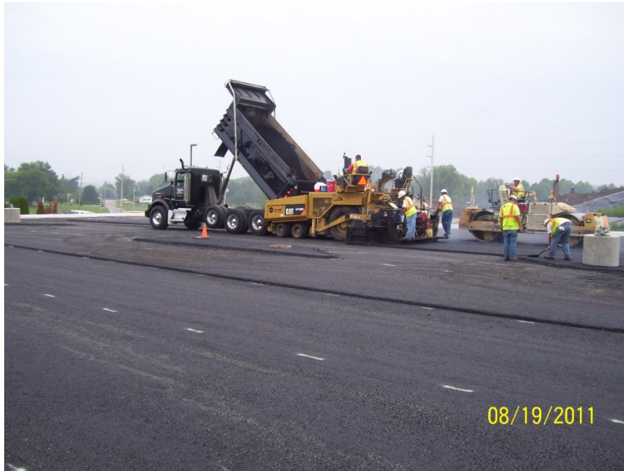
Photo No. 62: Installation of asphalt surface coat, facing northwest. August 2011.
