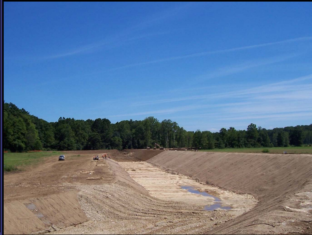
Diversion Channel No. 3 Excavation
