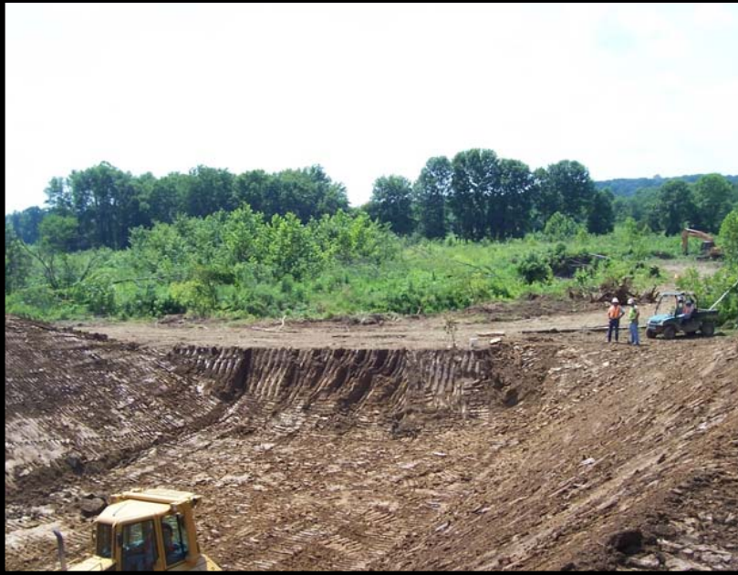
Diversion Channel No. 3 Excavation
