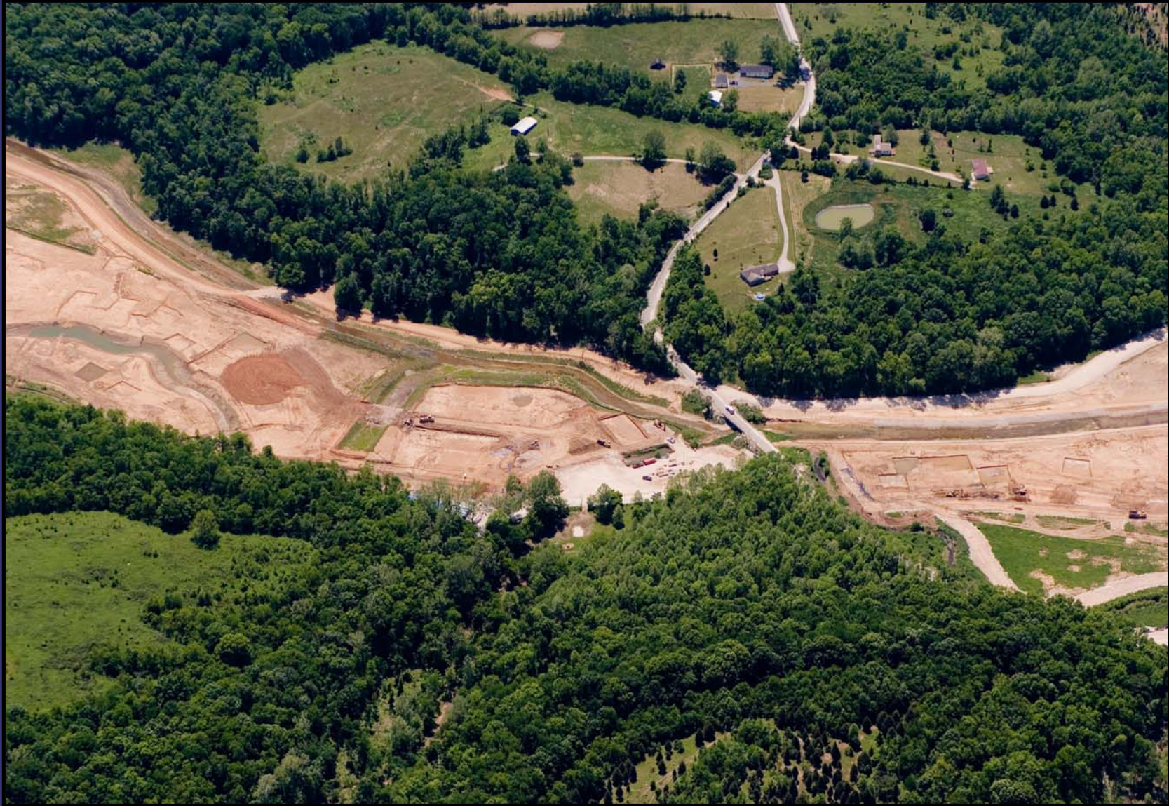
Excavation east of Peerless Road
