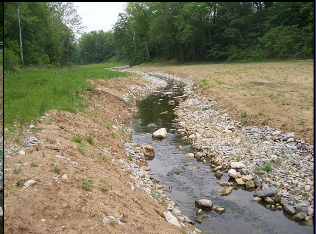
Property south of Broomsage Road
