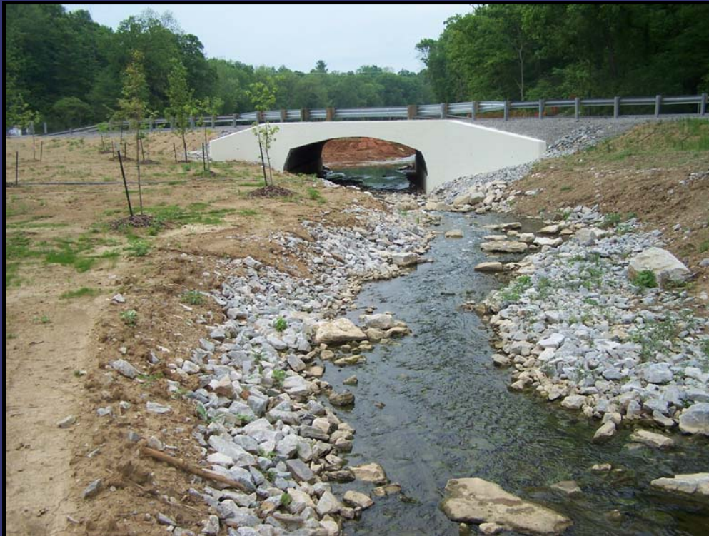
Property south of Broomsage Road restoration
