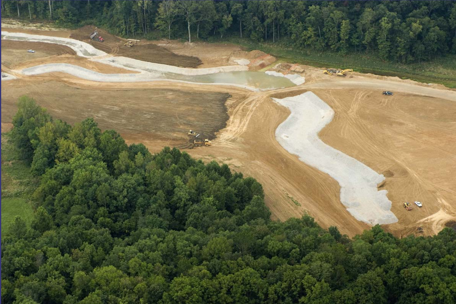
Restoration east of Peerless Road
