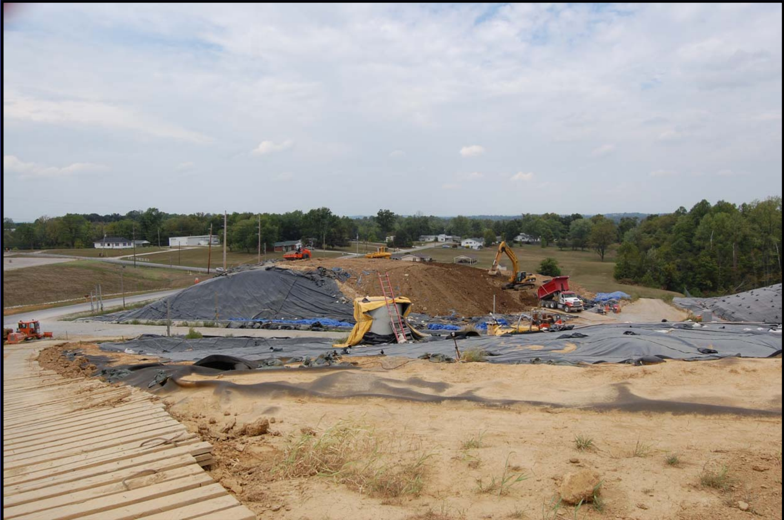
Stockpiling creek material in the East Plant Area off GM Drive.
