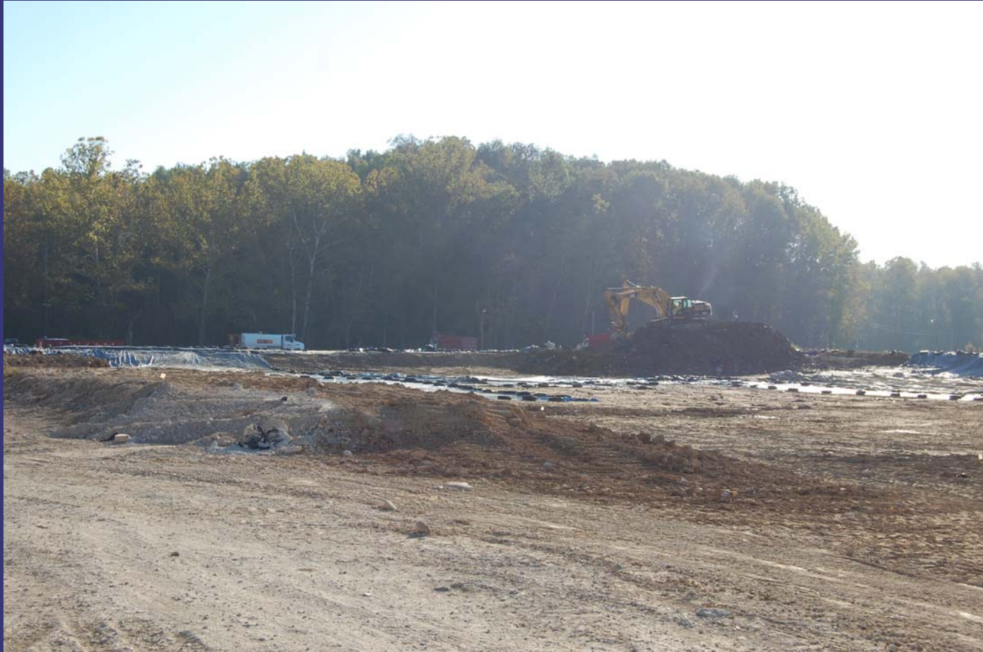
Soil pile remaining west of Peerless Road (September 2010)
