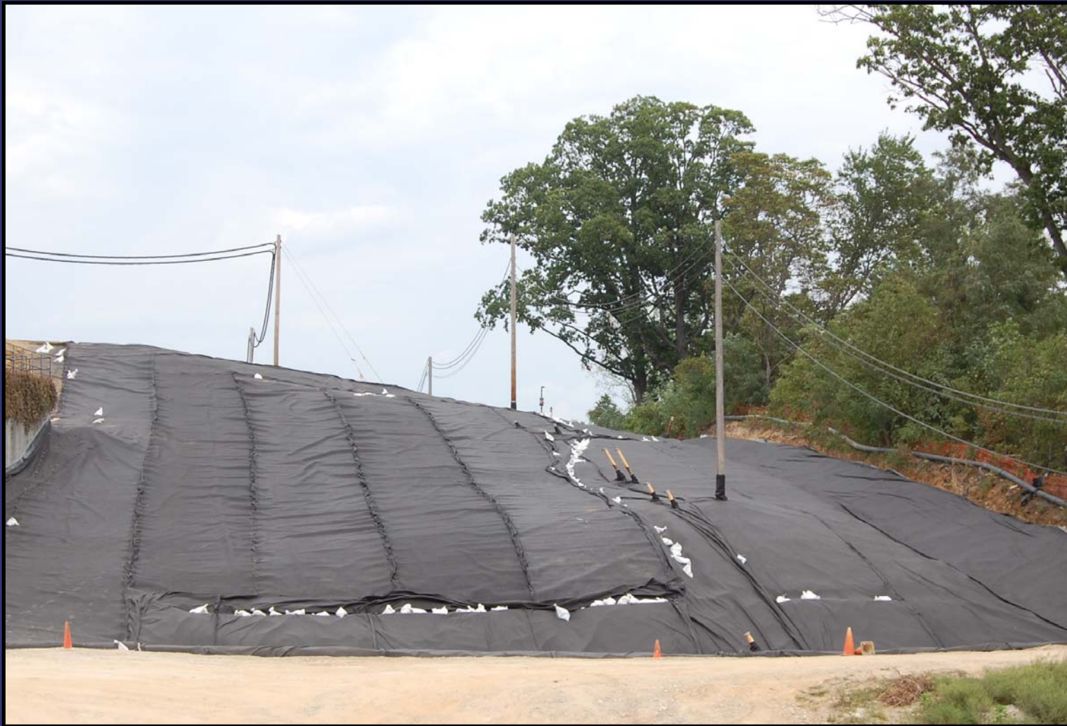
Liner installed east of water treatment facility prior to clay grading.
