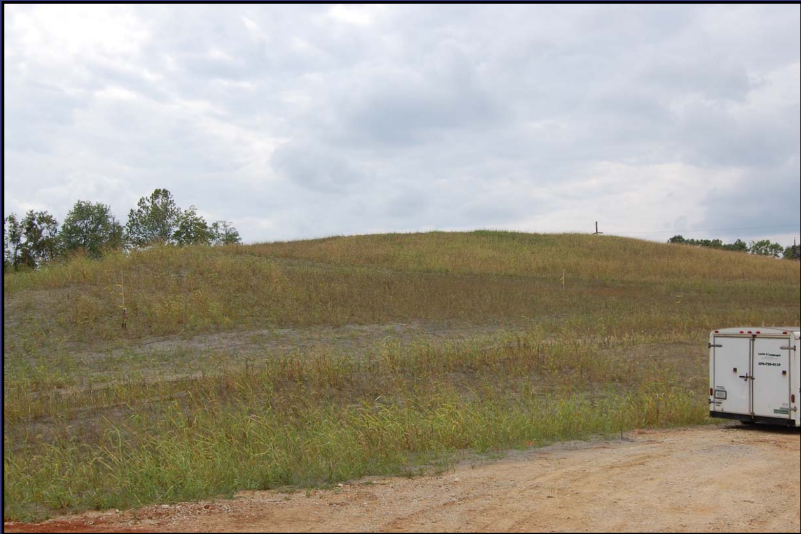
Parcel 201 off of GM Drive with completed cover.
