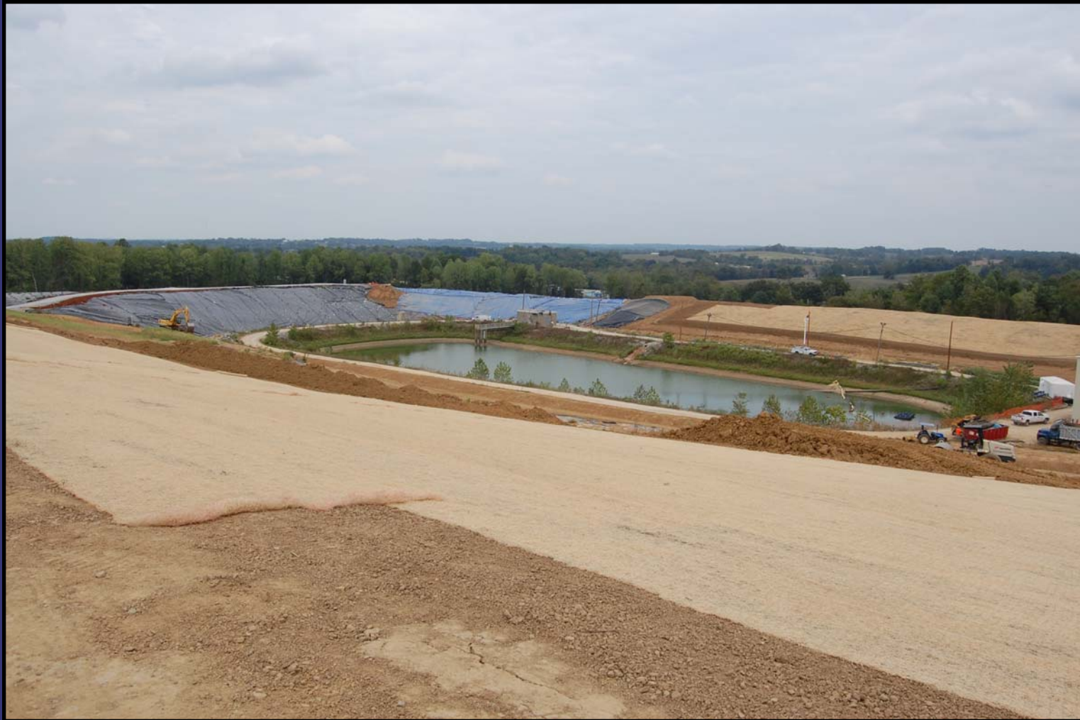
Partially completed covers and temporary liners visible around the stormwater pond.
