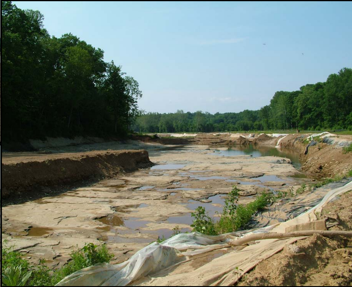
Parcels 25 and 28 – Excavation
