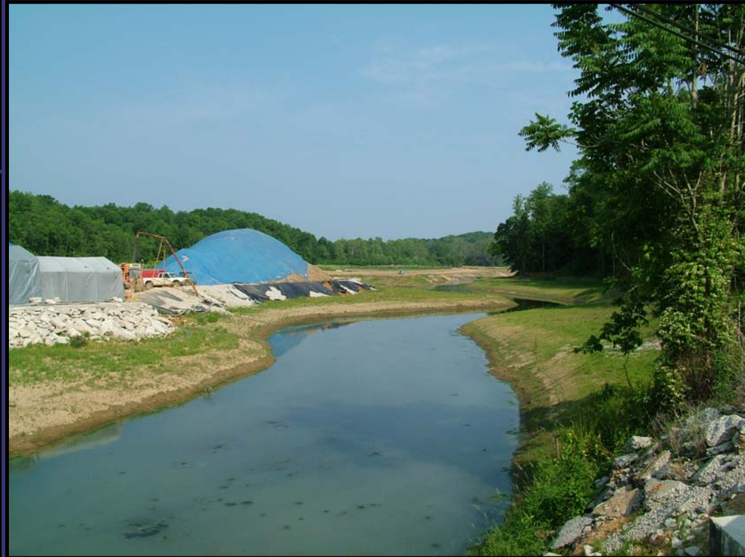
Diversion Channel No. 2 Excavation
