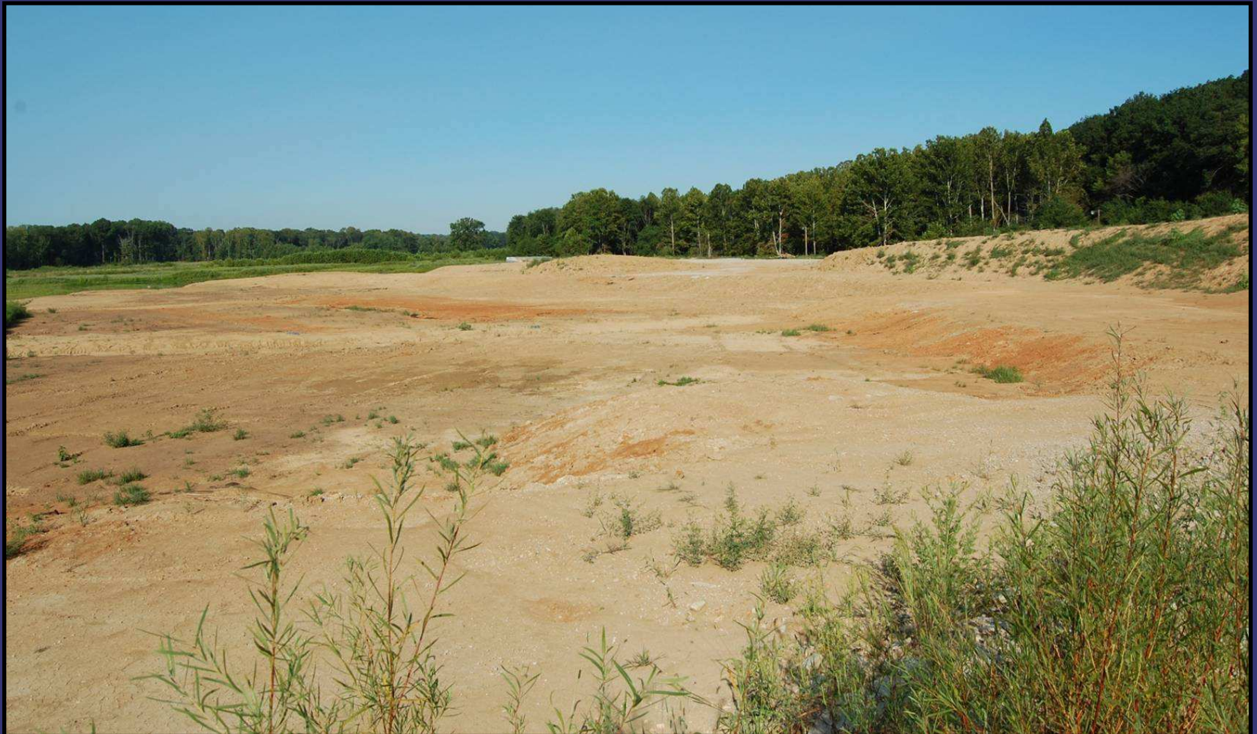
Completed excavation area west of Peerless Road
