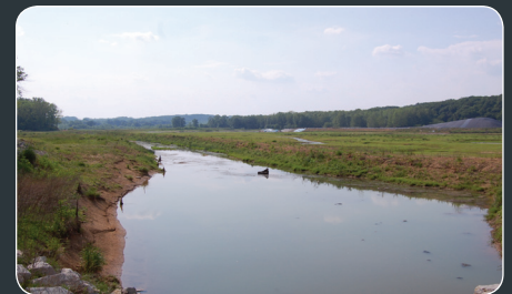
RESTORATION AND SOIL PILE REMAINING WEST OF PEERLESS ROAD.
