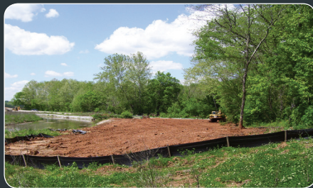
STATUS OF RESTORATION OFF OF BUD IKERD ROAD.
