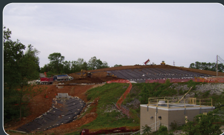
COVER SYSTEM WORK AT PARCEL 201.
