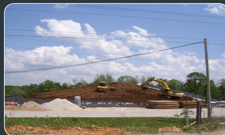
PARCEL 201 SOIL GRADING ACTIVITIES.
