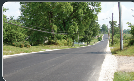
COMPLETED PAVING ALONG A STRETCH OF PEERLESS ROAD.
